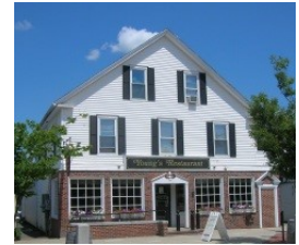
Young's Restaurant – a 2-1/2 story building (150)
