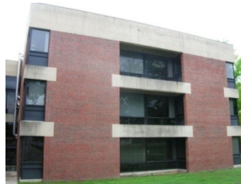
The mammoth concrete headers over the openings convey an outsized (non-human) scale to this Williams College (Massachusetts) building. (51)
