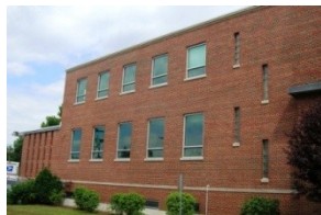
Creative variation in the window pattern, can add interest as in the Durham Post Office. (84)
