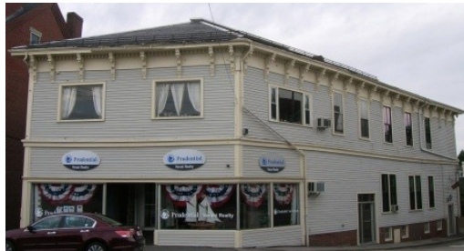
Square windows, especially when unbroken by muntins, are inherently unsatisfying. This is evident in comparing the original and inappropriate picture windows on this Exeter building. (91&92)
