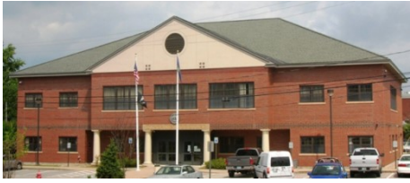
The new courthouse in downtown Dover suffers a fatal flaw in emphasizing horizontality over verticality. (111)
