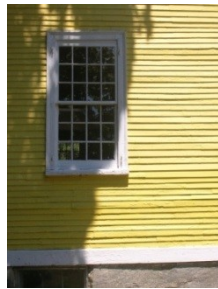
The narrow clapboards brings an intimate scale to the main structure of the Three Chimney's Inn (46)
