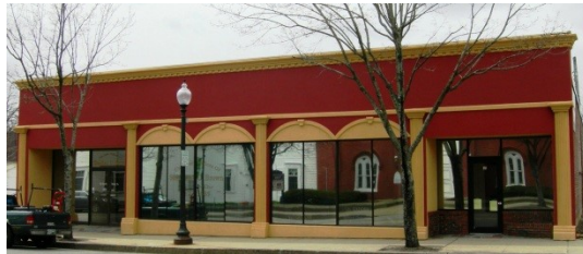
Rochester – new façade (59)
