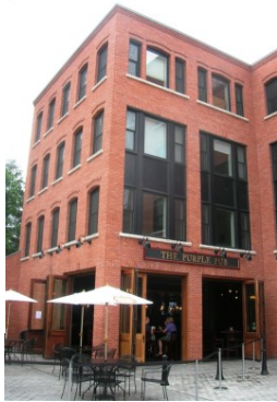
A high-quality red brick is used on this new Williamstown, MA building. (116)
