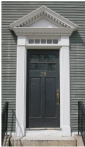
Door surround Ballard House (100)
