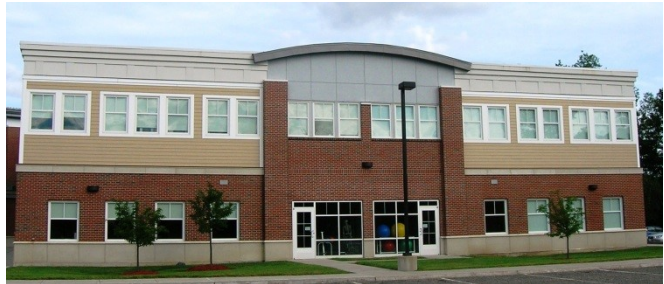
It is now vogue to mix clapboard and shingles, usually in vinyl (top), and other materials (above). Use of more than one primary material on the façade often presents a lack of clarity or focus in design. (120&121)
