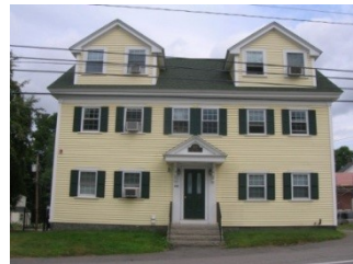
The dormers are out of proportion relative to the rest of the house resulting in an ungainly, top-heavy appearance. (58)
