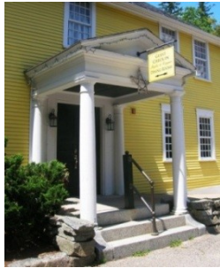
Portico/Entry Porch Three Chimney's Inn (101)
