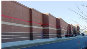
A series of stepped back facades is often used in a misguided attempt to add interest to building. (photographer unknown) (114)
