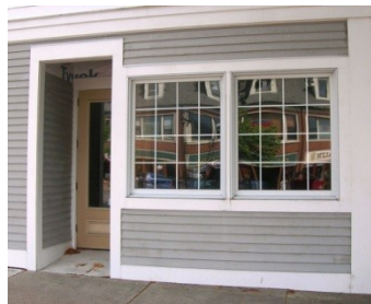
The windows are squat/square and the fake grille impedes visibility. Clapboards are generally too rustic in character to use on a storefront. (137)
