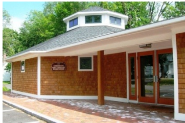
Cellular PVC is used for trim on the Unitarian Church function hall. (119)
