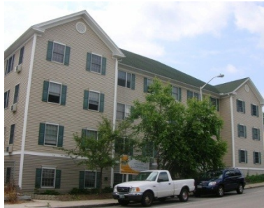
There is an overriding plastic feel about this building clad in vinyl. (122)
