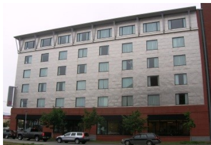
Insubstantial or eccentric materials, like this thin metal siding, shall not be used. (124)
