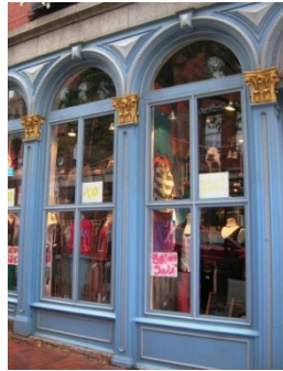
If a grille is to be used it shall be composed of real through-muntins and separate panes of glass. (133)
