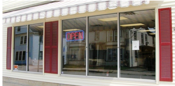
The base/bulkhead is too low and the expanse of large glass panes is too extensive. (136)
