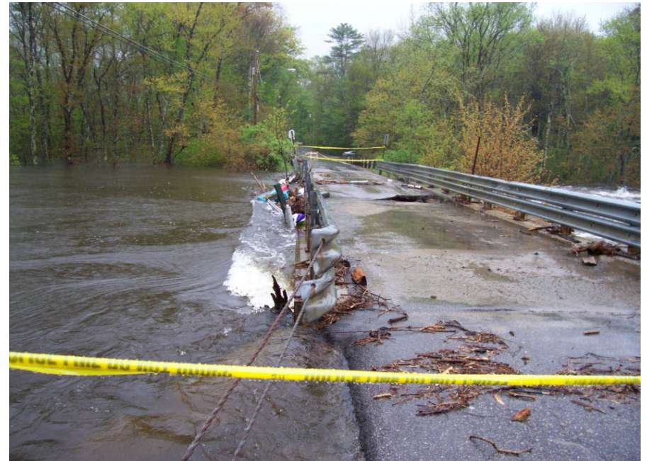
Wiswall Bridge during May 2006 Flood Event (Photo Credit: Durham Hazard Mitigation Plan)
