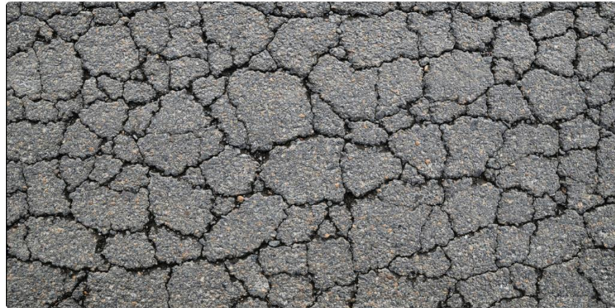
Fatigue cracking
