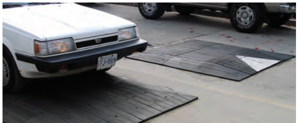
Temporary Speed Cushion
