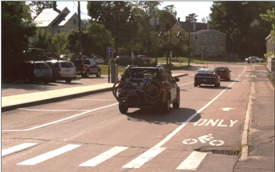
FIGURE 3: BICYCLE LANE, CROSSWALK, AND SIDEWALKS ON PETTEE BROOK LANE
