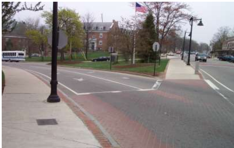
Figure 3: Mill Road Stop-Controlled Approach
