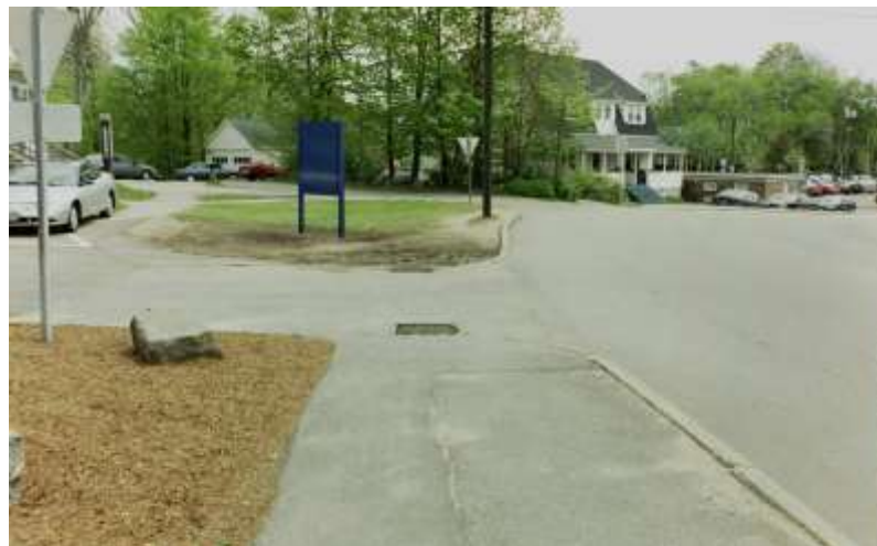
Figure 9: Discontinuous Sidewalk on Pettee Brook Lane
