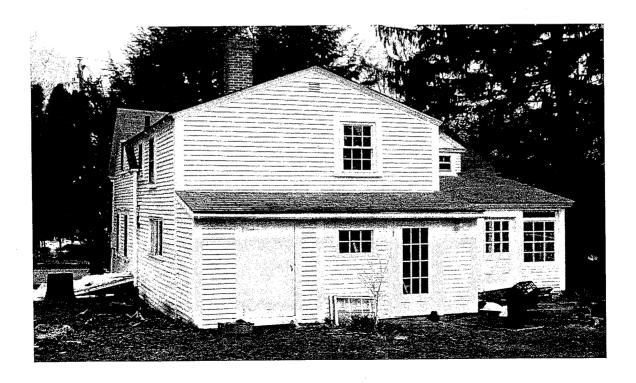
**Southerly side changes**. The photograph below shows the proposed changes of the southerly side of the "ell" which would include changing the existing sliding window to a six over six window/sash, changing the existing second floor bathroom window to a six over three window /sash and adding another six over three window /sash beneath the new upper six over three window /sash.
