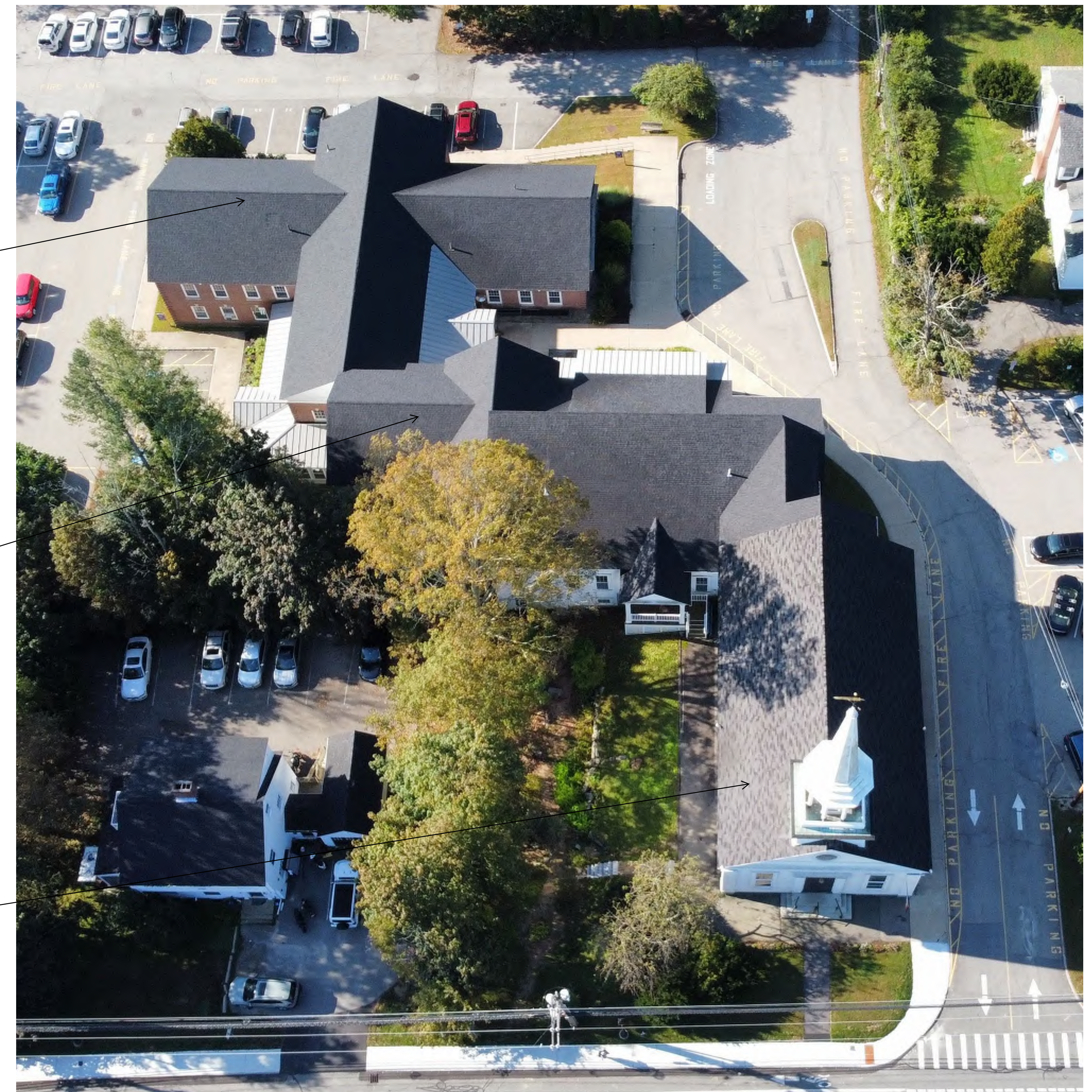
Overall Building & Site Layout (Overhead view from North/ Main St.) No Scale
