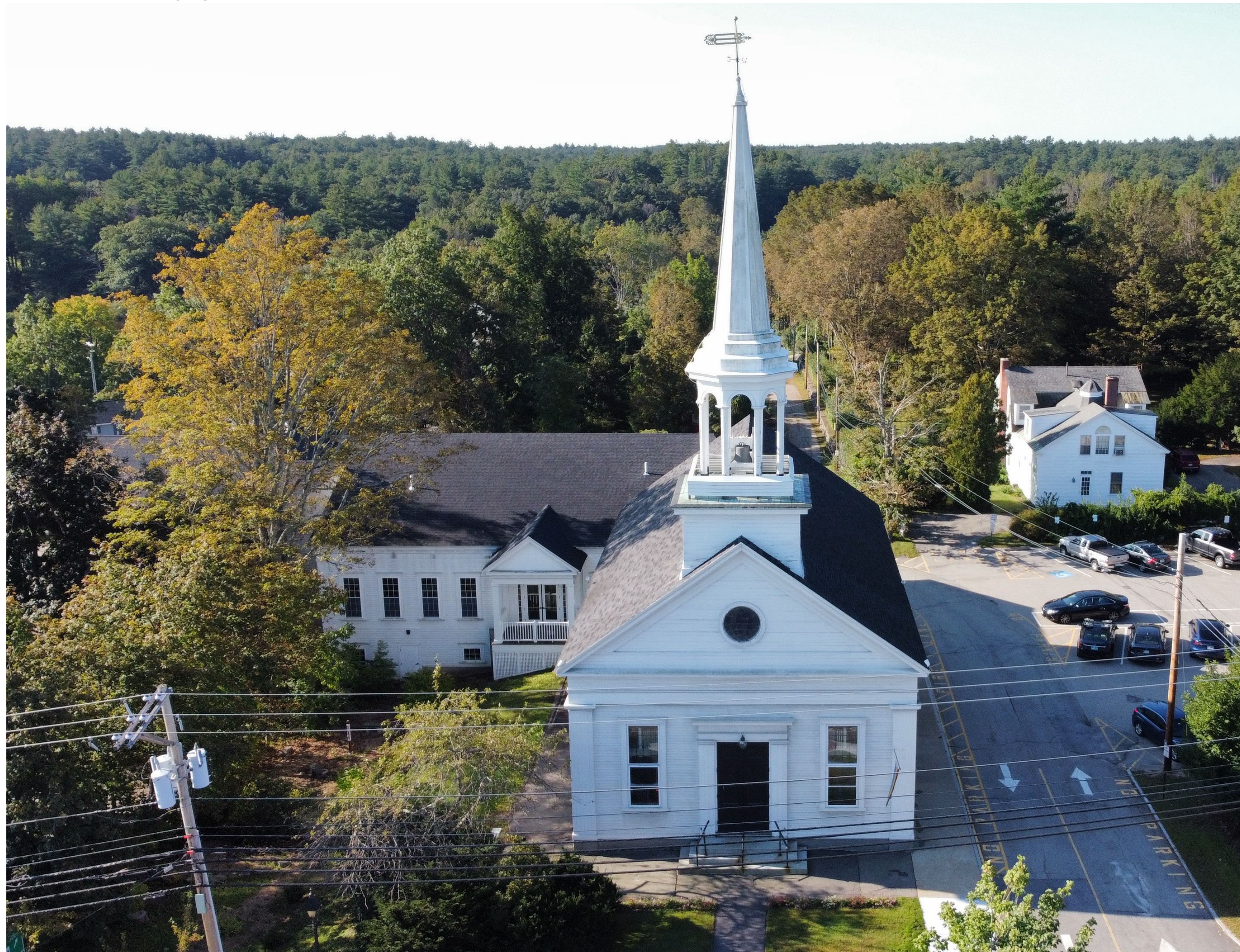
View of Existing Church from Main Street No Scale
