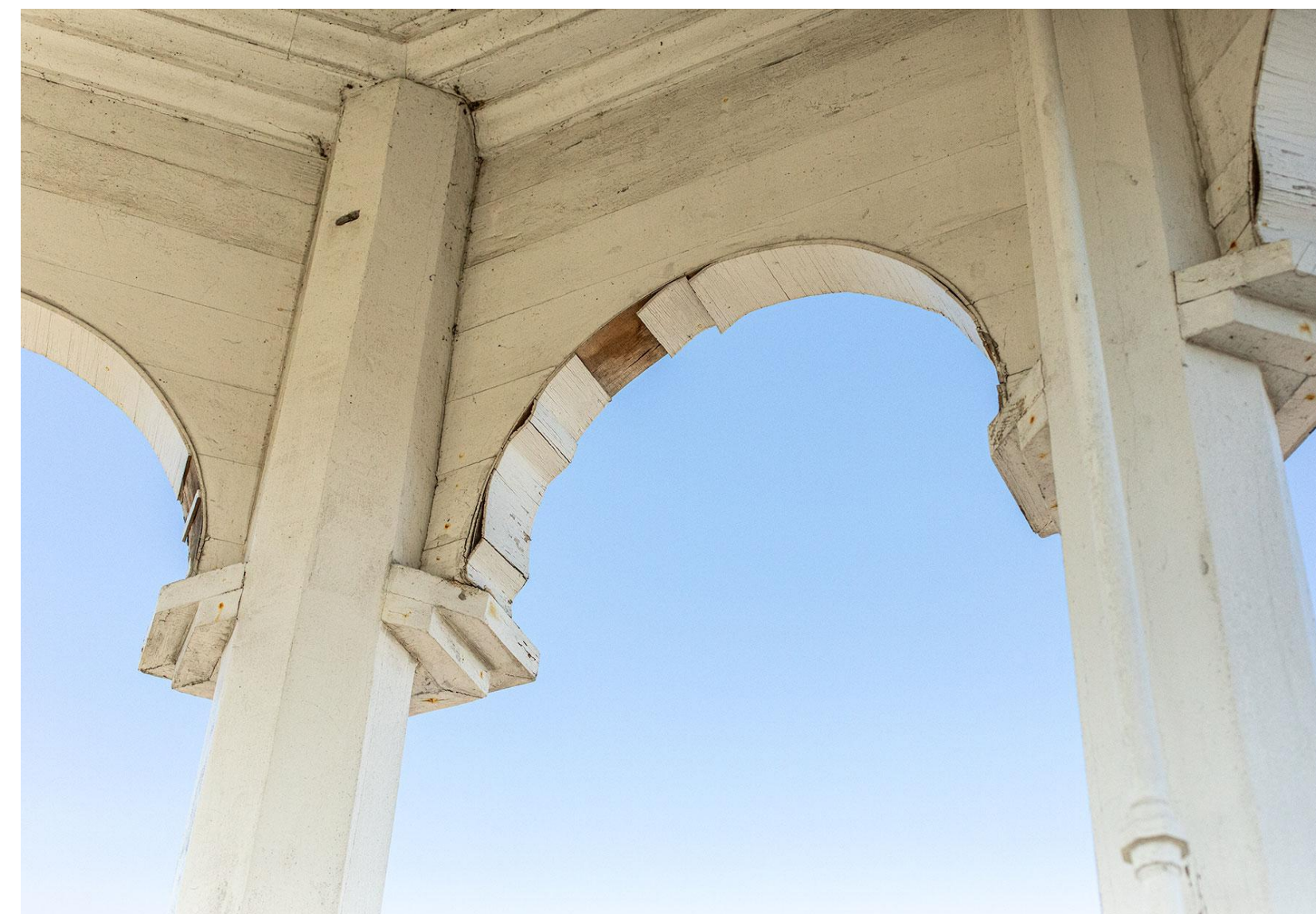
Image of Existing Arched Trim Condition
