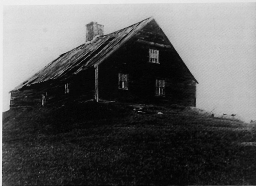
Bunker garrison house, Durham, built in 1652. The war-party's first priority was to ambush the fortified houses toward which neighborhood residents would attempt to flee. The Bunker garrison was one of the few to withstand the attack. Garrisons differed little from other houses of the time, except for their hewn log construction and their defensible location, often on a height of land. Photograph courtesy of the Durham Historical Association Museum.
