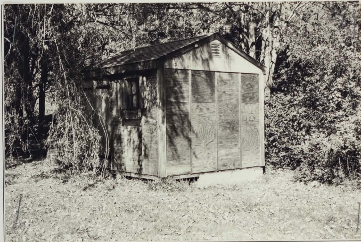
Photo 18 description: Shed Roll: 1 Frame: 12 Direction: NW
