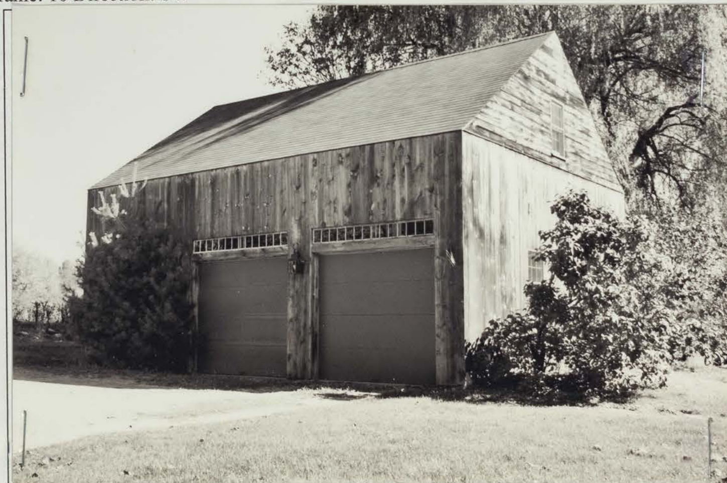
Photo 17 description: New barn/garage erected ca. 1992 Roll: 1 Frame: 13 Direction: NE Address: 97 Newmarket Road Date taken: October 2004-January 2005 Negative stored at: NHDHR
