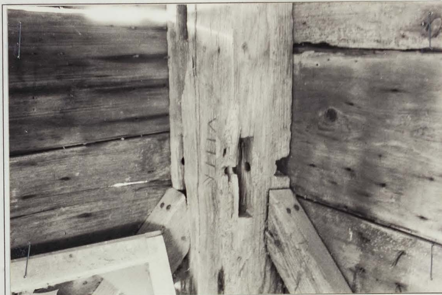
Photo 16 description: Detail of SW corner post, showing scribe mark at unused mortise Roll: 3 Frame: 10 Direction: SW
