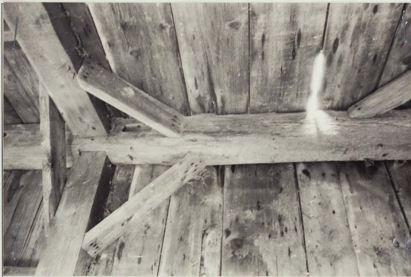
Photo 14 description: Detail, SE corner of barn Roll: 3 Frame: 8 Direction: SE
