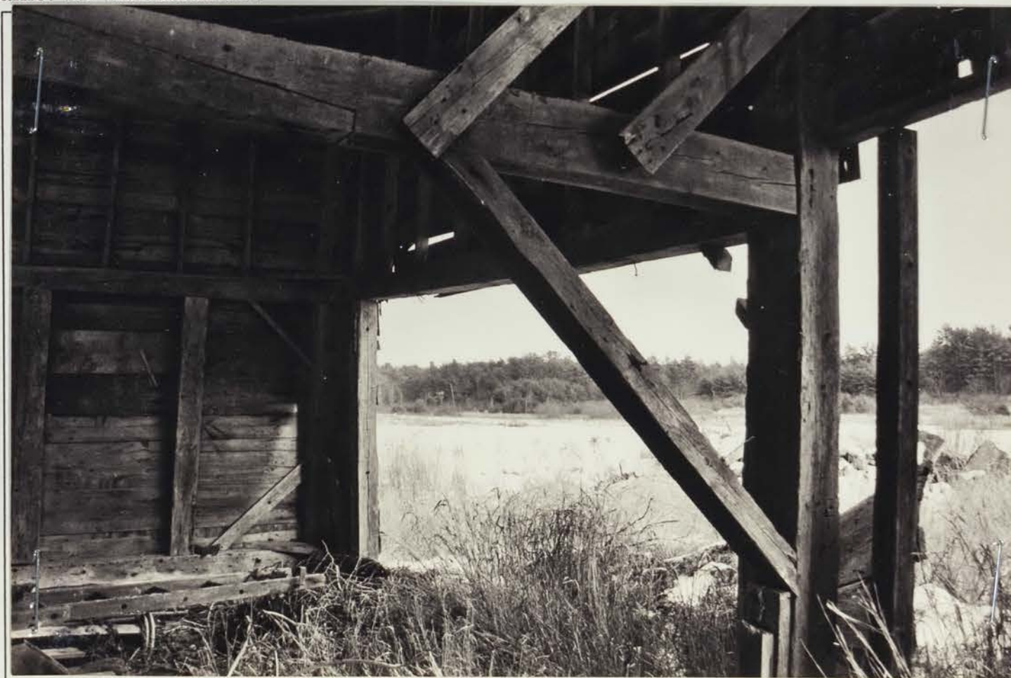
Photo 11 description: Interior framing of barn, showing the two wagon openings along east wall Roll: 3 Frame: 7 Direction: NE
