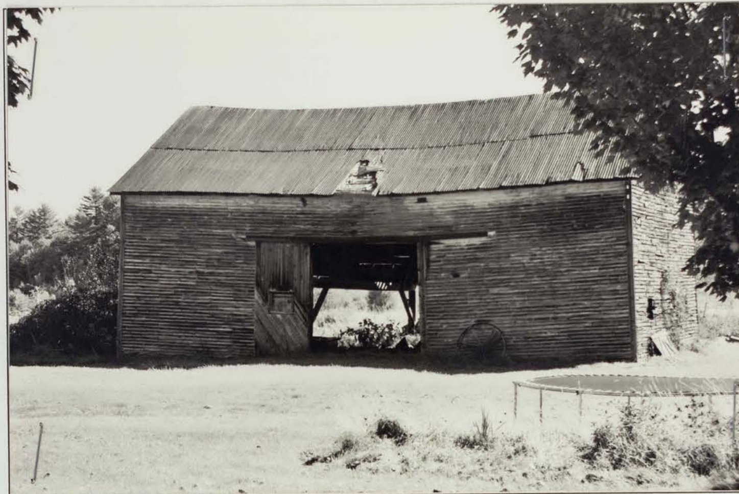
Photo 8 description: West elevation of barn Roll: 1 Frame: 8 Direction: E
