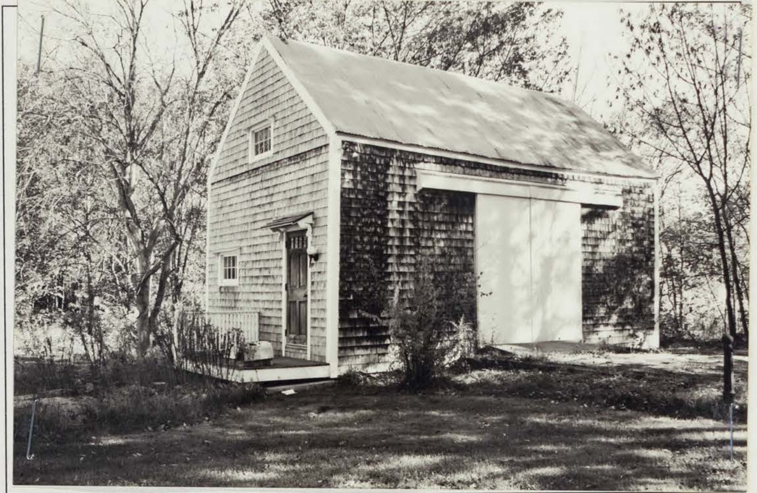
Photo 4 description: Barn/cottage: facade and north elevation Roll: 2 Frame: 15 Direction: SE
