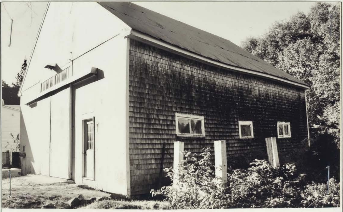
Photo 7 description: Barn: facade and east elevations Roll: 2 Frame: 20 Direction: NW
