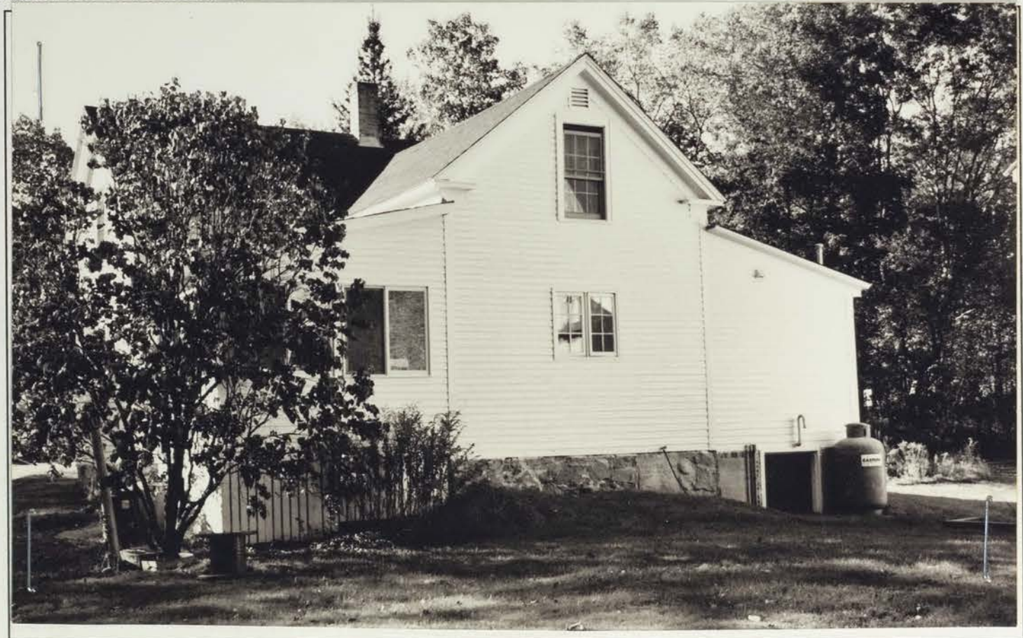
Photo 3 description: Rear elevation of ell, showing north addition at right Roll: 2 Frame: 19 Direction: NW
