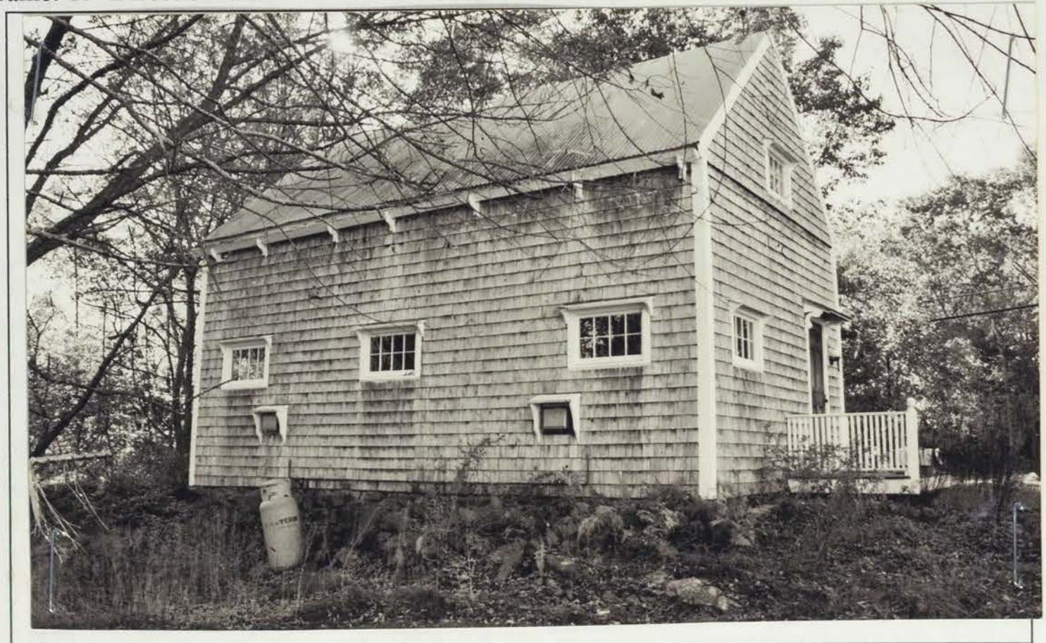
Photo 5 description: Barn/cottage: rear (east) and north elevations Roll: 2 Frame: 16 Direction: SW
