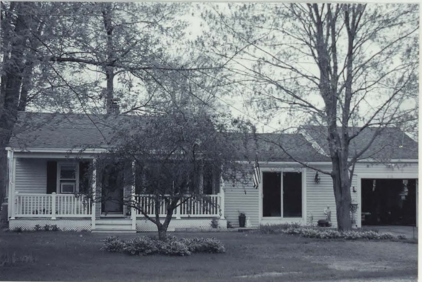
Photo #42 Description: 216 Newmarket Road (#19), façade (east elevation) Direction: W
