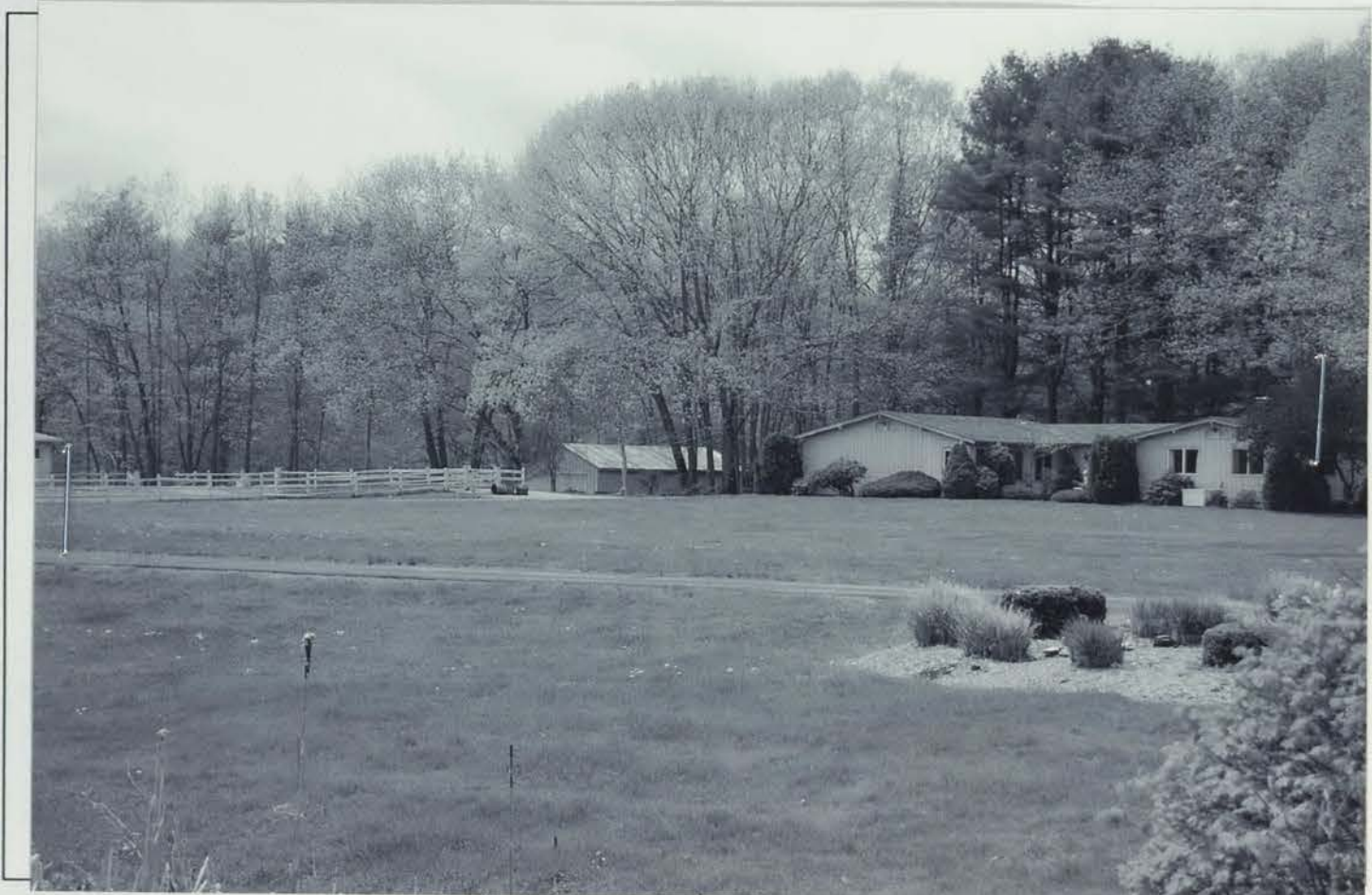
Photo #44 Description: 250 Newmarket Road (#21), façade (east elevation) Direction: W
