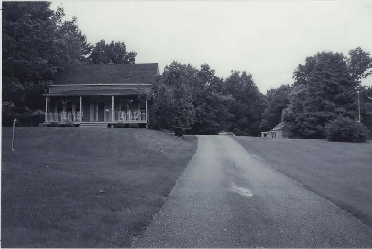
Photo #7 Description: Jos. Bunker-Emile Hamel House (#4), 110 Newmarket Rd. House at left & shed/shop at right
