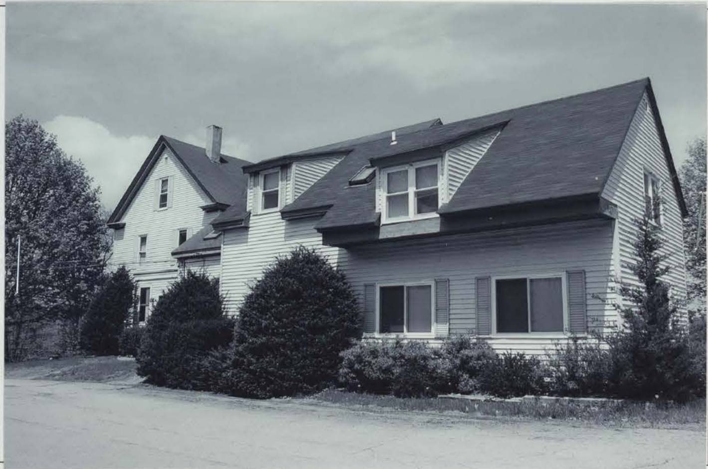
Photo #46 Description: Hale Stevens Farmhouse (#22), south elevation, showing ell & rear addition (or former attached barn) Direction: NW
