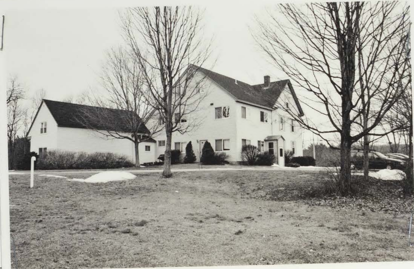
Photo #36 Description: Hale Stevens Farmhouse, rear and north elevations Roll: 4 Frame: 3 Direction: SW
