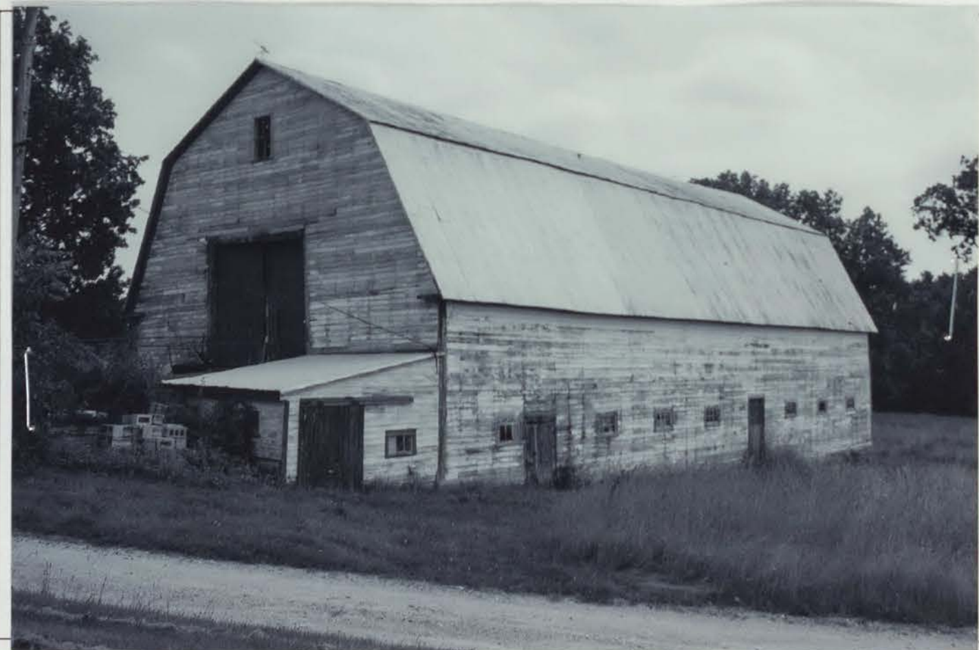
Photo #34 Description: Dame-Bedard Farm (#16): barn (north gable front & west elevation) and milk house Direction: SE
