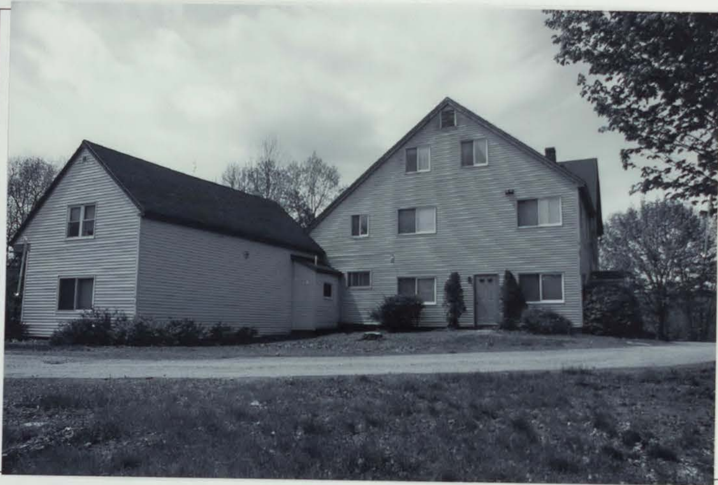
Photo #47 Description: Hale Stevens Farmhouse (#22), rear elevation & former attached barn (?) at left
