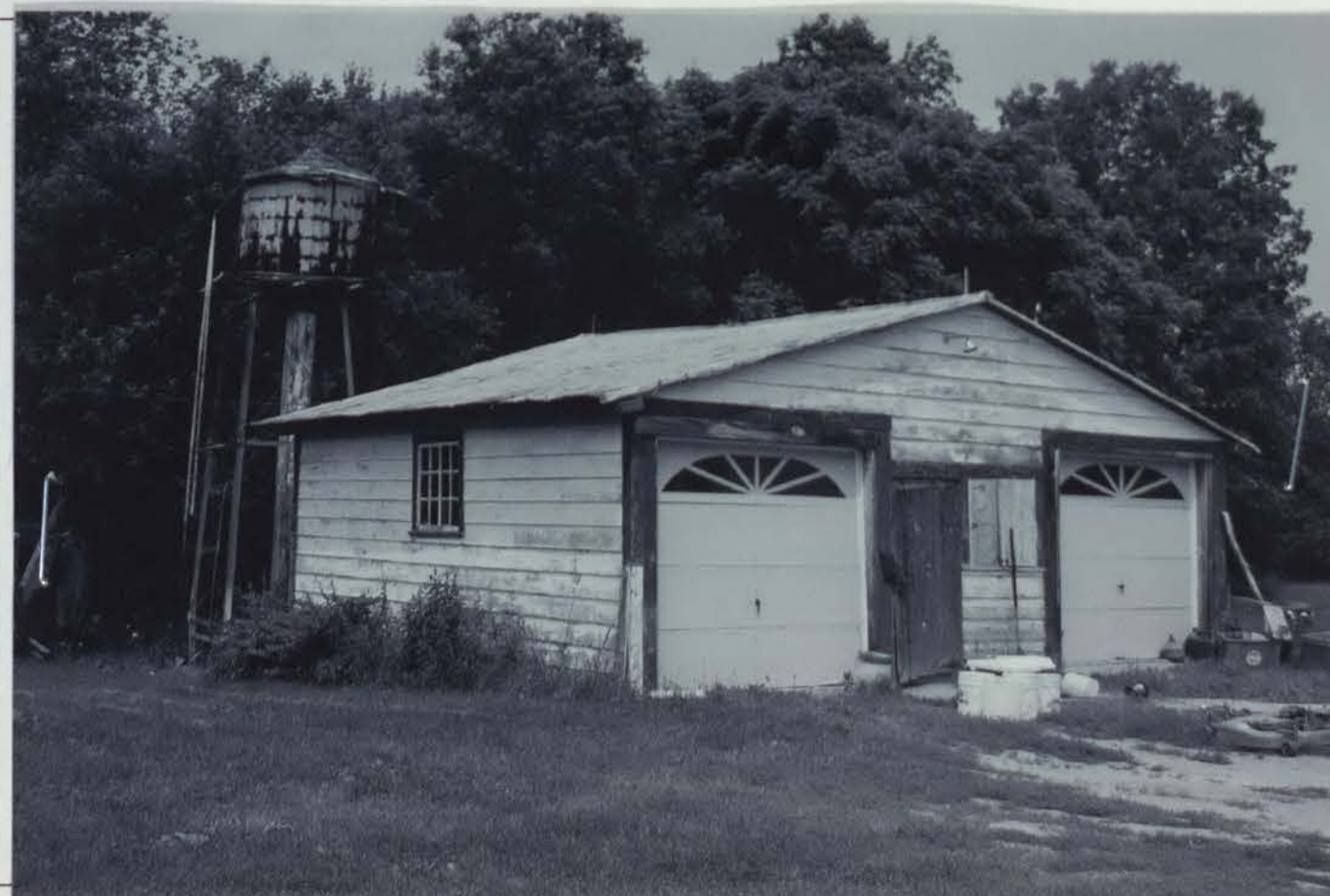
Photo #36 Description: Dame-Bedard Farm (#16): water storage tank and garage
