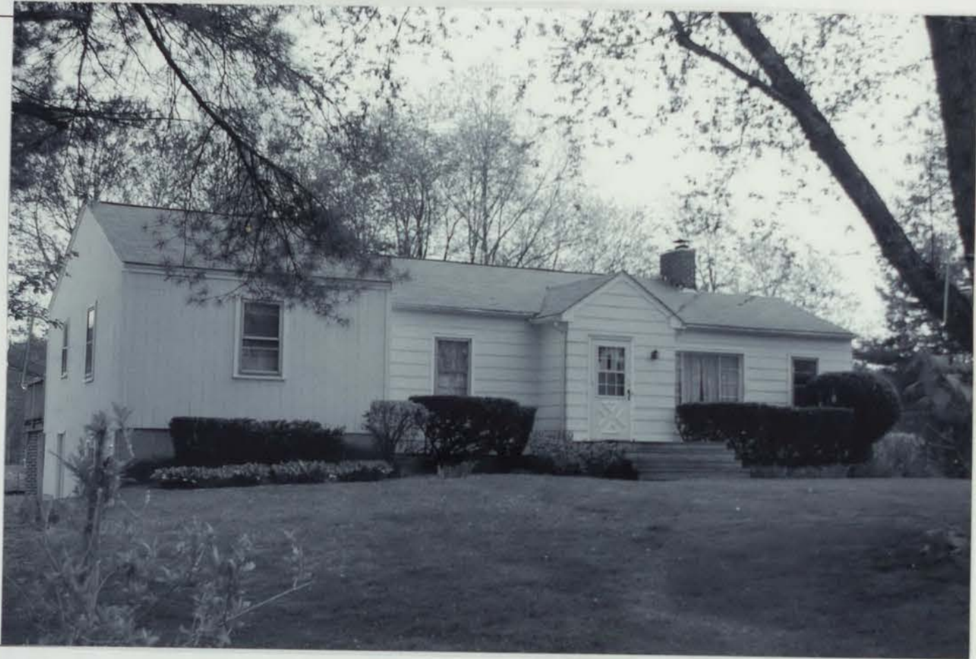
Photo #41 Description: 221 Newmarket Road (#18), façade (west elevation) Direction: SE
