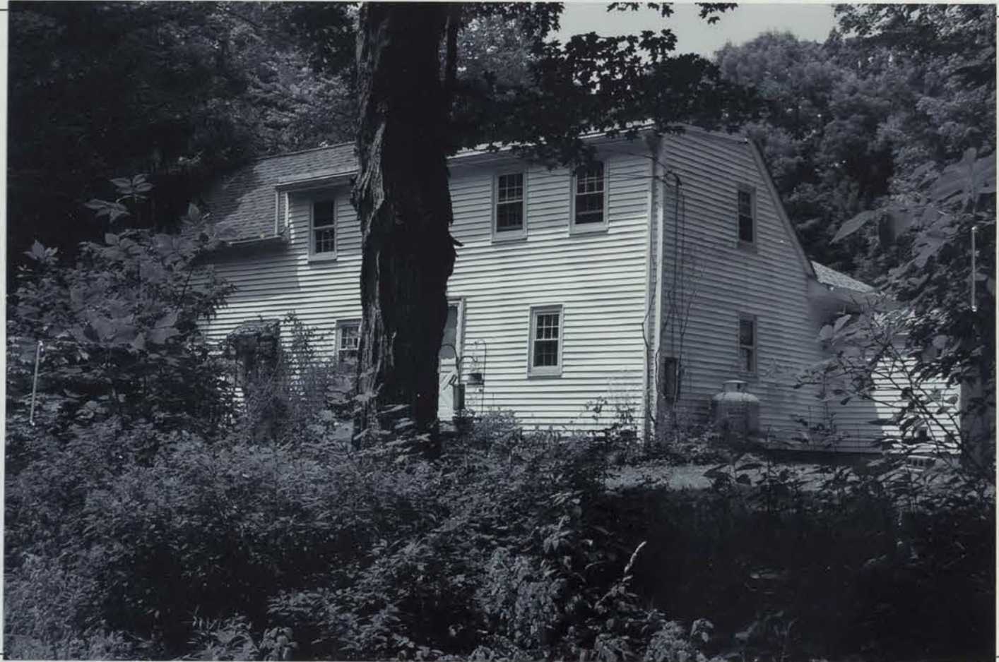
Photo #27 Description: 32 Bennett Road (#10), façade Direction: NW
