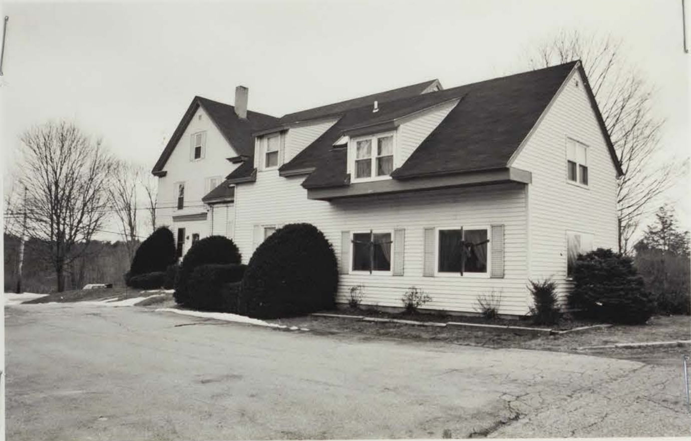
Photo #35 Description: Hale Stevens Farmhouse, south elevation Roll: 3 Frame: 23A Direction: NW
