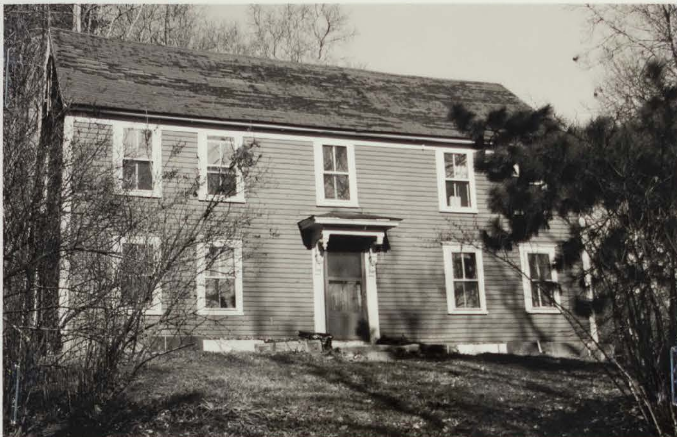
Photo #3 Description: Moriarty House, 4 Bennett Road (#2), facade Roll: 1 Frame: 10 Direction: N
