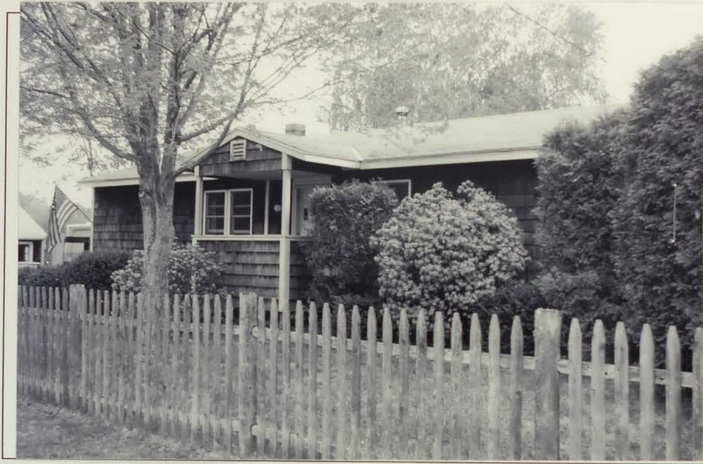
Photo #5 Description: Binette House, 103 Newmarket Road (#2) Direction: E
