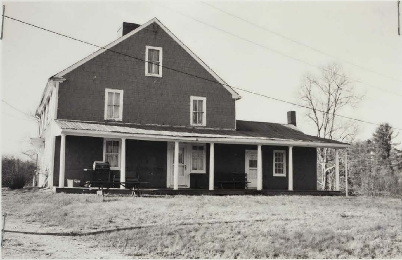
Photo #7 Description: Mooney-Beaudet Farmhouse, east elevation Roll: 1 Frame: 7 Direction: W
