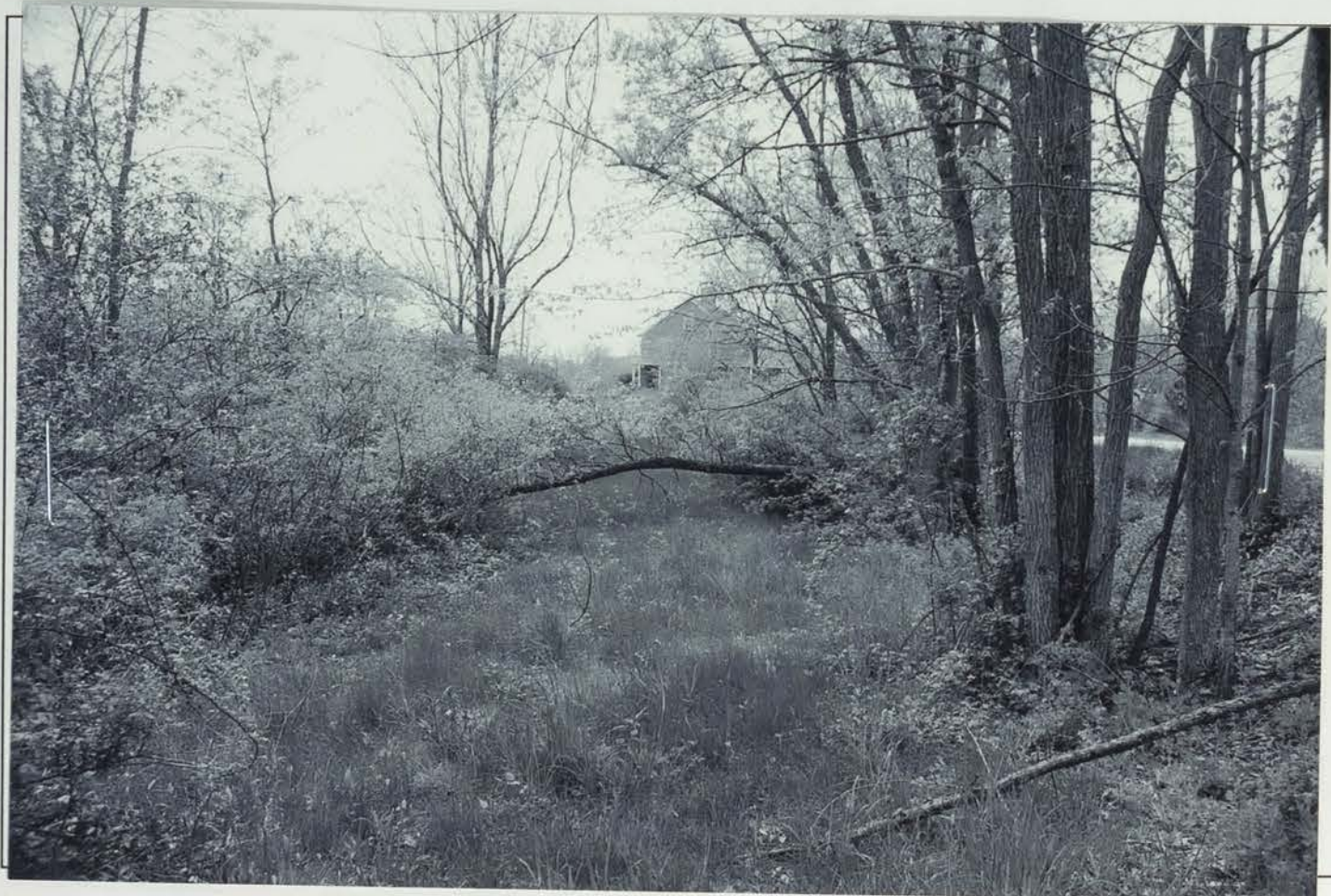
Photo #14 Description: Roadbed of Bennett Road prior to early 1960s realignment, showing Mooney-Beudet Farmhouse (#8) in rear
