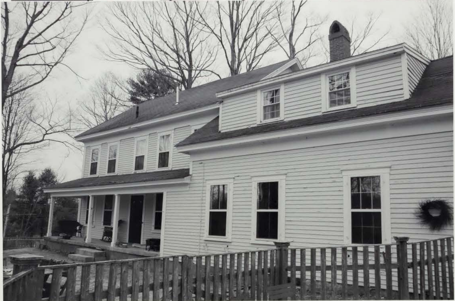
Photo 2: Façade and ell from driveway
