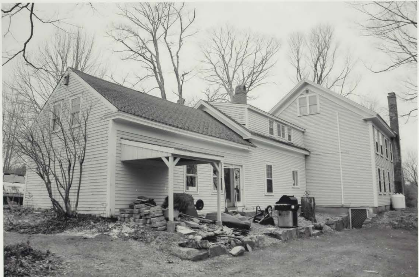
Photo 3: Rear of ell and house
