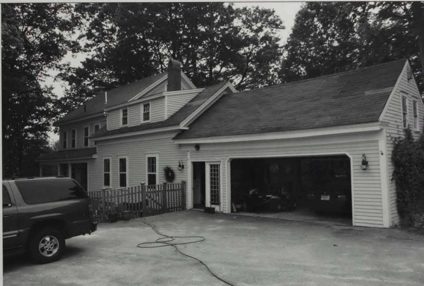
Photo 4. Rear view showing front (east) elevation with attached wings (kitchen and garage). Looking: SW Image file: DUR000_04
