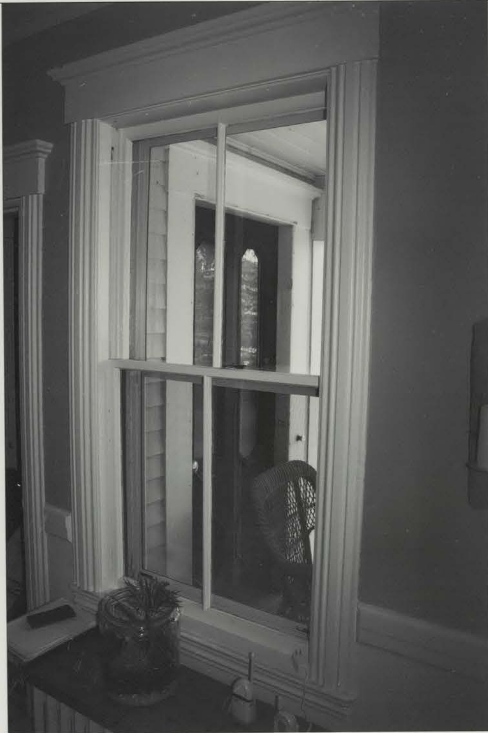
Photo 9. First-floor window with later 2/2 sash; note side-entrance door with twin lights through window.
