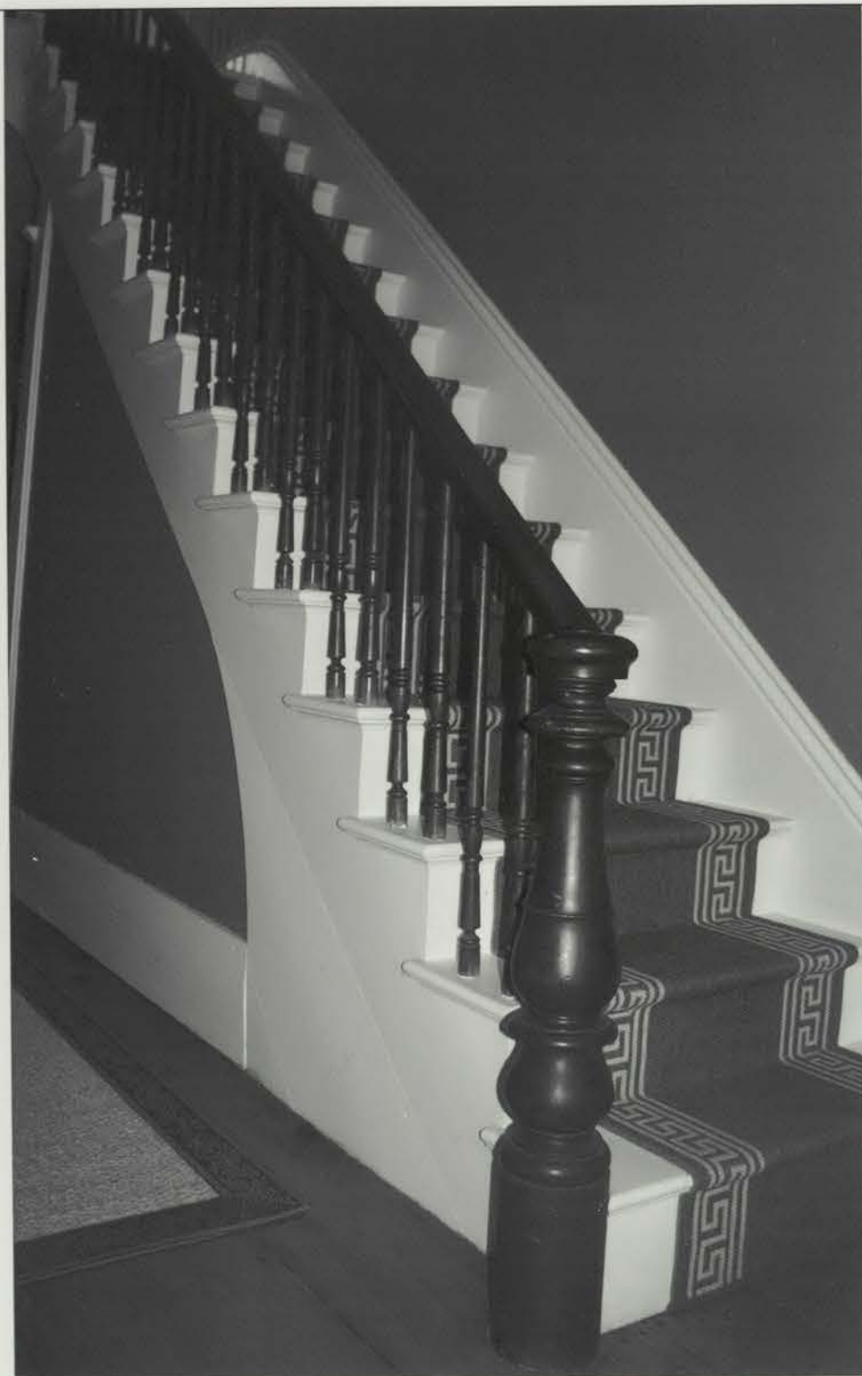
Photo 7. First-floor staircase with newel post and banister; note pine floors. Looking: NW Image file: DUR000_07
