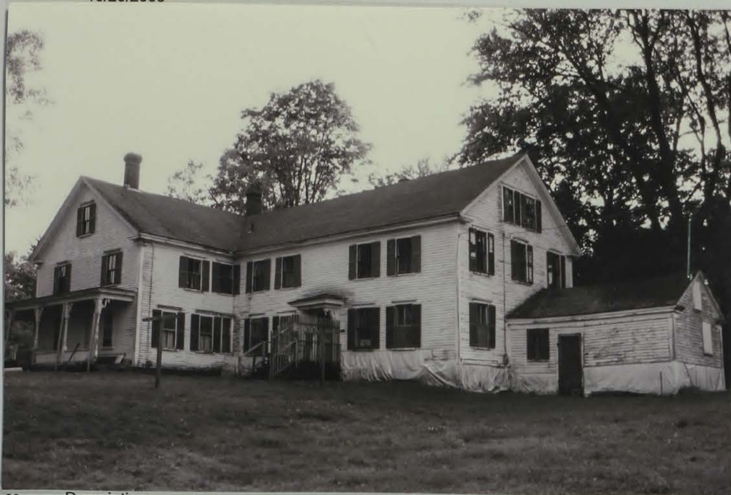
Photo # 20 Description: East facade with attached shed prior to renovations that began in 10/2006. Reference (file name or frame#):: East Facade with attached shed later removed. Direction: Southwest
