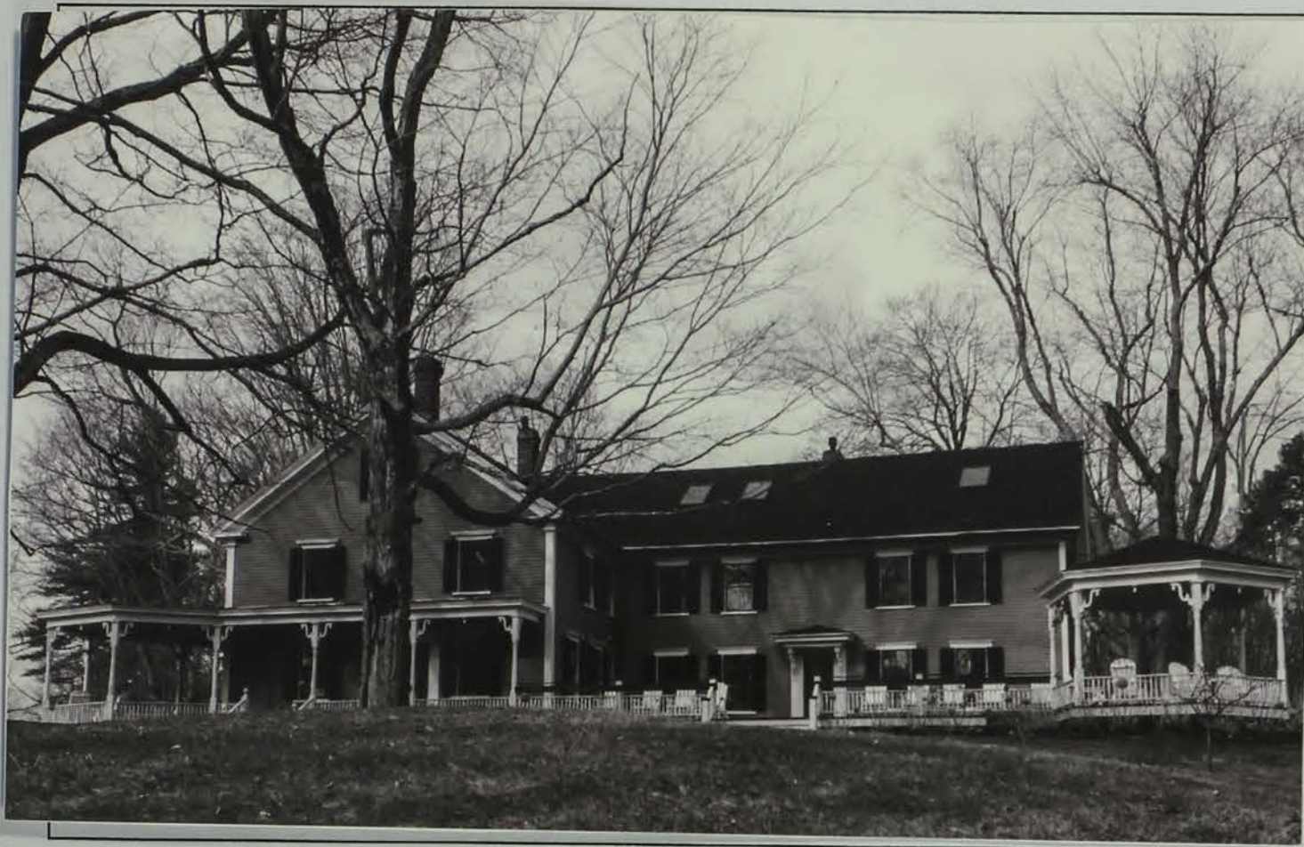
Photo # 4 Description: East Facade of Highland House. Deck and Gazebo on right added in 2011. Skylights added in 2007. Reference (file name or frame#):: East Facade Direction: West
