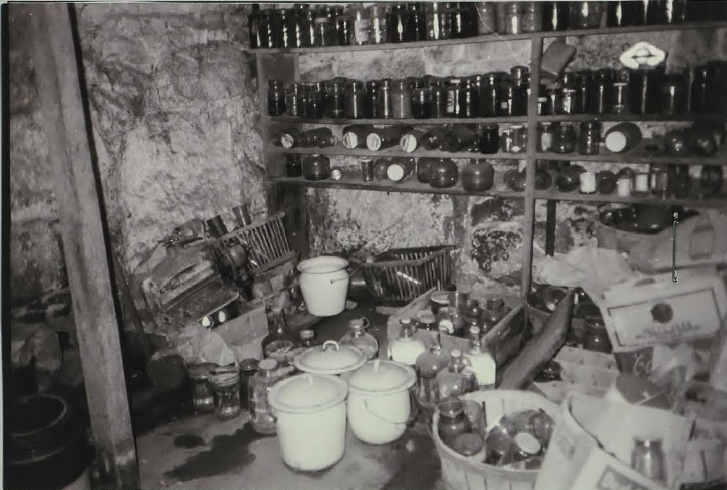
Photo # 32 Description: Whitewashed cold storage room in cellar with granite walls and floor Reference (file name or frame#):: Buttery in Cellar Direction: Norhtwest
