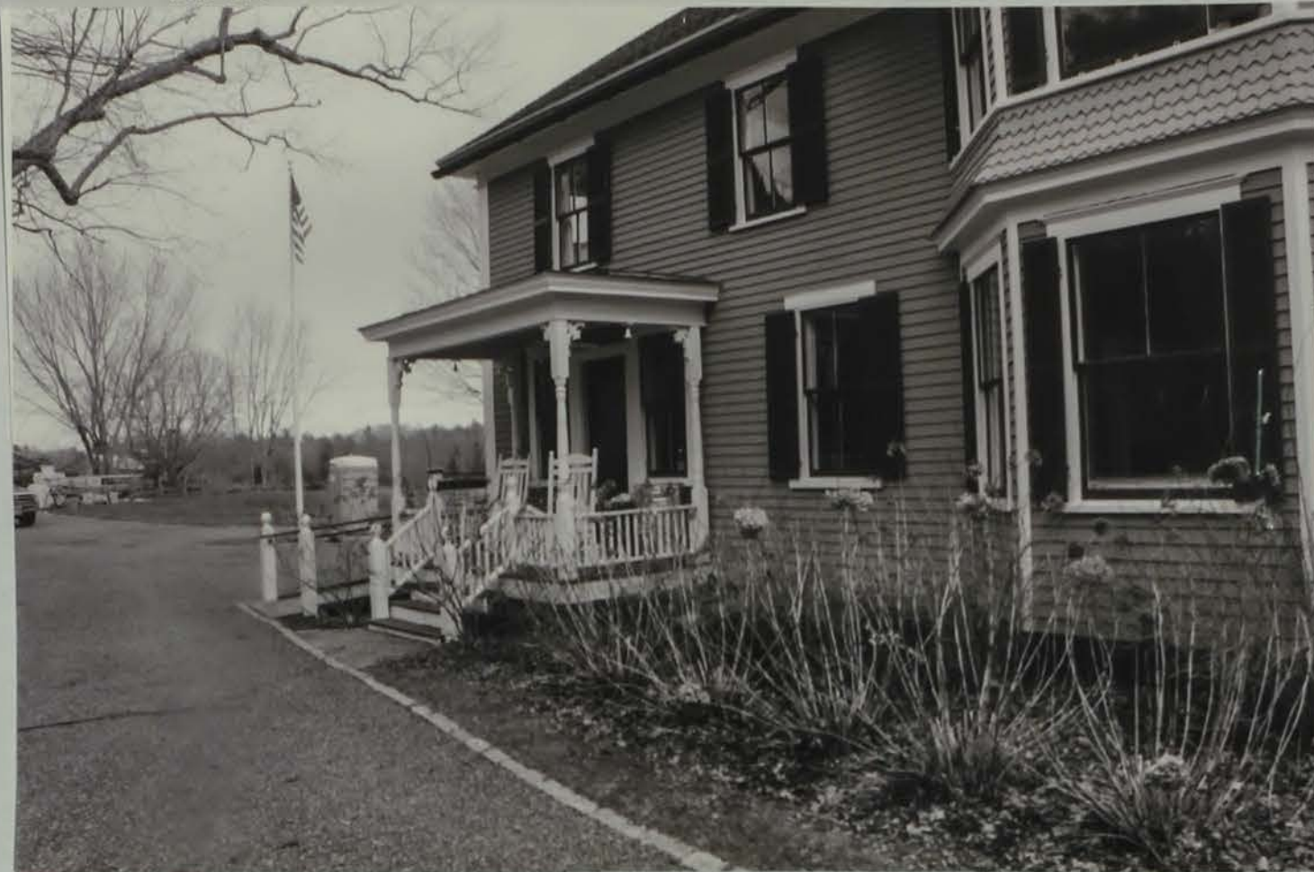
Photo # 22 Description: West facade with kitchen porch renovated in 2007 and bay window dormer. Reference (file name or frame#):: IMG 4465 Direction: North
