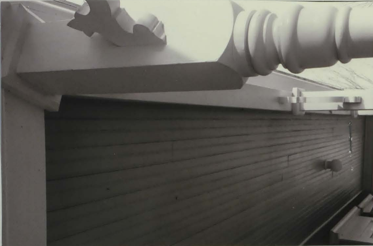
Photo # 28 Description: Preserved beadboard veranda ceiling and post detail.
