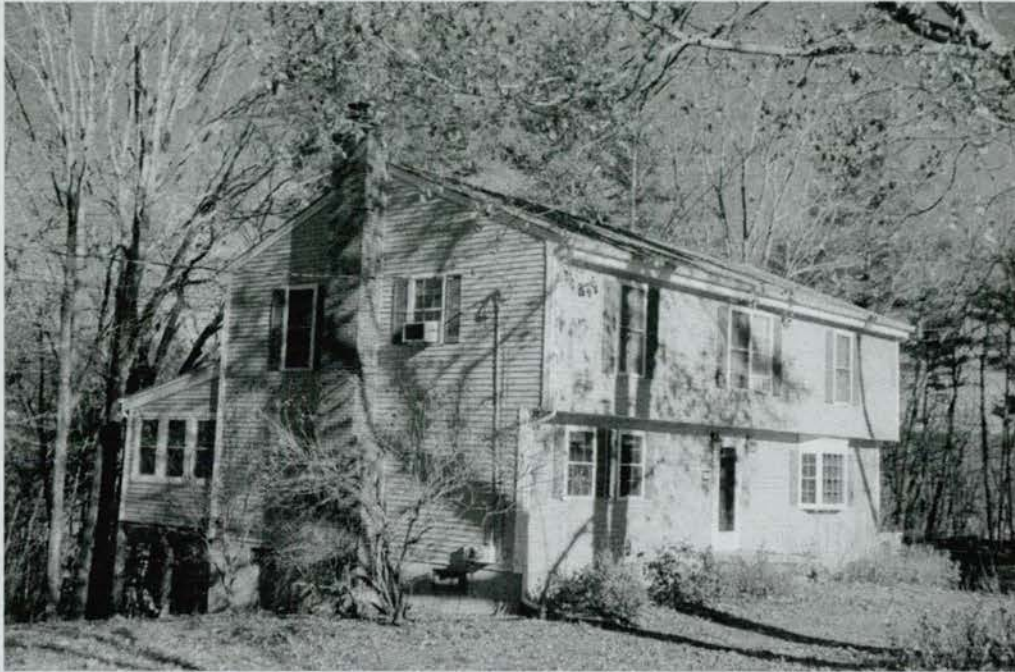
Wedgewood Development – 29 Pinecrest Lane, Durham
