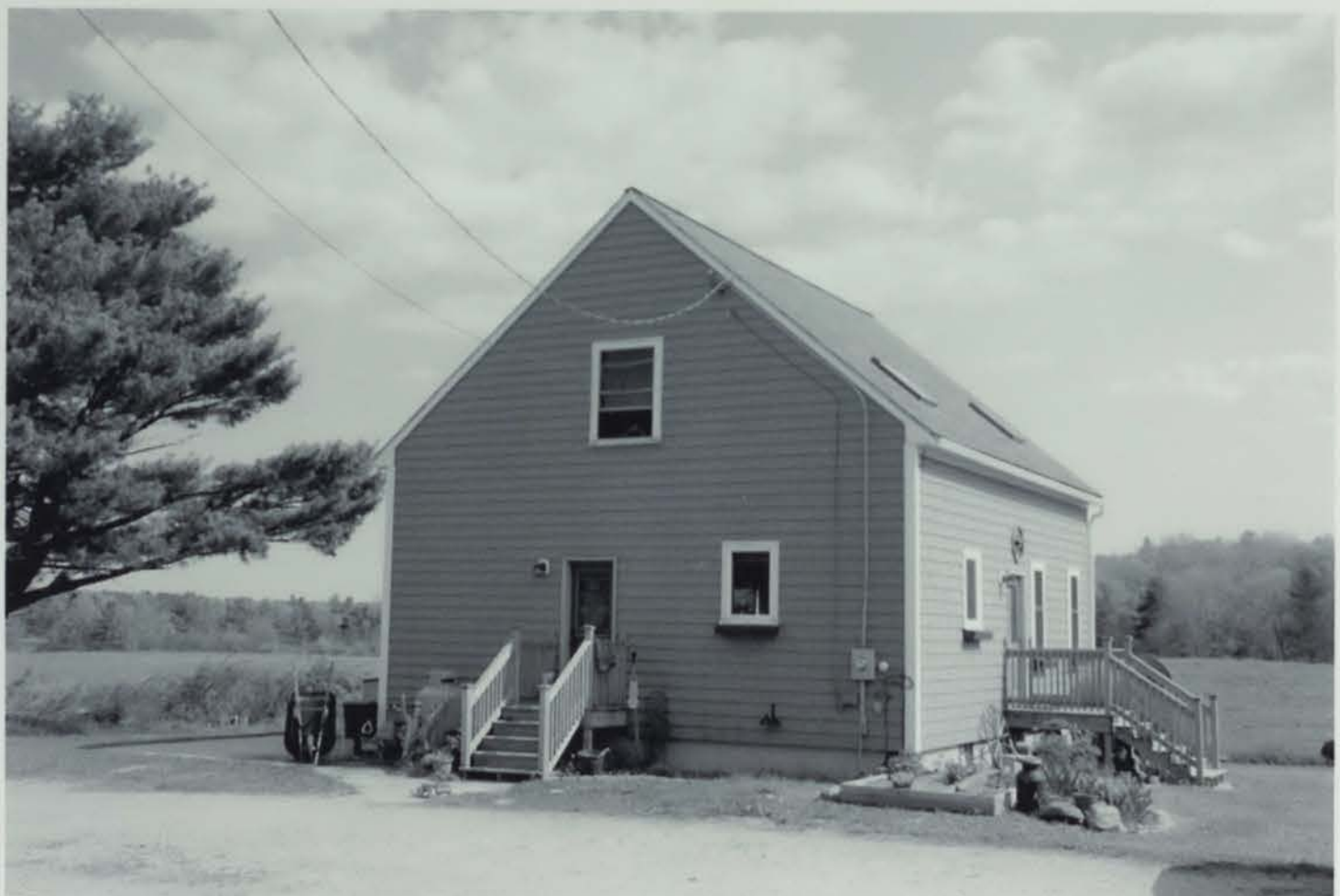
Photo 73) 50 Langley Road house-shop Date taken: May 2016
