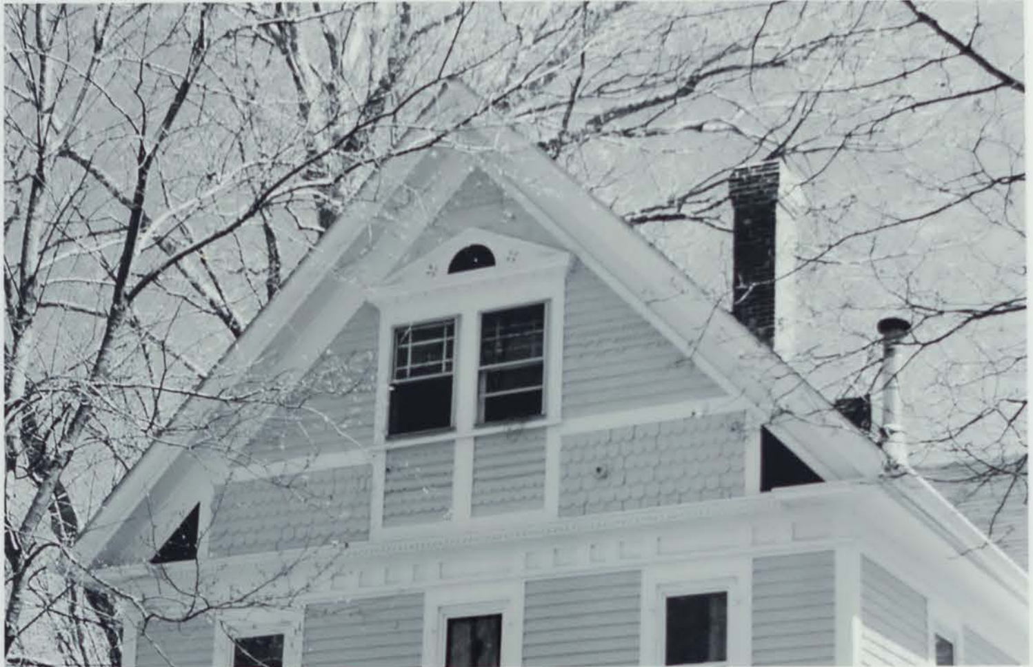
Detail of Photo 16, 253 Durham Point Road, gable detail (NE) Date taken: April 2016
