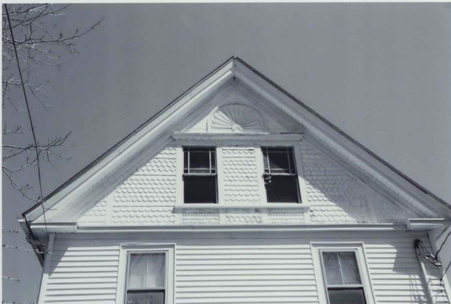
Photo 24) 247 Durham Point Road, gable detail Date taken: April 2016
