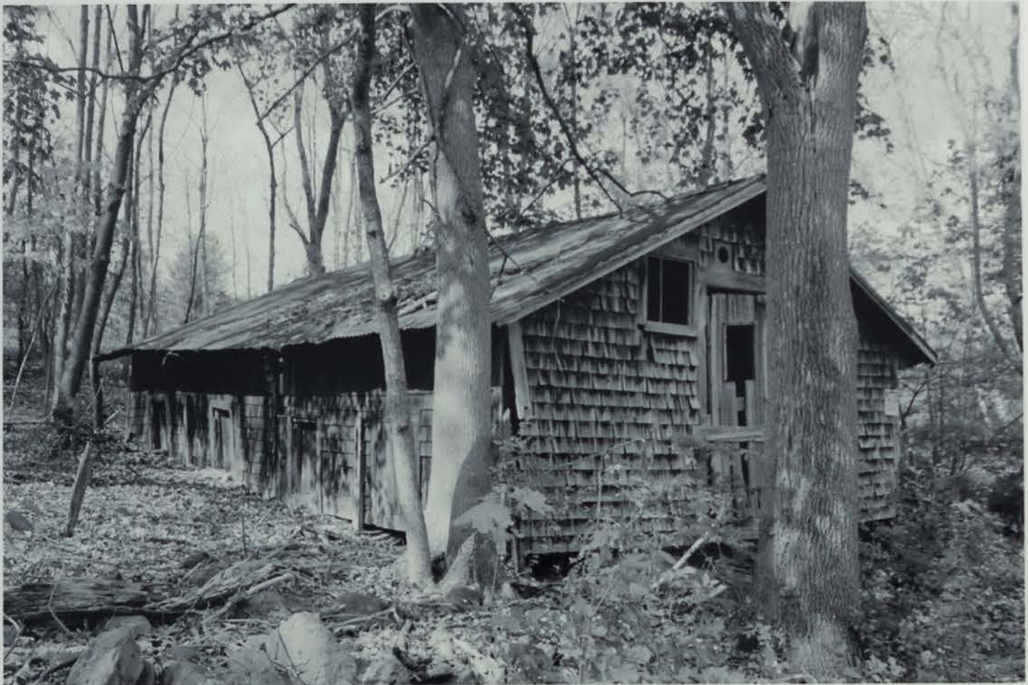
Photo 68) Shed on parcel 12-12-00 Date taken: May 2016
