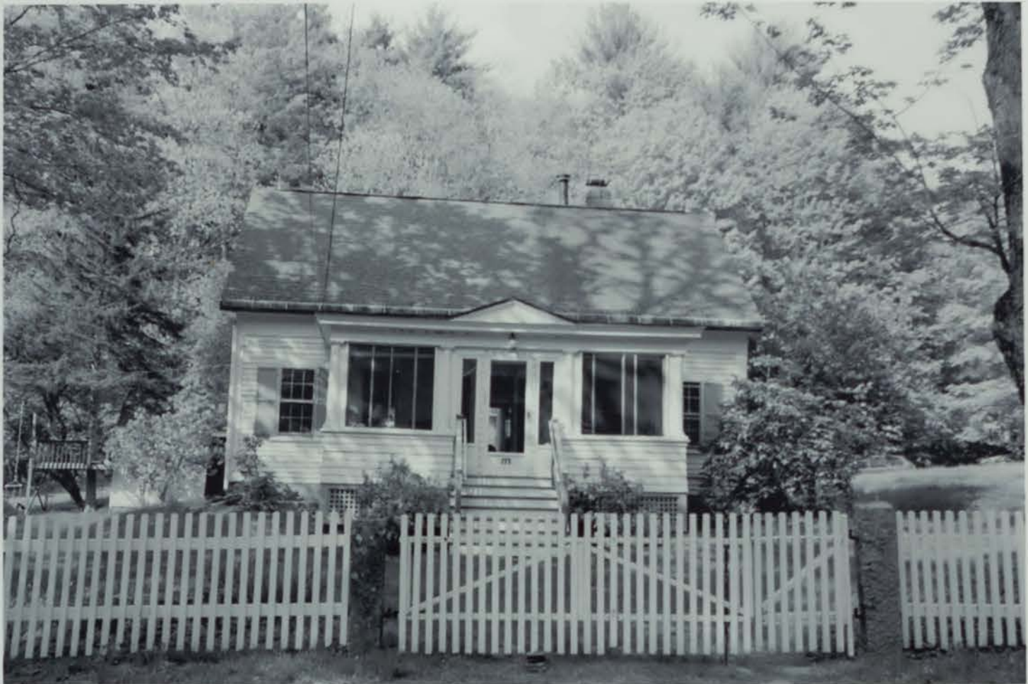
Photo 48) 177 Durham Point Road façade Date taken: May 2016
