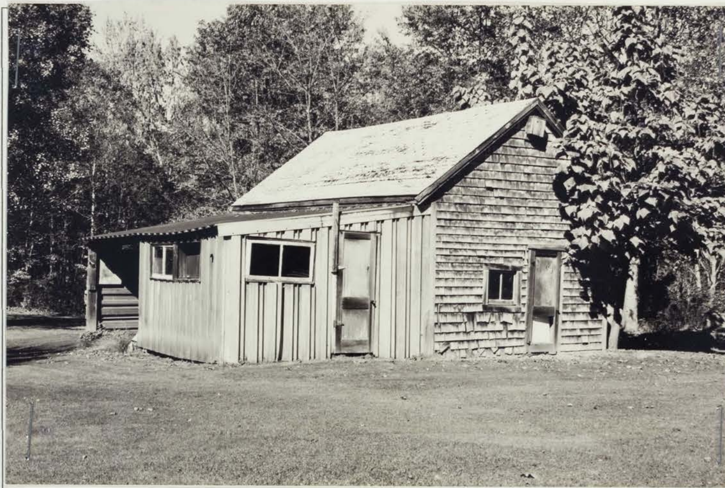
Photo 6 description: Shed/shop Roll: 1 Frame: 4 Direction: NW
