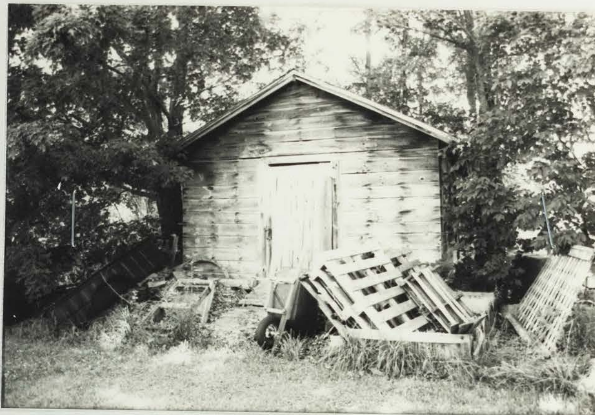
Photo # 8 description: Shed Roll #: 1 Frame #: 13 Direction: SW
