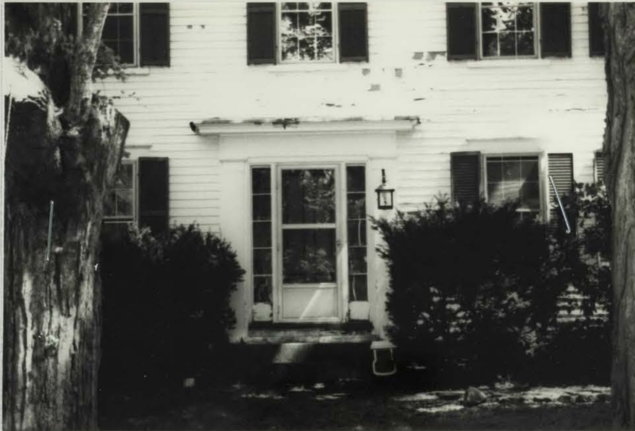
Photo # 4 description: Detail, front entrance Roll #: 1 Frame #: 5 Direction: SE
