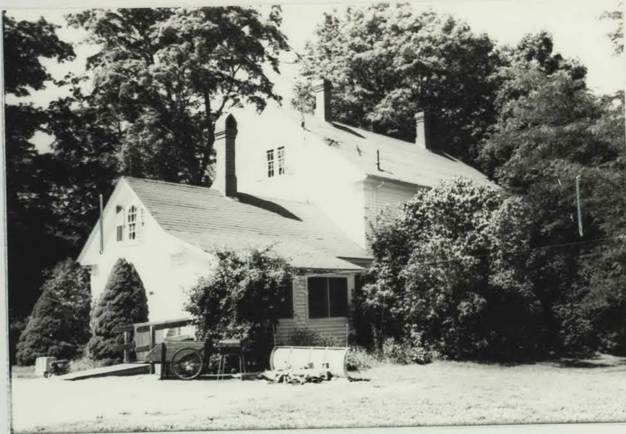
Photo # 6 description: East (rear) elevation Roll #: 1 Frame #: 15 Direction: north
