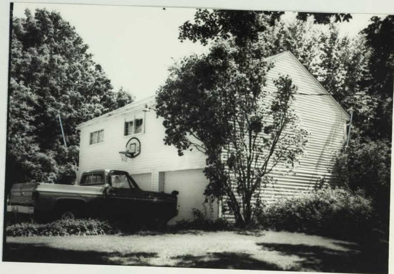
Photo # 7 description: Garage Roll #: 1 Frame #: 1 Direction: south
