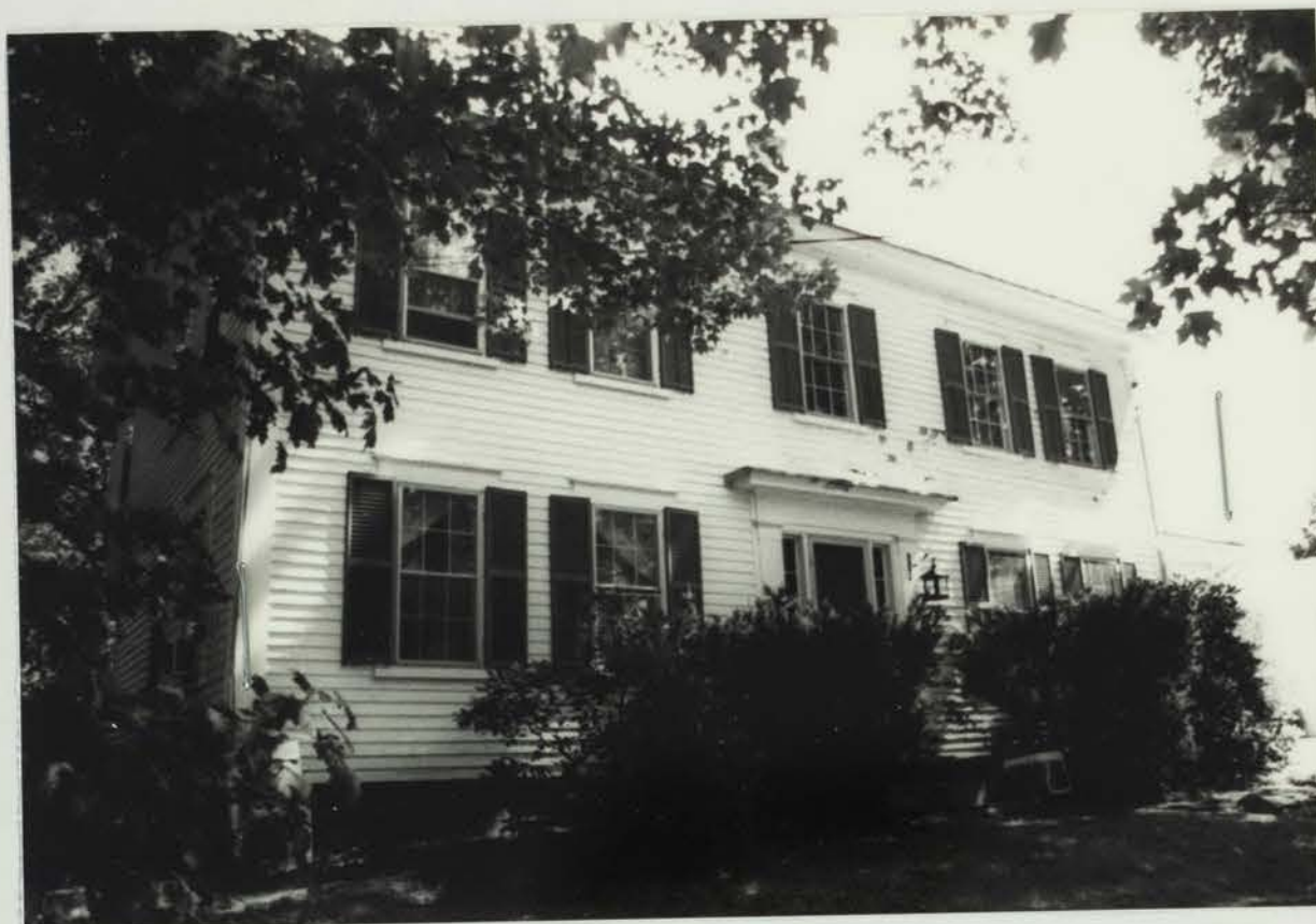
Photo # 2 description: West facade Roll #: 1 Frame #: 6 Direction: south
