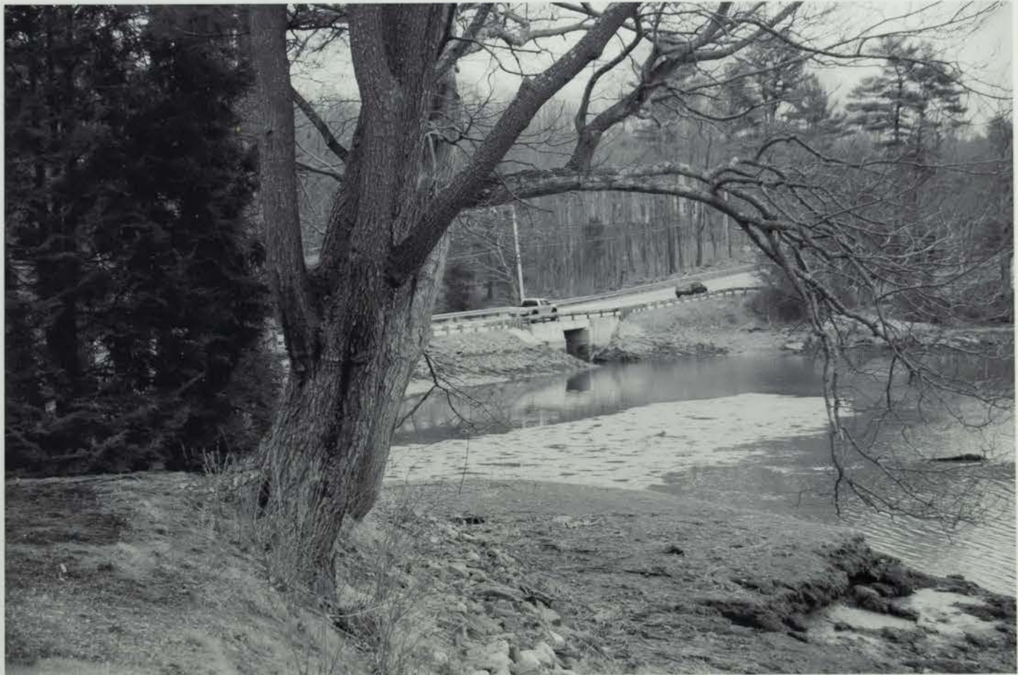
Photo 1: Bunker Creek Bridge at mouth of Great Bay
