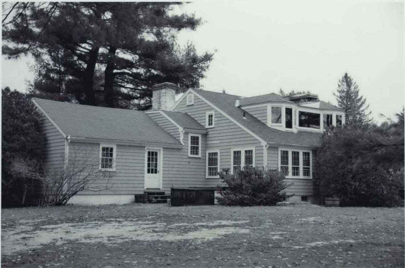
Photo 12: 100 Piscataqua Road, rear (garage and main block)
