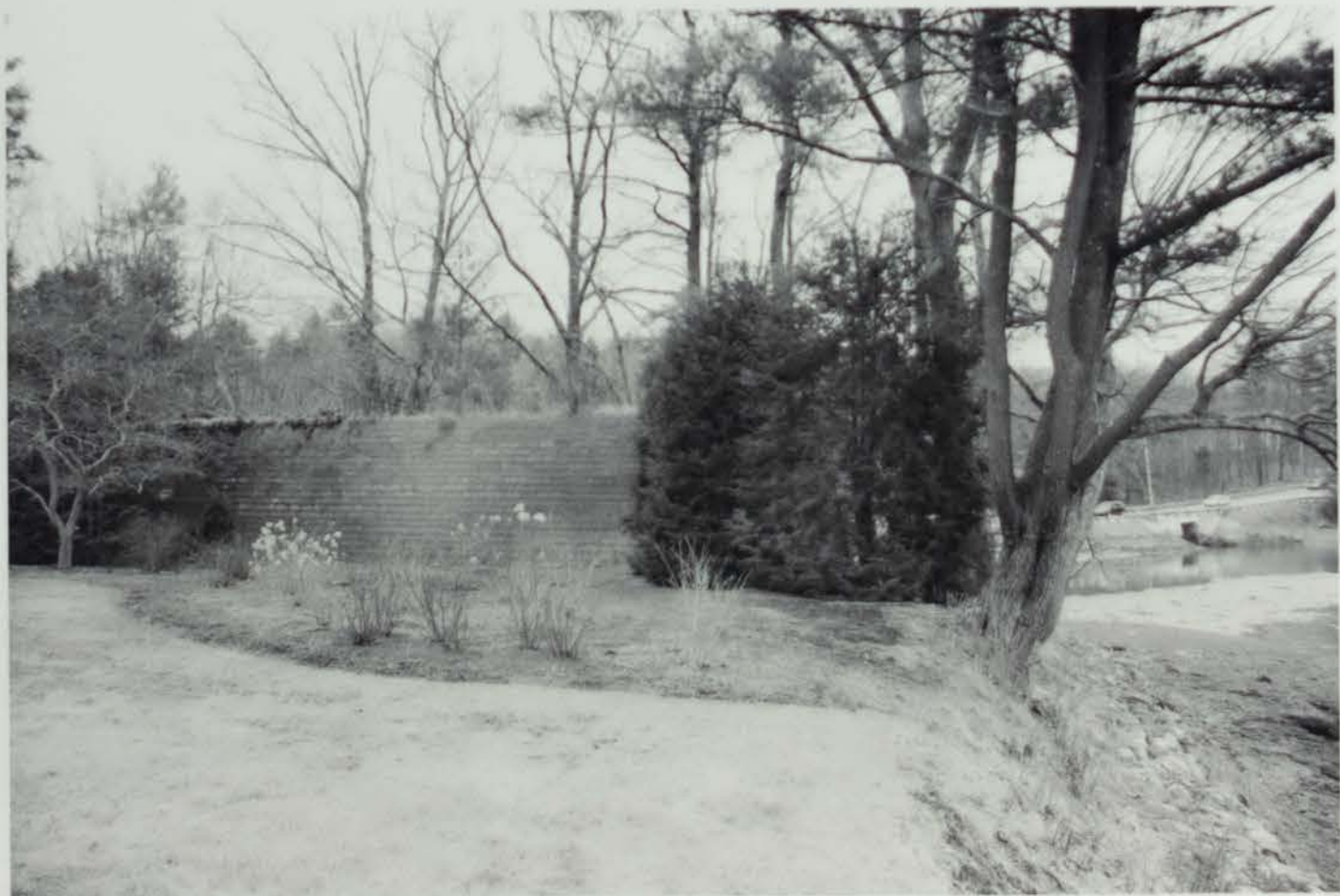
Photo 21: 104 Piscataqua Road, masonry wall and berm along Bunker Creek
