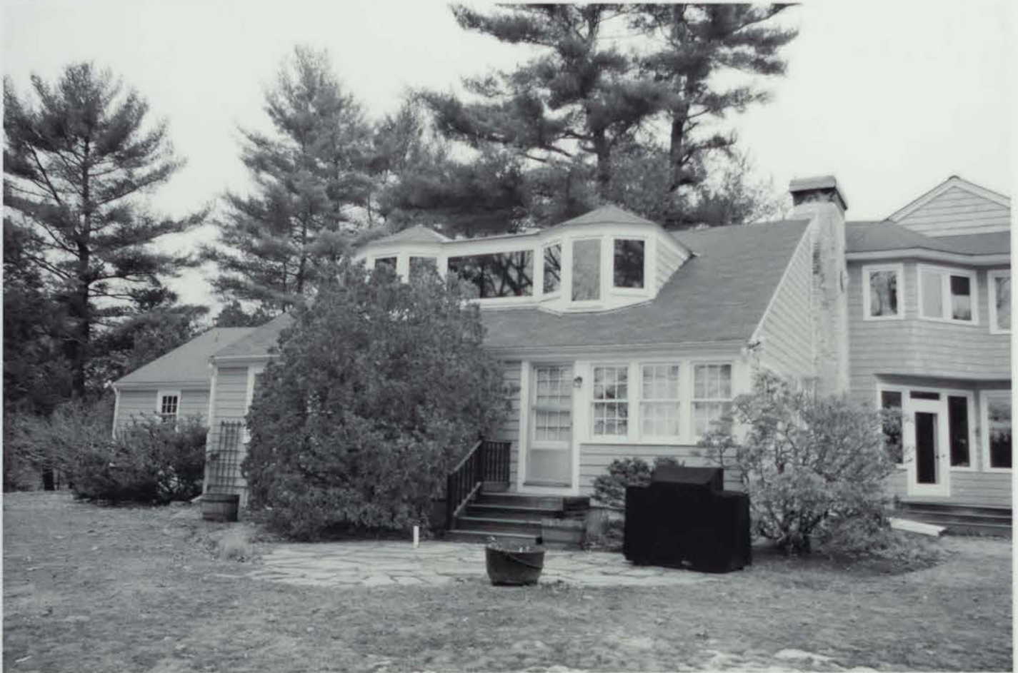
Photo 14: 100 Piscataqua Road, addition
