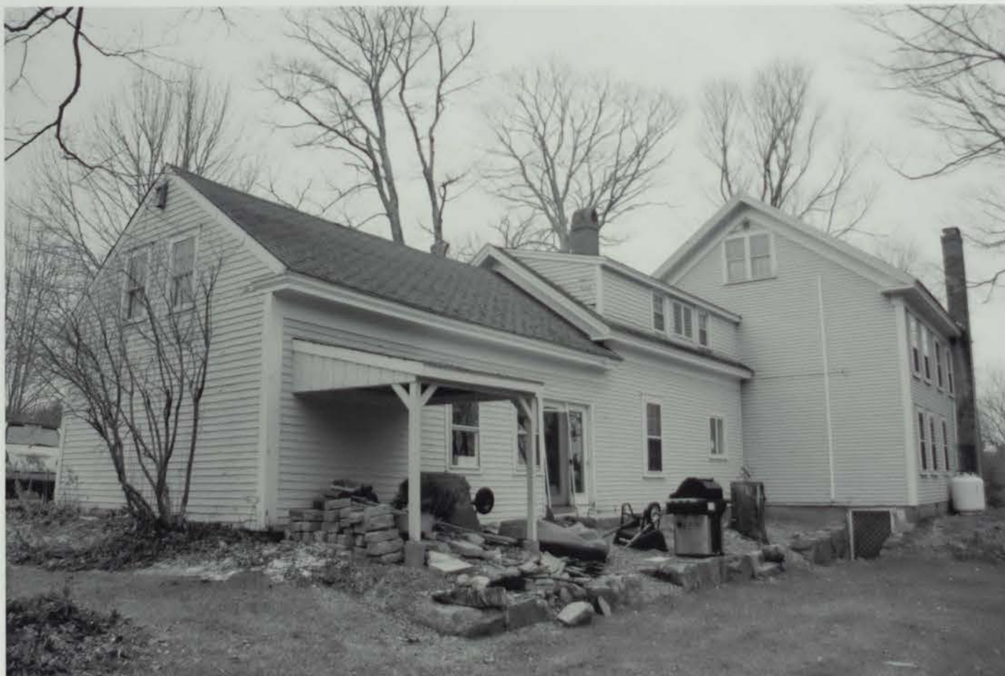
Photo 9: 3 Williams Way, rear of ell and house
