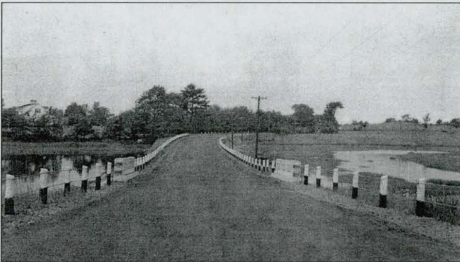
"East approach, looking towards Durham," ca. 1940 photograph of the original appearance of the roadbed of the 1933 Bunker Creek Bridge, from NHDOT bridge files.
