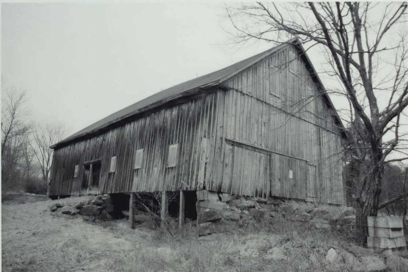
Photo 5: 5 Bunker Lane, rear of barn
