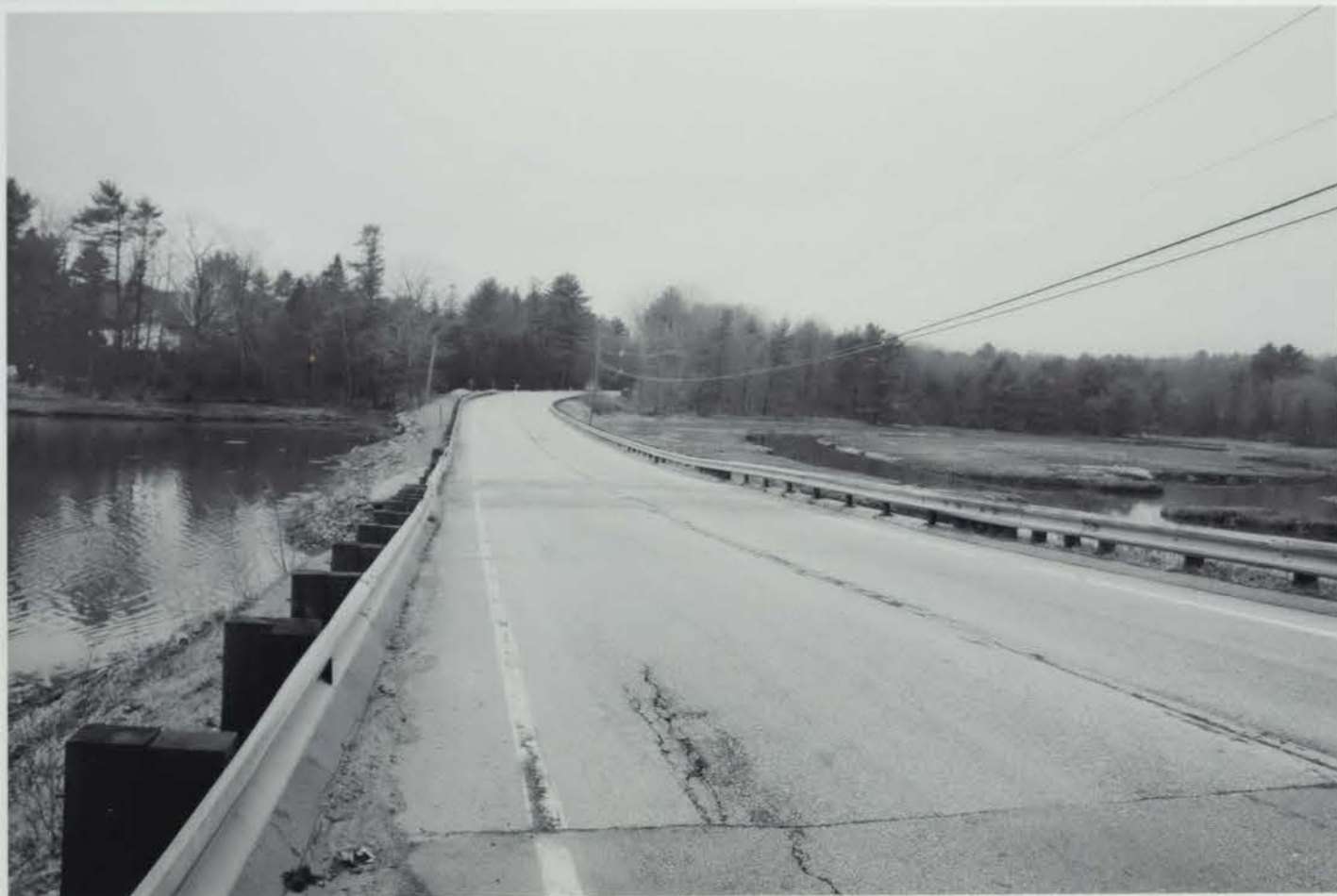
Photo 2: Bunker Creek Bridge overpass
