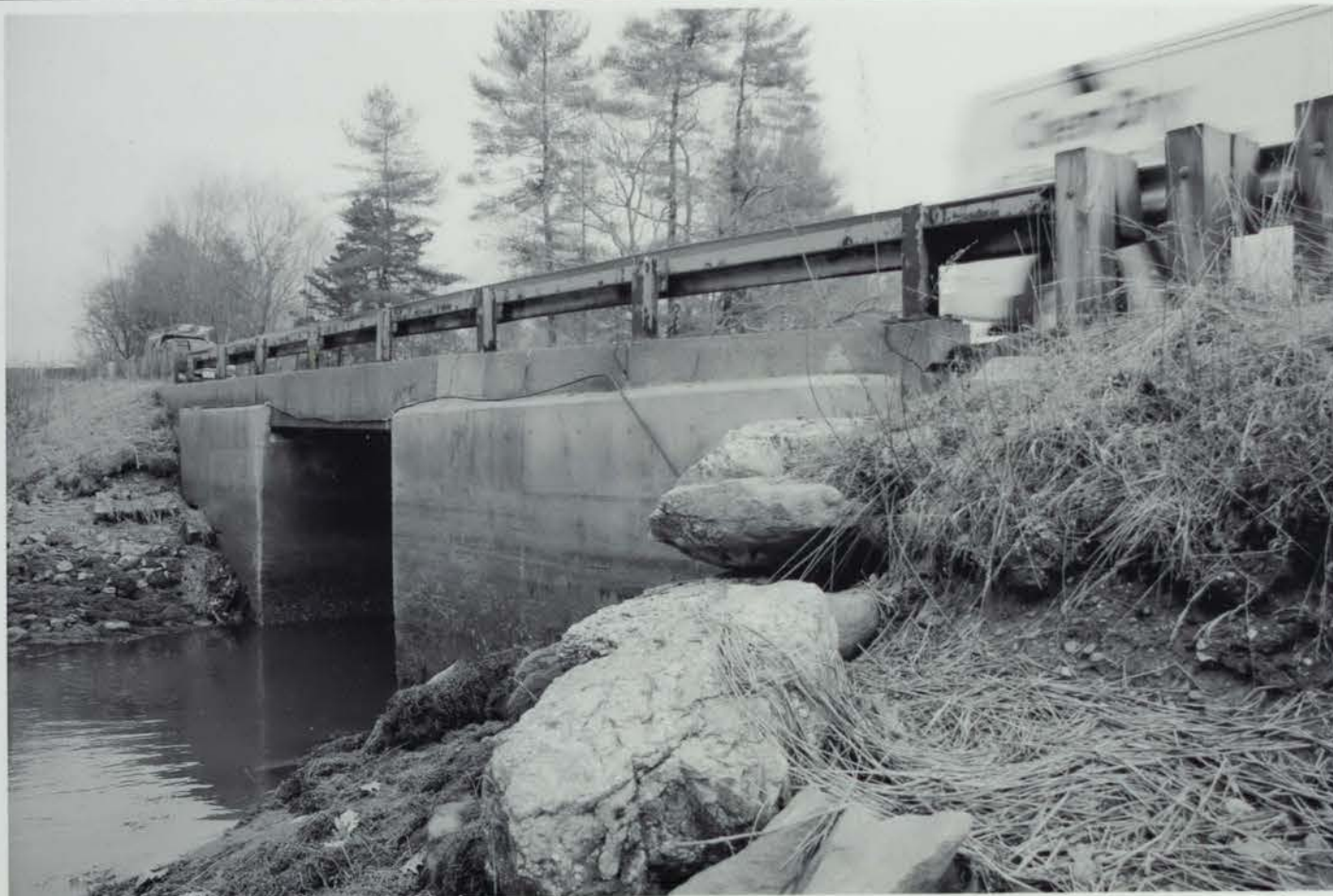
Photo 24: Bunker Creek Bridge, north abutments
