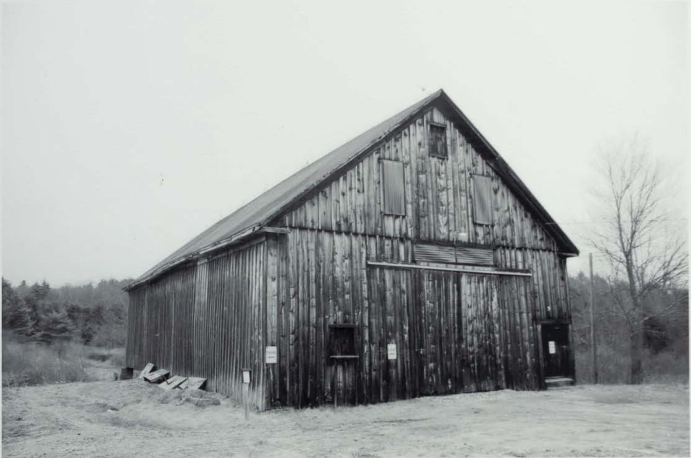
Photo 4: 5 Bunker Lane, barn façade
