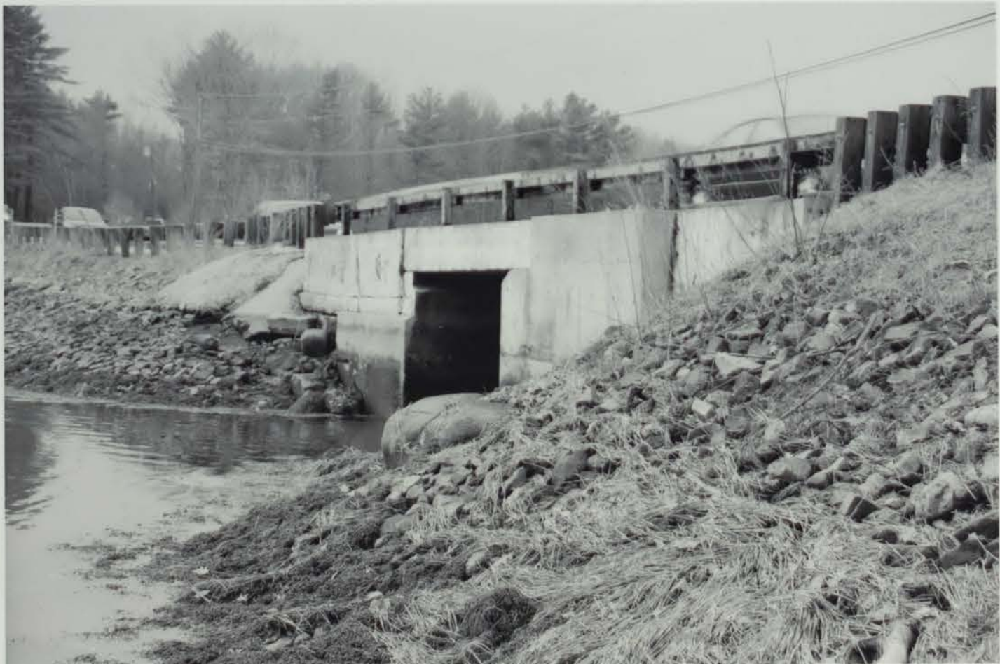
Photo 23: Bunker Creek Bridge, south abutments
