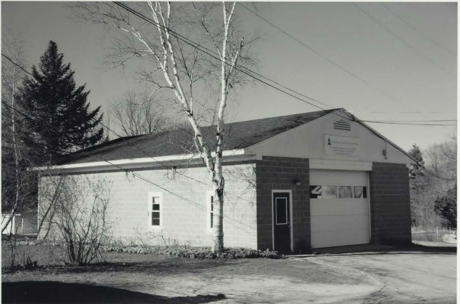
Photo 7: Cold storage building
