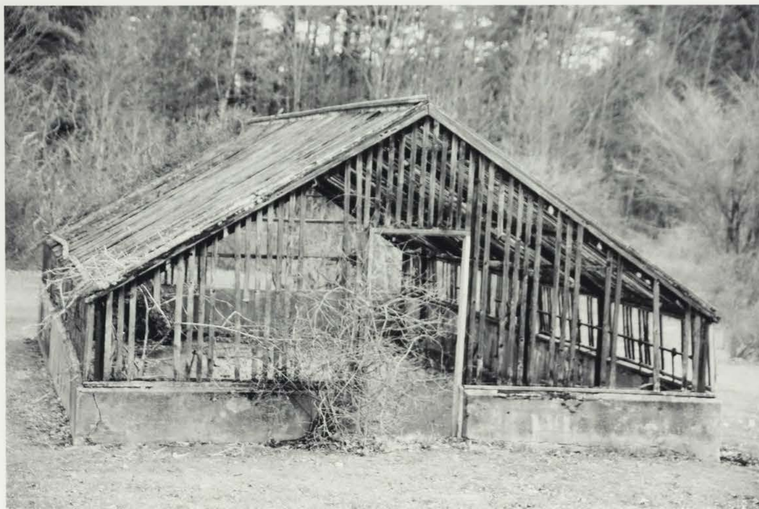
Photo 9: Old greenhouse with iron frame
