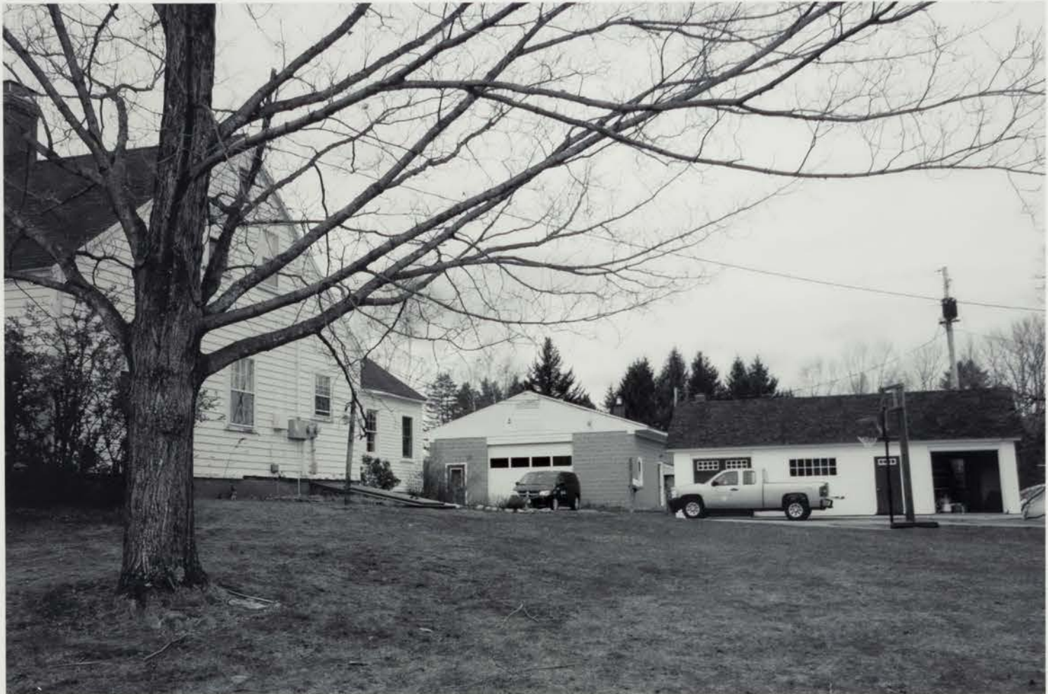
Photo 4: Northeast gable end of house and outbuildings north of farmhouse
