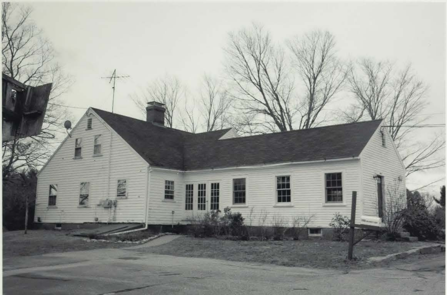
Photo 3: Northeast gable end of farmhouse and rear ell
