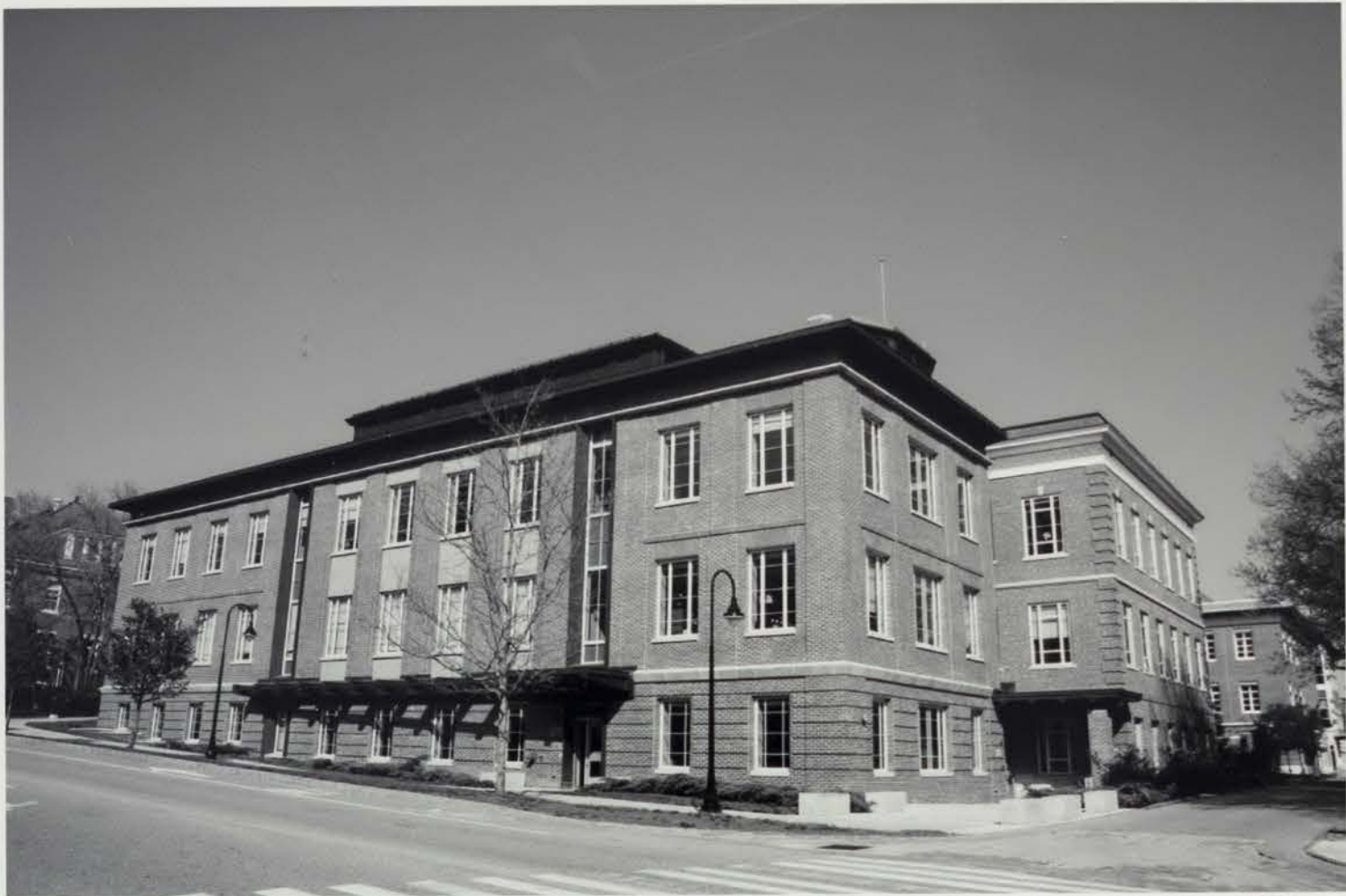
Photo 014) 56 College Road – James Hall photo taken May 2016
