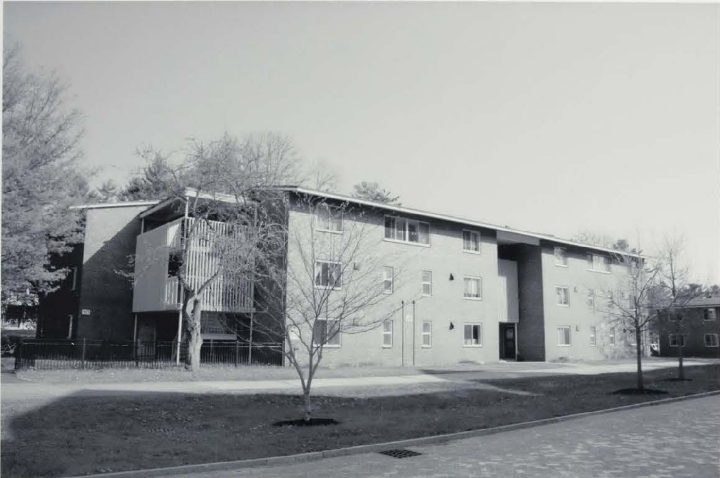
Photo 065) 4 Demeritt Circle – Forest Park Apartments photo taken May 2016
