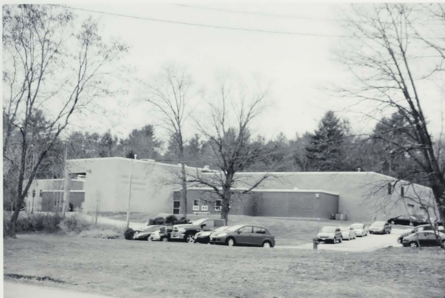
Photo 075) 24 Colovos Road – Chase Ocean Engineering Laboratory photo taken December 2015
