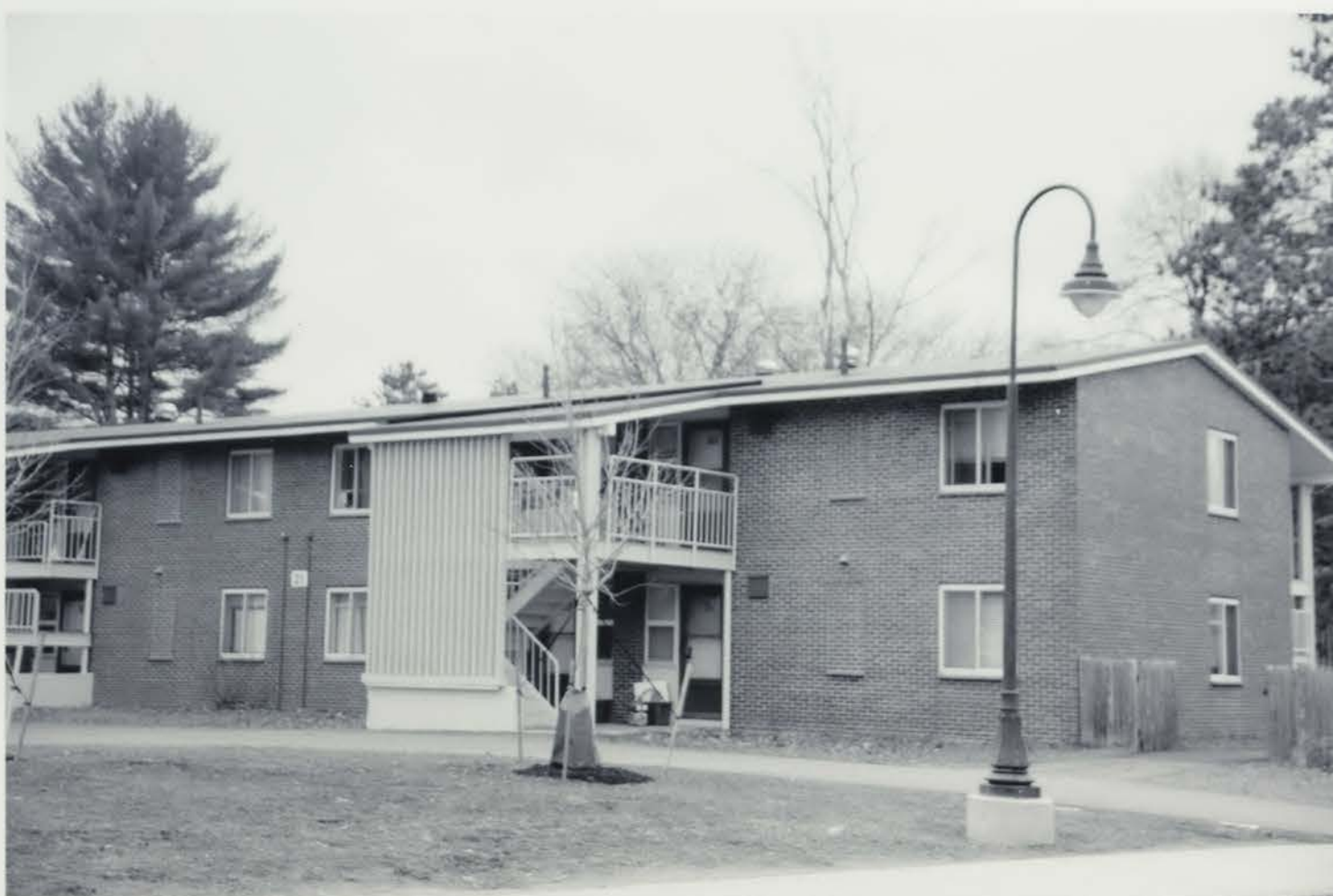
Photo 062) 4 Demeritt Circle – Forest Park Apartments photo taken December 2015
