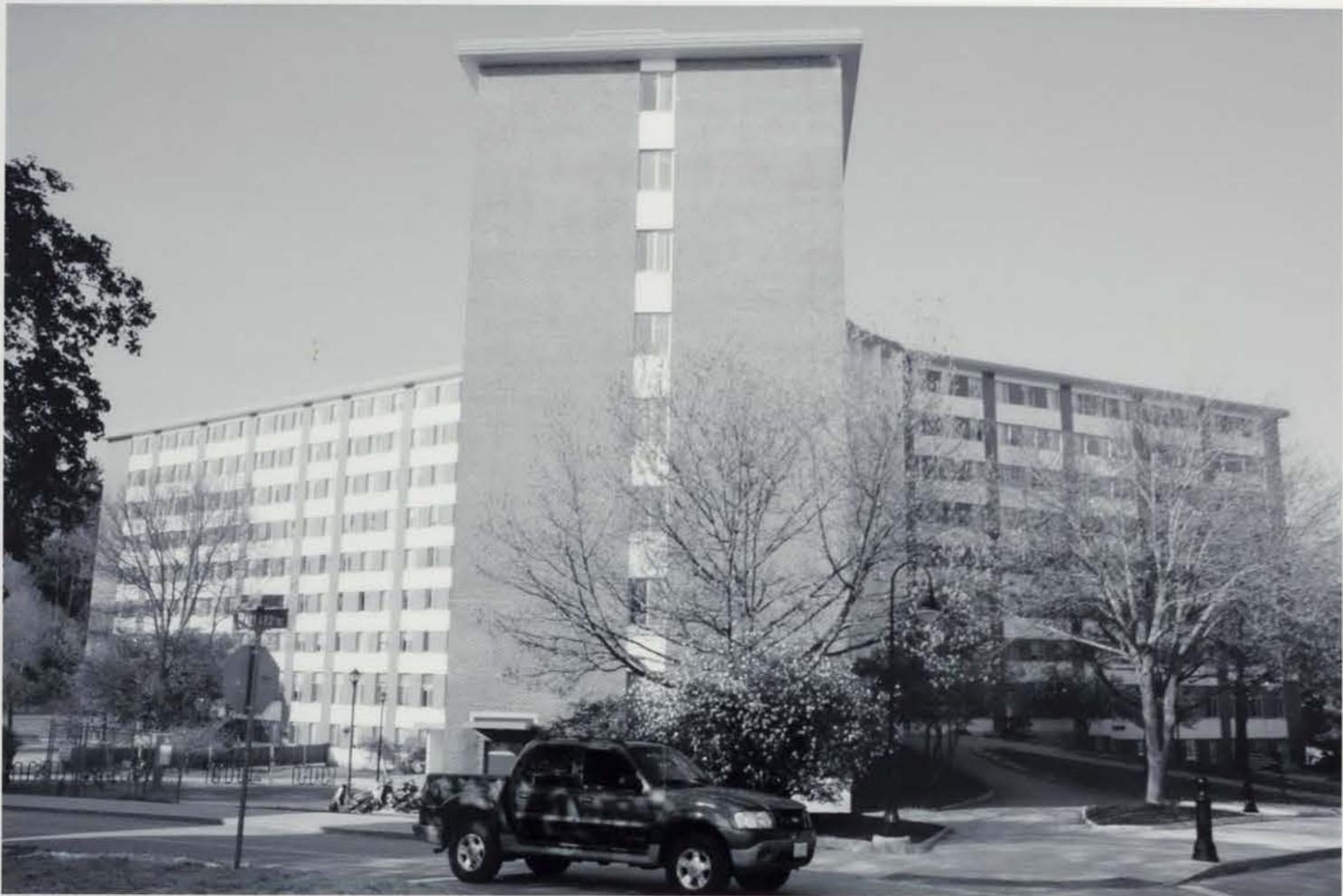
Photo 055) 11 Garrison Avenue – Stoke Hall photo taken May 2016
