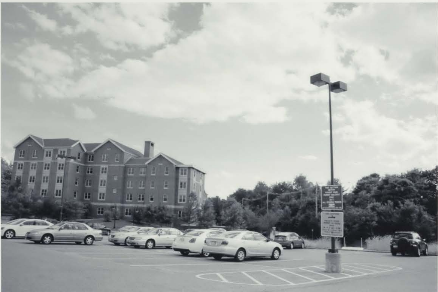
Photo 070) 5 Demeritt Circle – Handler Hall, railroad tracks at right Direction: S photo taken June 2015
