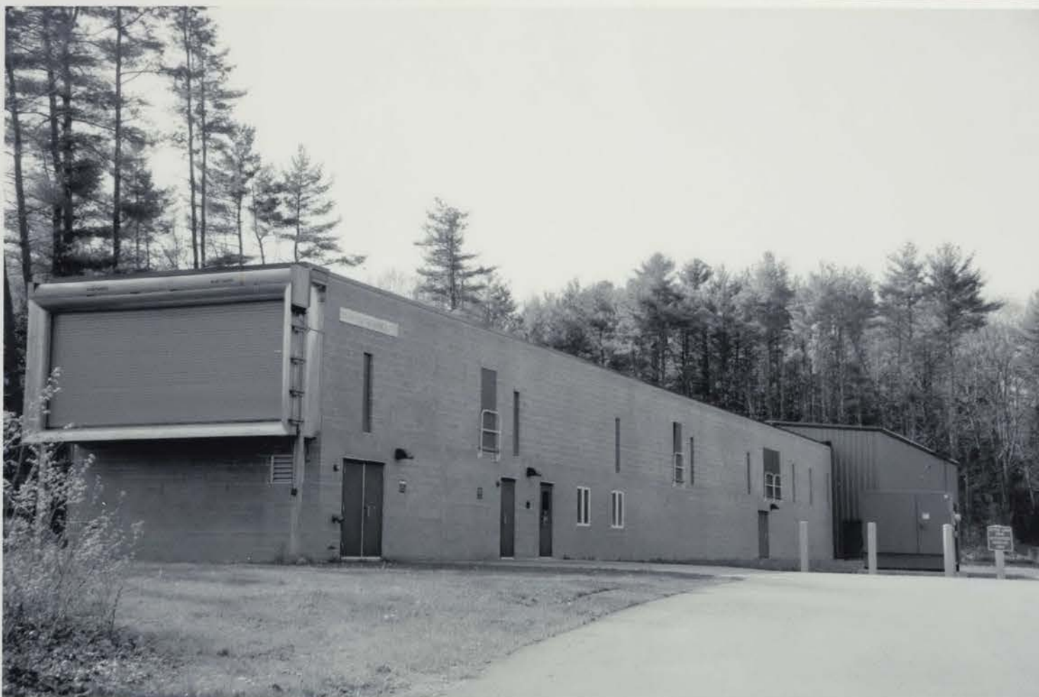
Photo 078) 24 Waterworks Road – Flow Physics Lab photo taken May 2016
