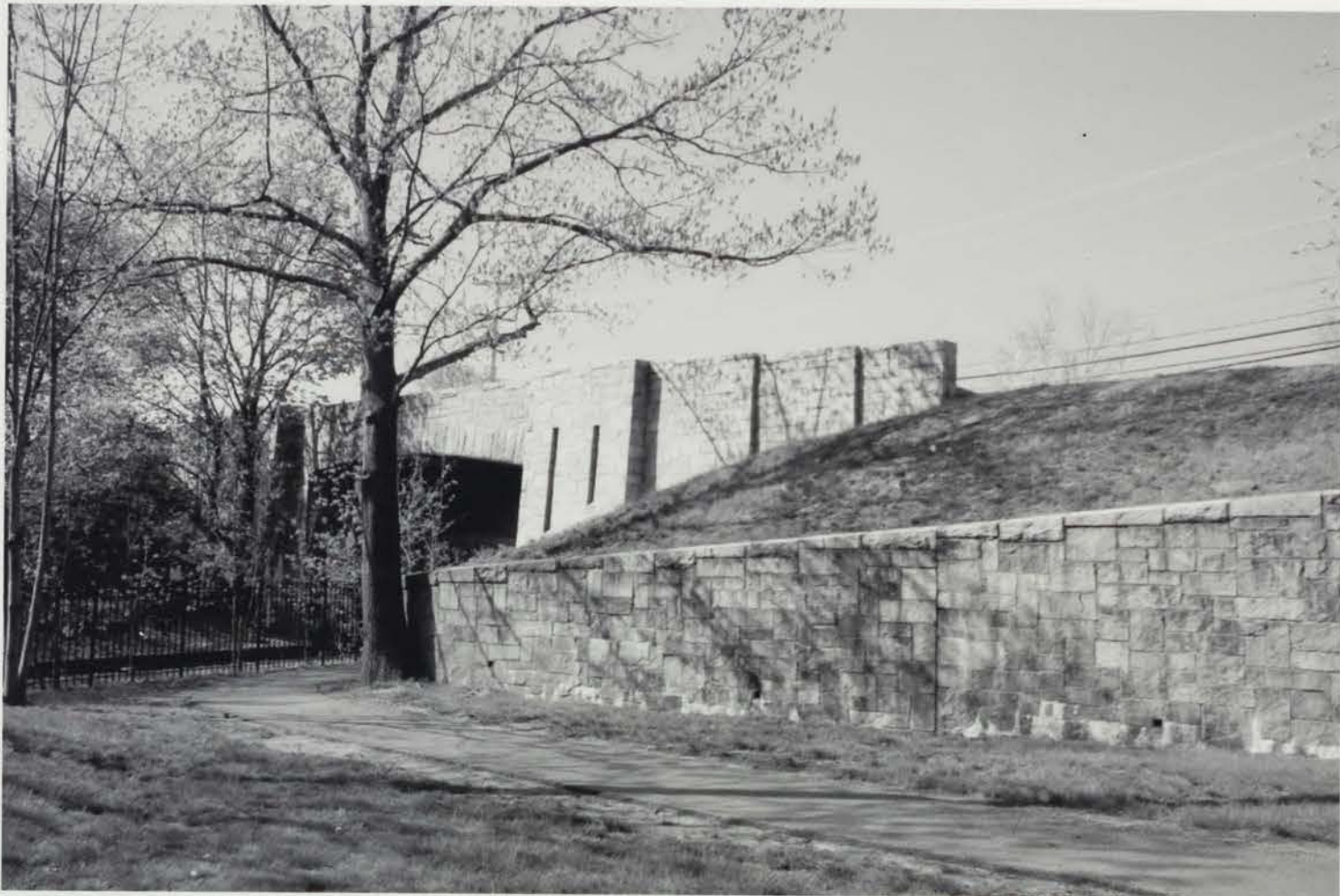
Photo 004) Main Street – Retaining wall in front of Nesmith Hall, railroad and bridge over Main Street to left photo taken May 2016 Direction: NW
