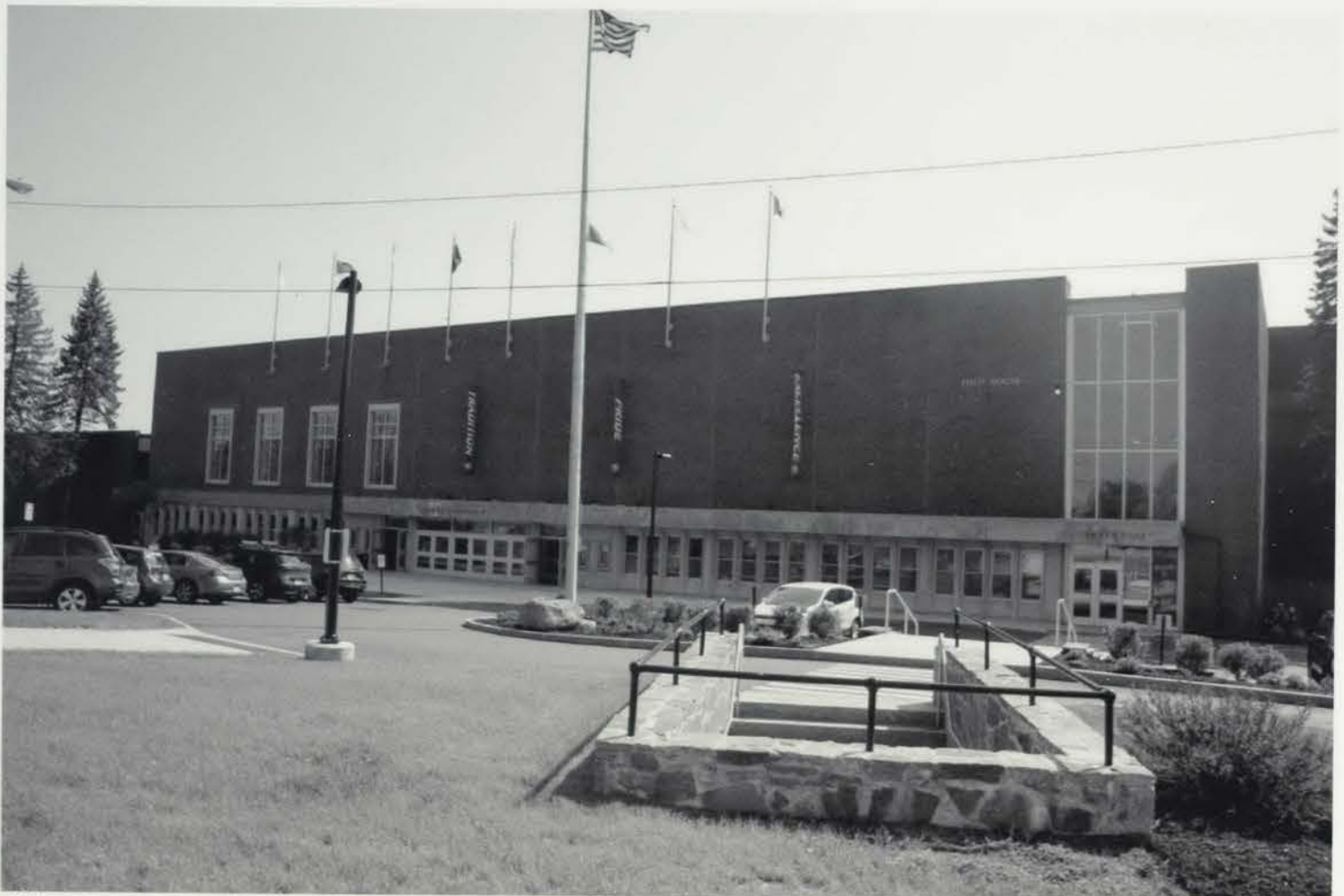
Photo 041) 145 Main Street – Fieldhouse/Lundholm Gymnasium photo taken May 2016
