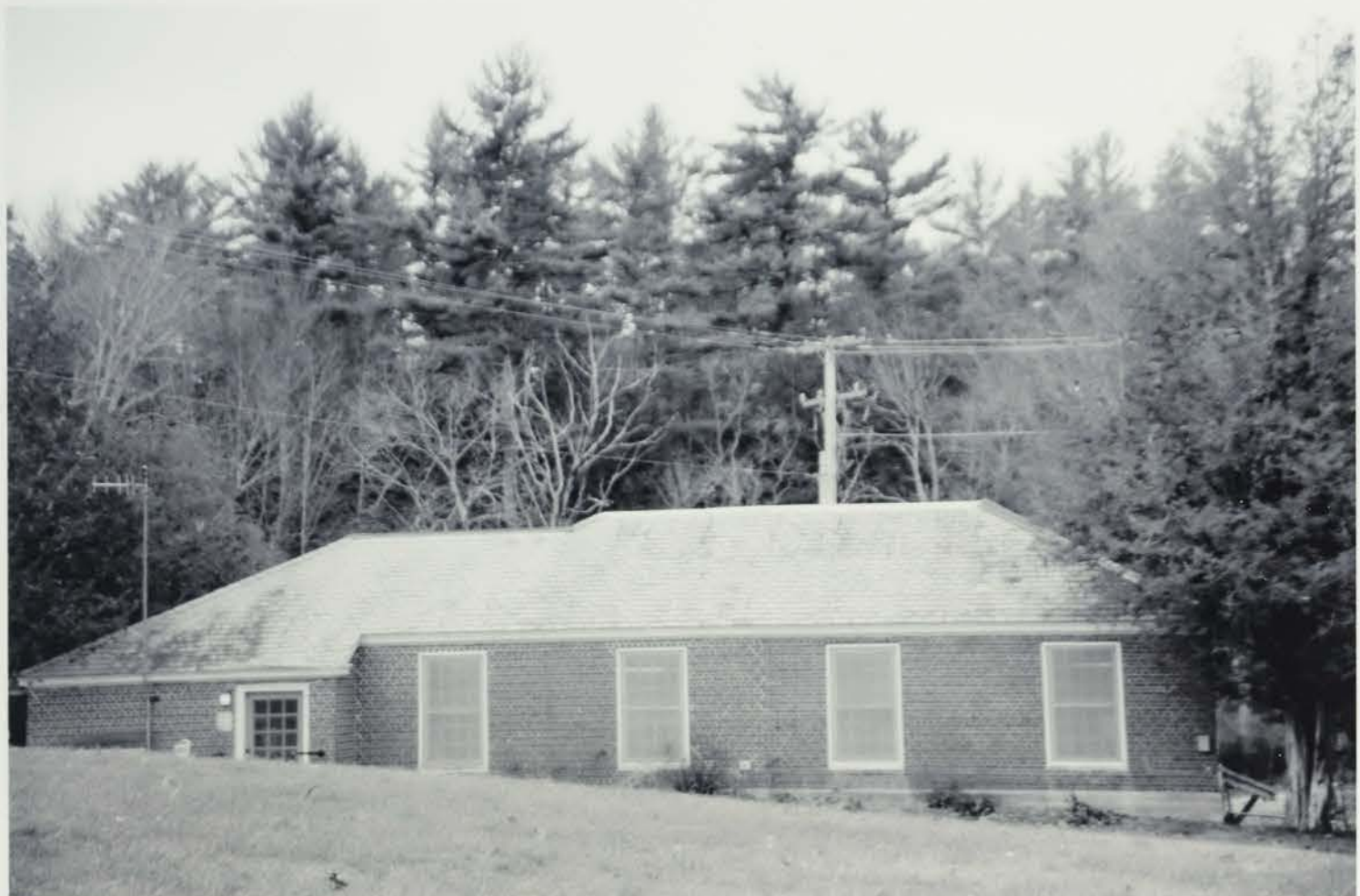
Photo 081) 42 Waterworks Road – Water Treatment Building photo taken December 2015
