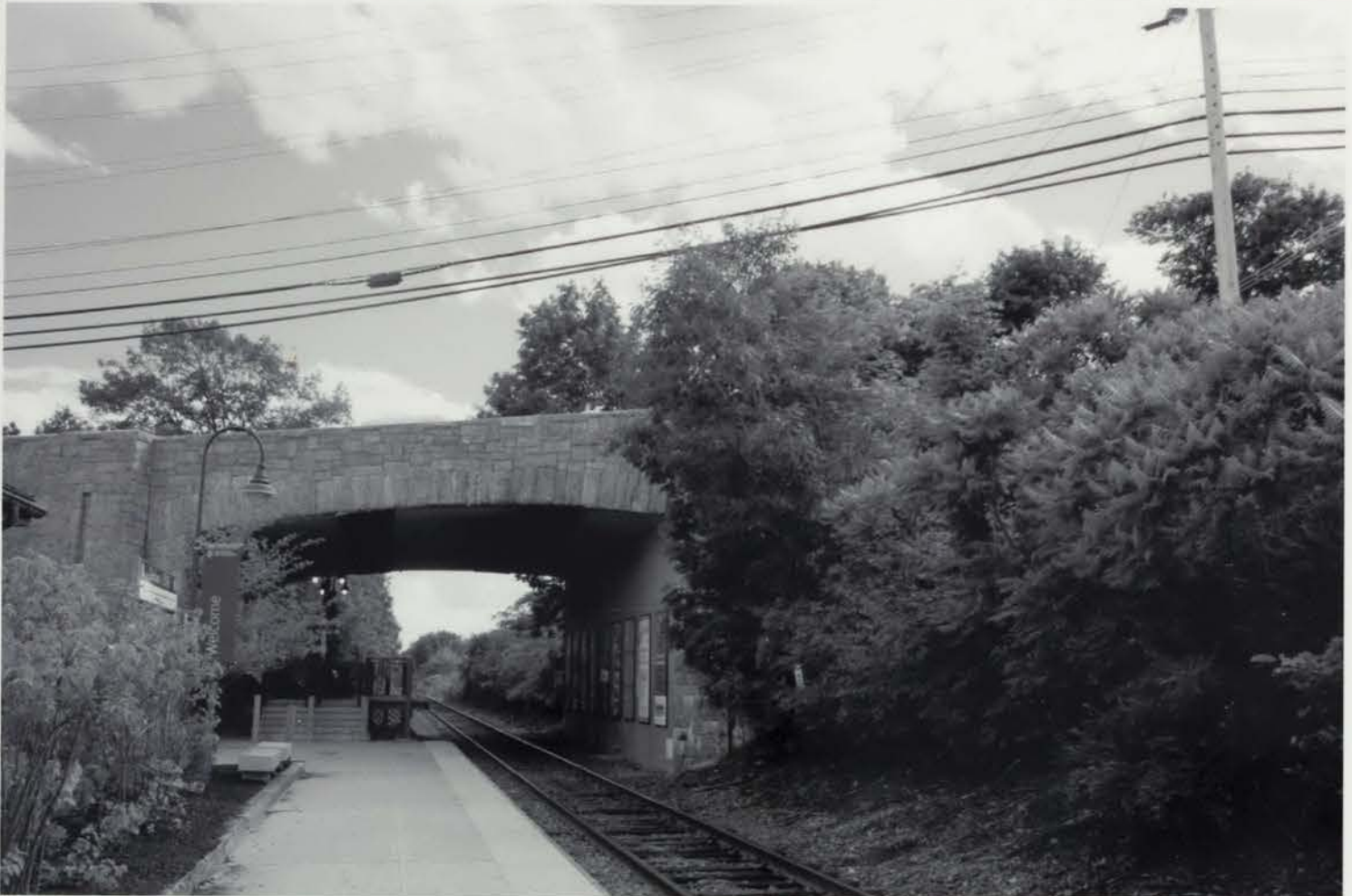
Photo 036) Main Street Bridge over Railroad, Boston and Maine Railroad Western Division Historic District photo taken June 2015 Direction: S
