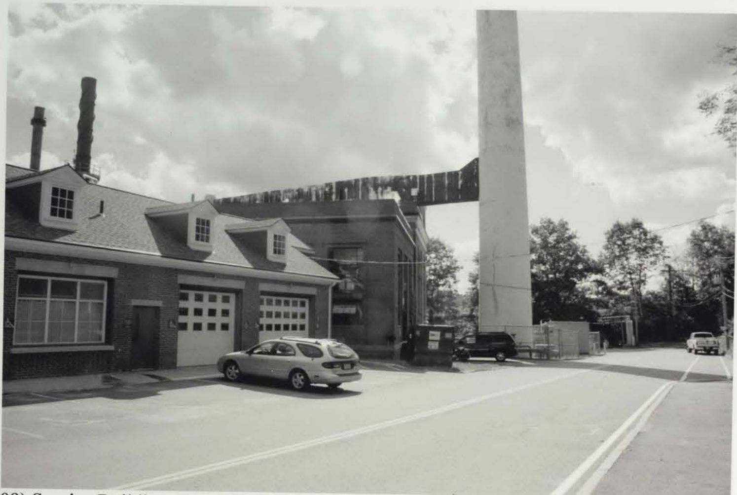
Photo 009) Service Building (51 College Road) and Heating Plant (2 Library Way) photo taken June 2015
