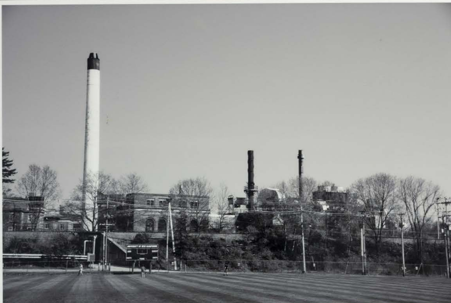
Photo 050) View from field to south of Stadium toward central campus and power plant on other side of railroad photo taken May 2016 Direction: SE
