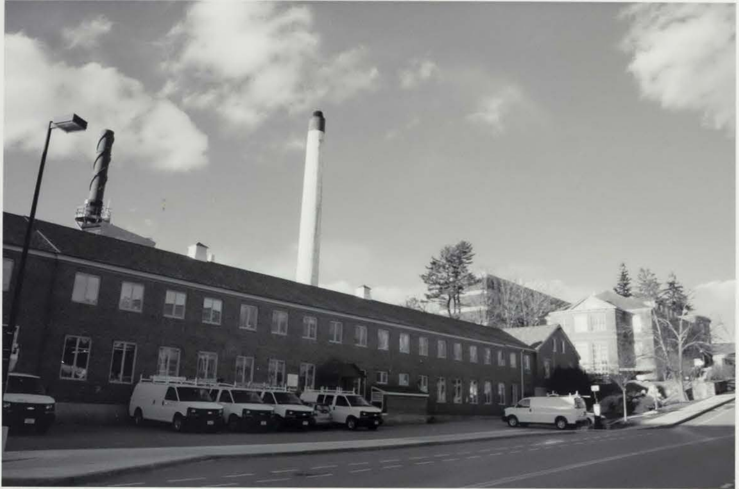
Photo 018) 51 College Road – Service Building photo taken January 2016
