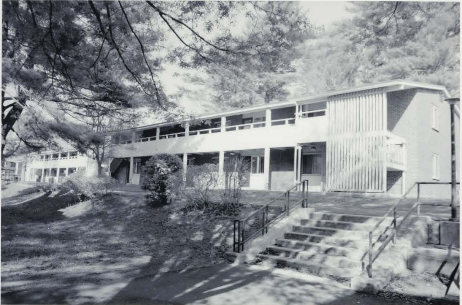
Photo 063) 4 Demeritt Circle – Forest Park Apartments photo taken May 2016
