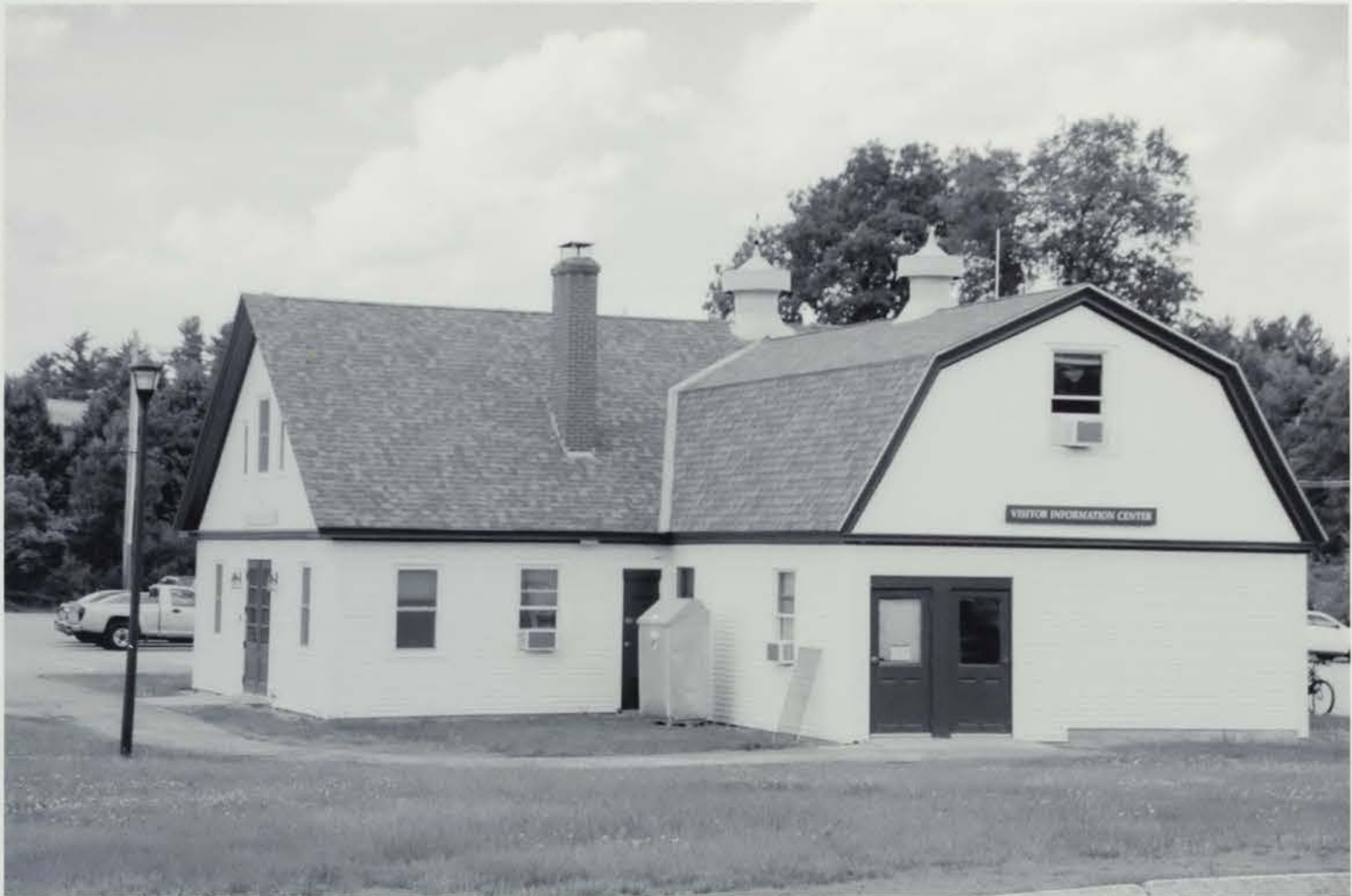
Photo 089) UNH Transit and Visitor Center, former stable, 20 Sage Way photo taken June 2015
