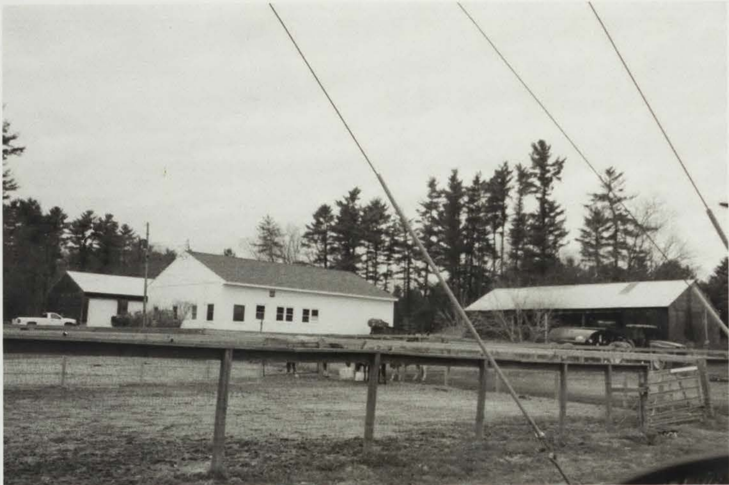
Photo 93) Farm Services Buildings, 287 Mast Road photo taken December 2015
