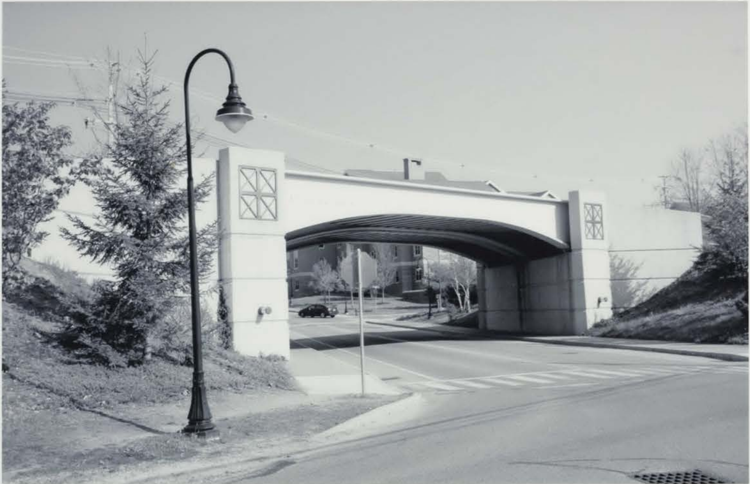
Photo 072) Looking from Waterworks Road toward bridge under railroad to South Drive Direction: SSE photo taken May 2016
