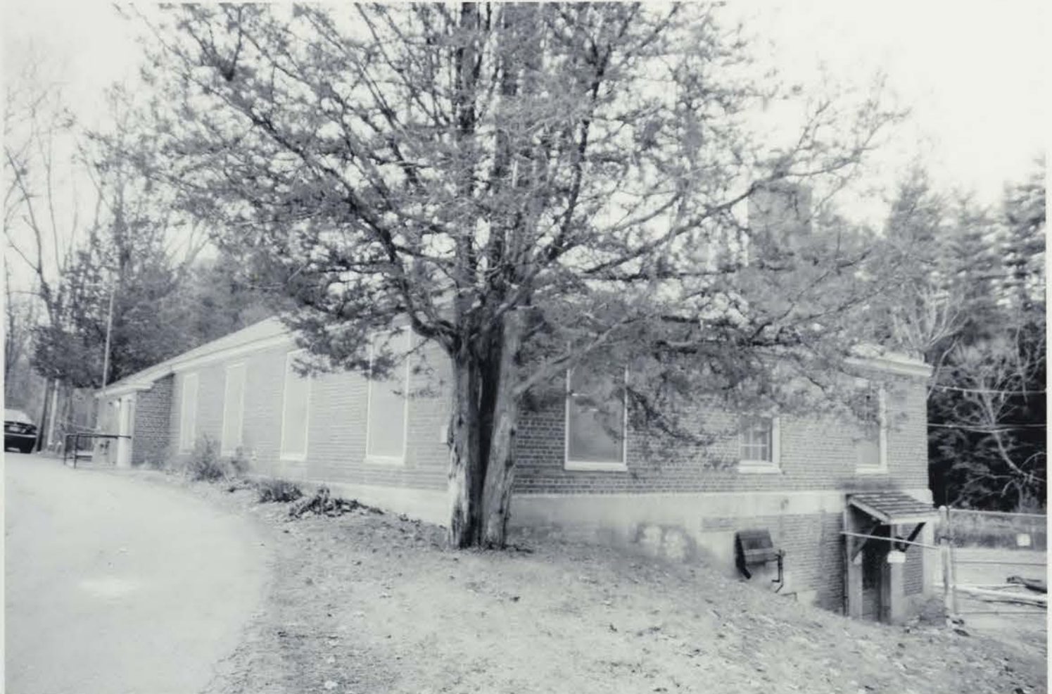
Photo 080) 42 Waterworks Road – Water Treatment Building photo taken December 2015
