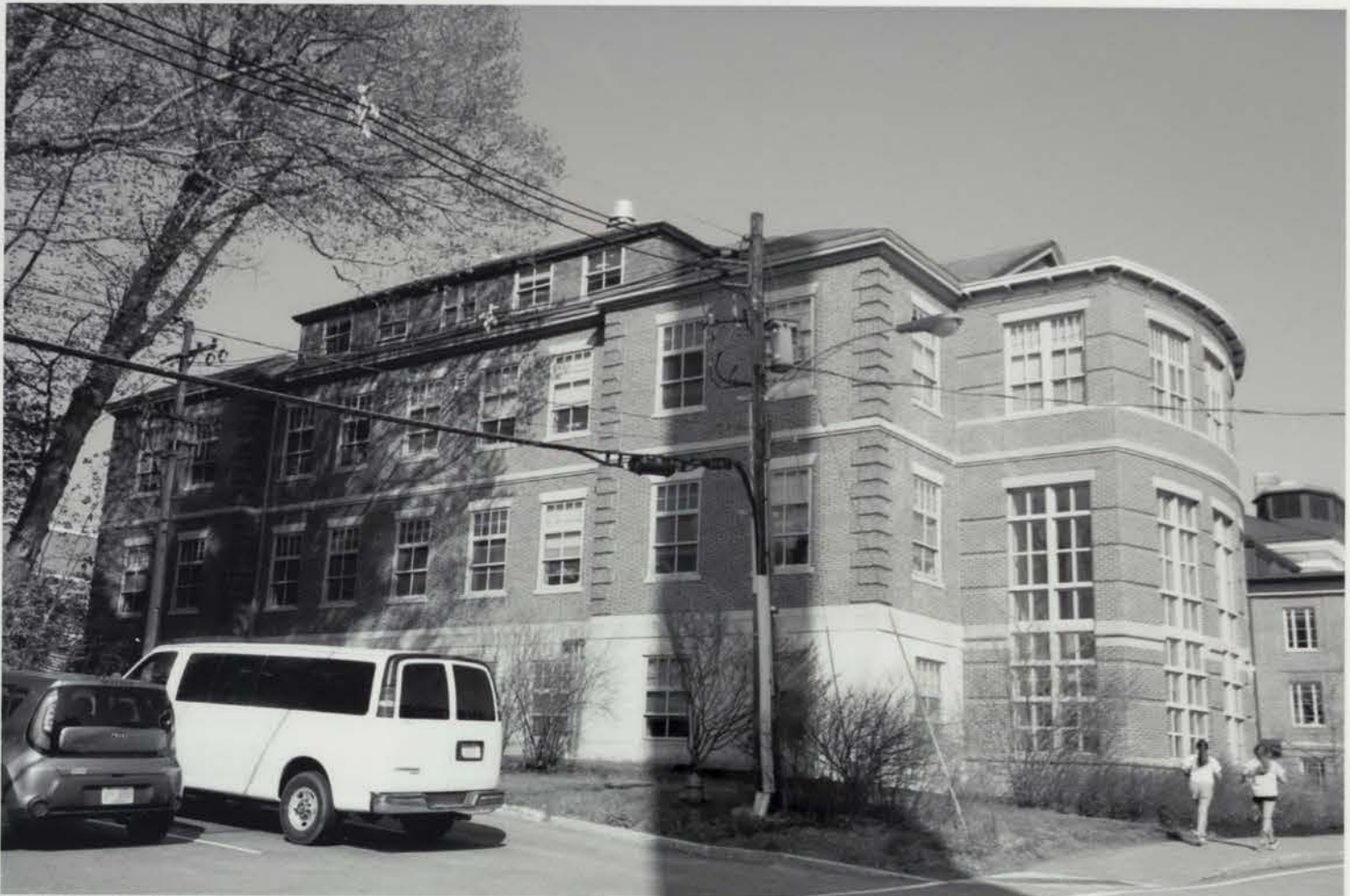
Photo 016) 55 College Road – Pettee Hall photo taken May 2016
