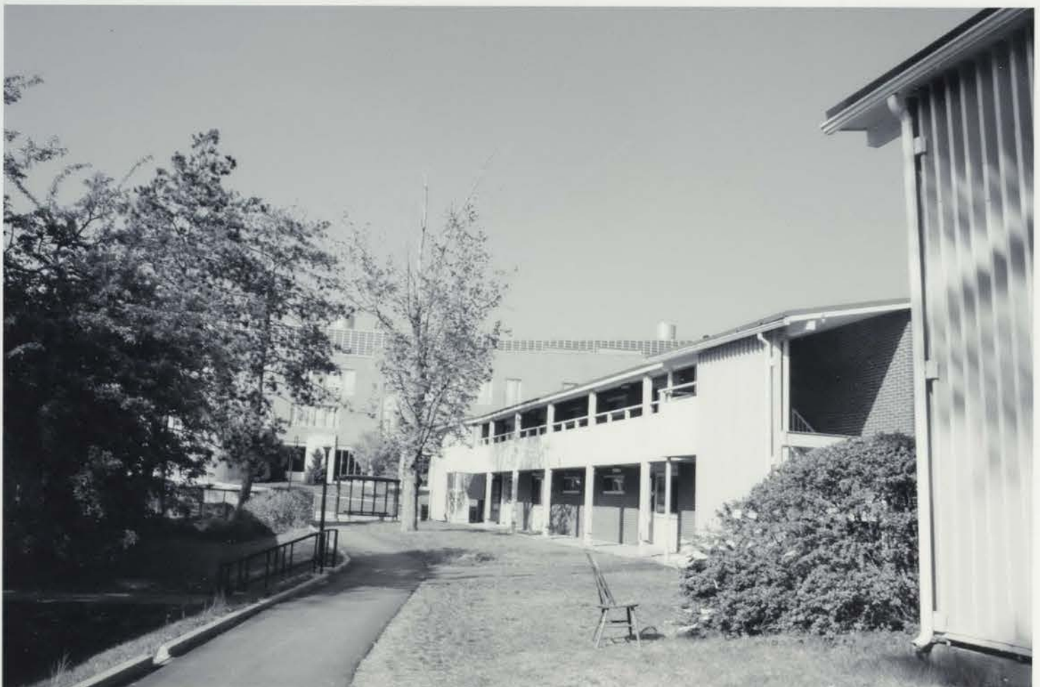
Photo 064) 4 Demeritt Circle – Forest Park Apartments photo taken May 2016
