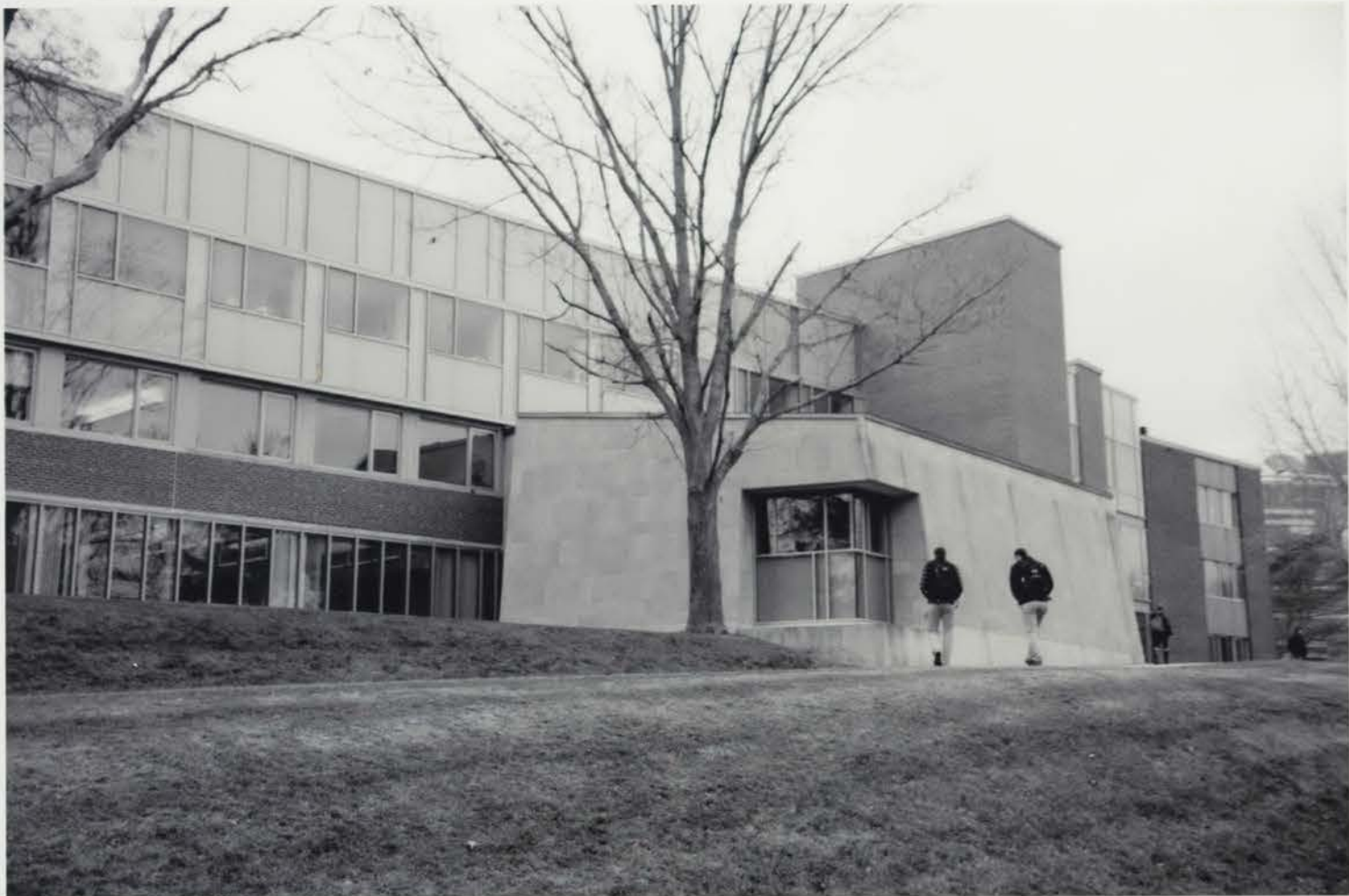
Photo 022) 33 Academic Way – Kingsbury Hall photo taken December 2015
