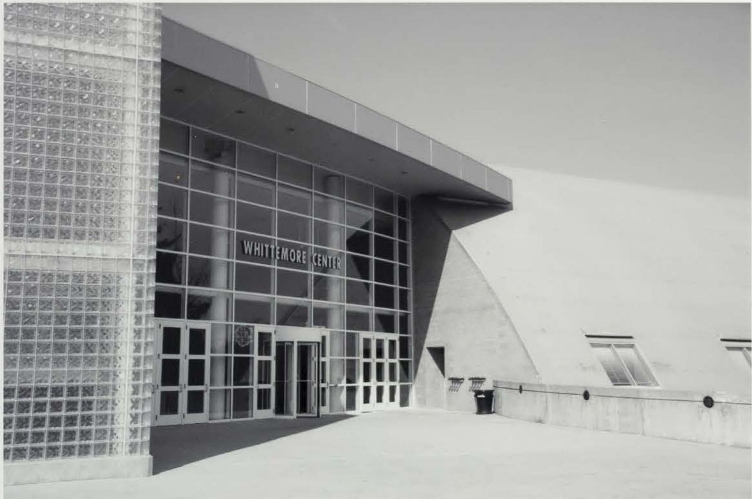
Photo 030) 128 Main Street – Whittemore Center photo taken May 2016
