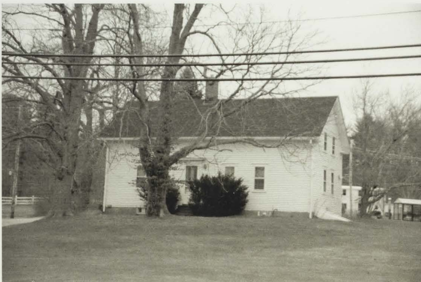
Photo 0100) 208 Main Street – John Woodman/Mathes House photo taken December 2015
