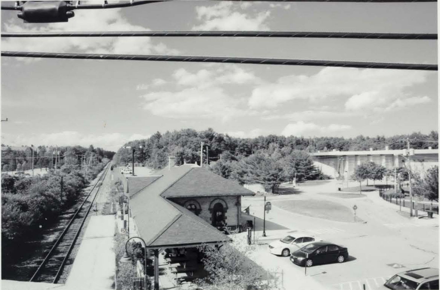
Photo 038) 3 Depot Road – Durham UNH Railroad Station, from Main Street Bridge Direction: NNE photo taken June 2015
