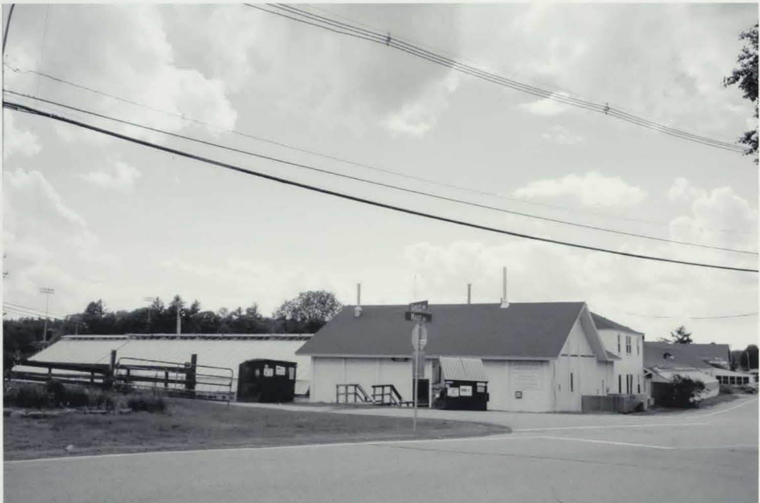
Photo 086) Macfarland Greenhouses, 13 Botanical Lane photo taken June 2015
