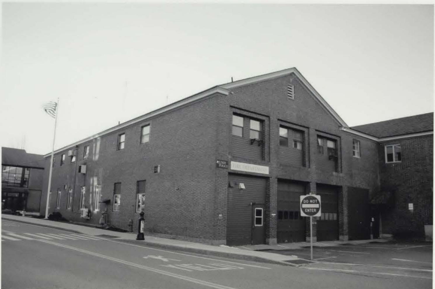
Photo 017) 51 College Road – Service Building photo taken January 2016
