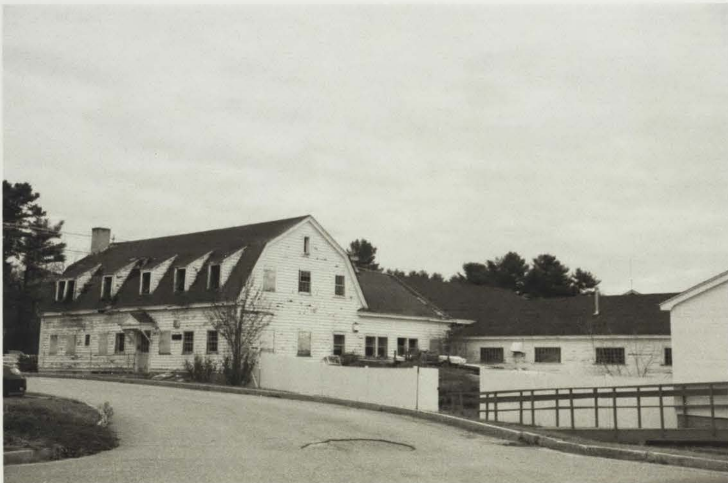
Photo 098) Old Dairy Barn, 278 Mast Road photo taken December 2015
