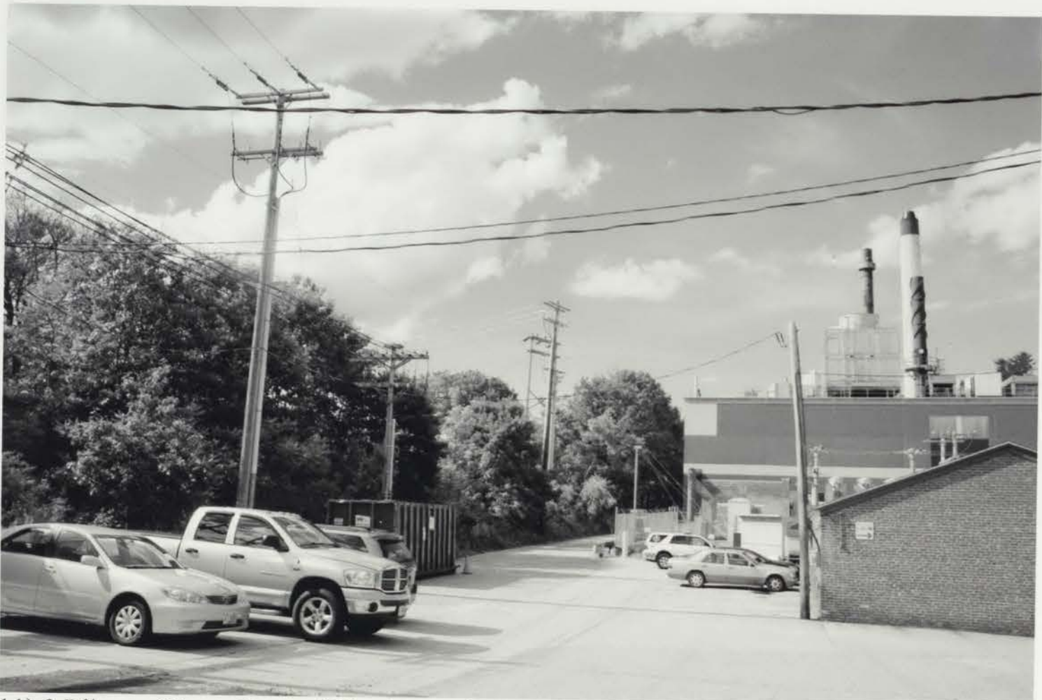
Photo 011) 2 Library Way – Rear of Heating and Power Plant rear, railroad tracks at left Direction: N photo taken June 2015
