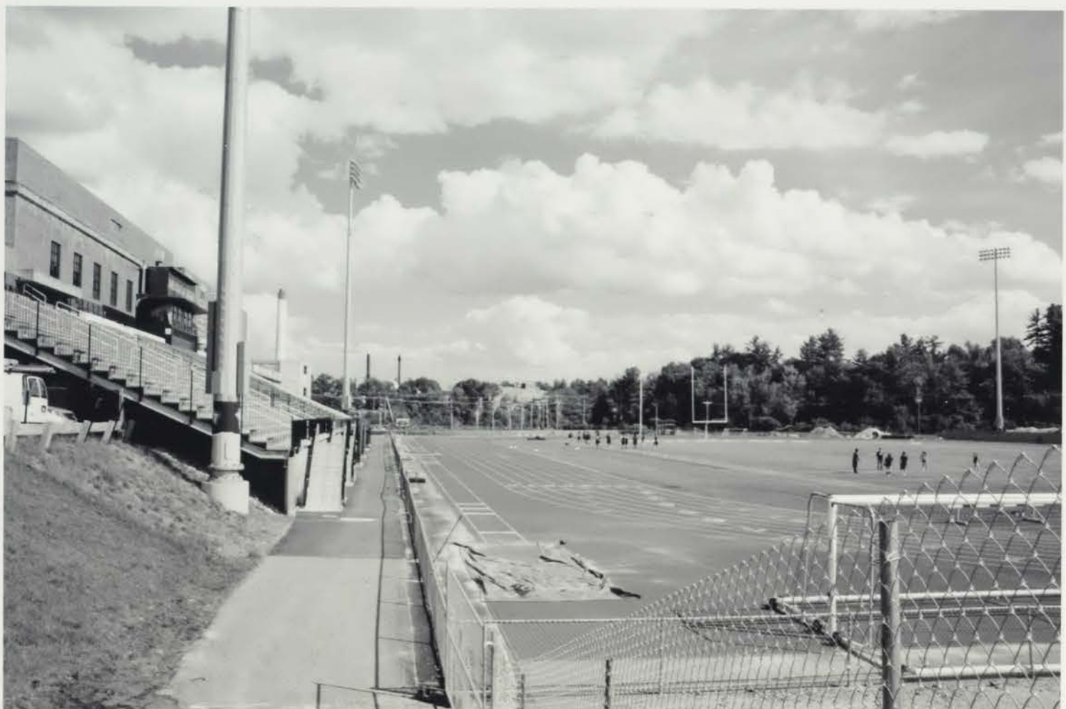
Photo 045) Stadium and football field Direction: SE photo taken June 2015 7
