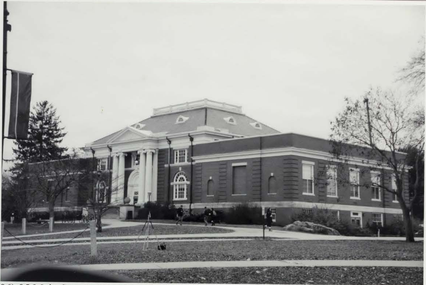
Photo 006) 95 Main Street – Hamilton Smith Hall photo taken December 2015
