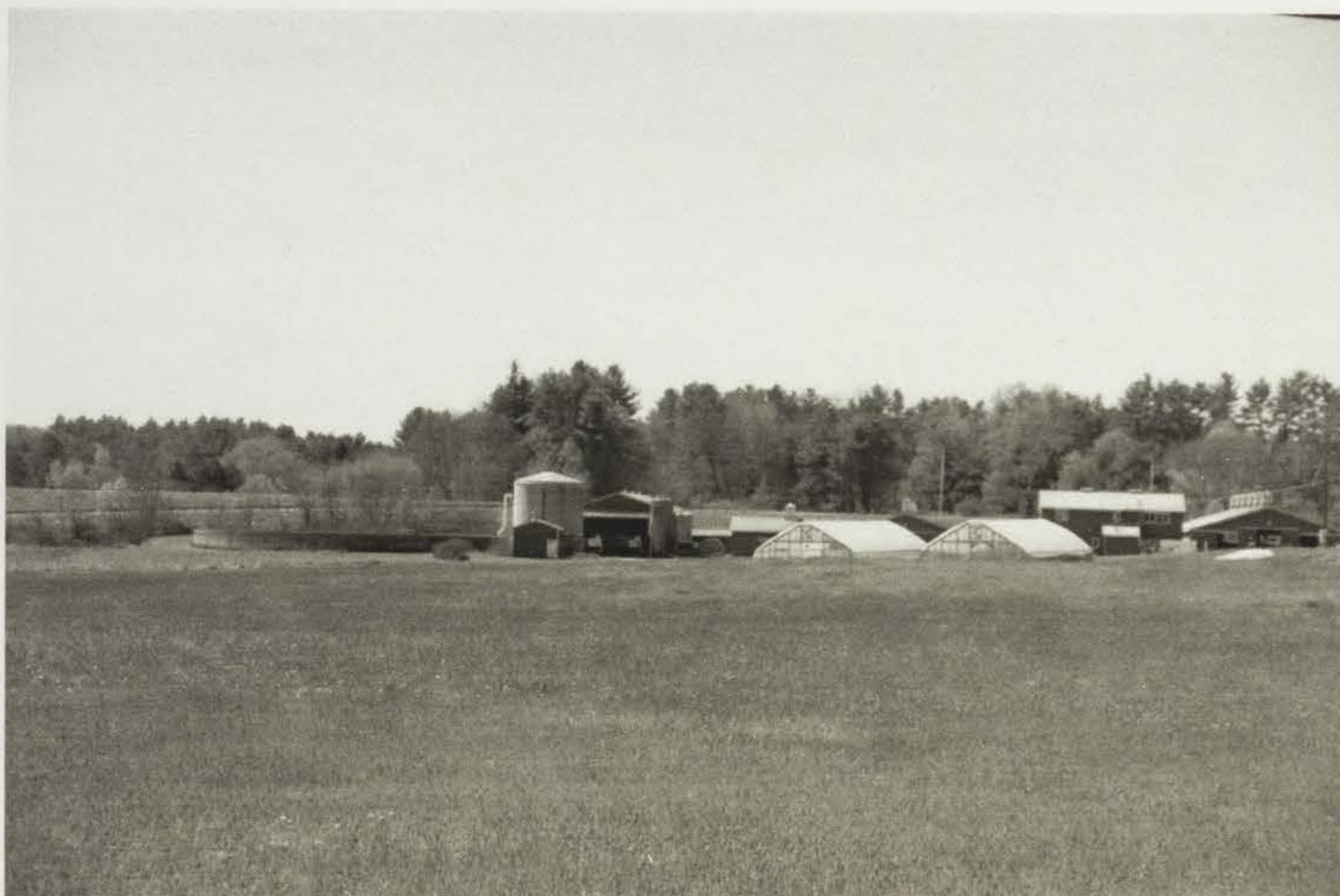
Photo 0104) Dairy Research Center and farm buildings, 36 O'Kane Road photo taken May 2016
