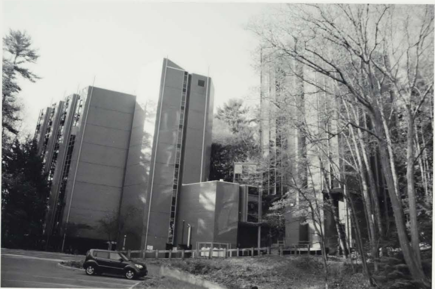
Photo 029) 21 Strafford Avenue – Adams Tower photo taken May 2016
