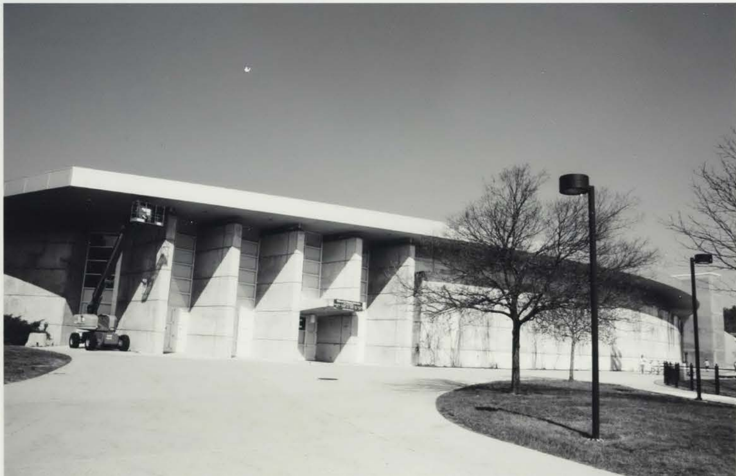
Photo 031) 128 Main Street – Whittemore Center photo taken May 2016
