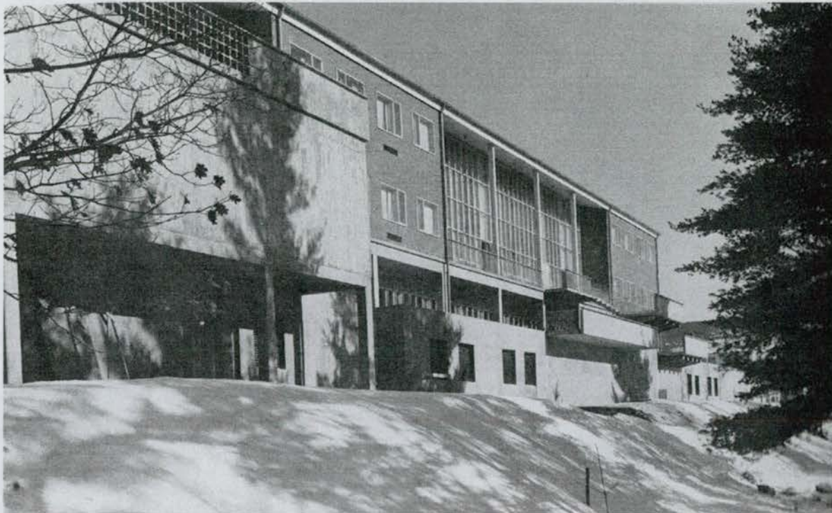
Memorial Union Building ca. 1960s (Sackett 1974, 150)
