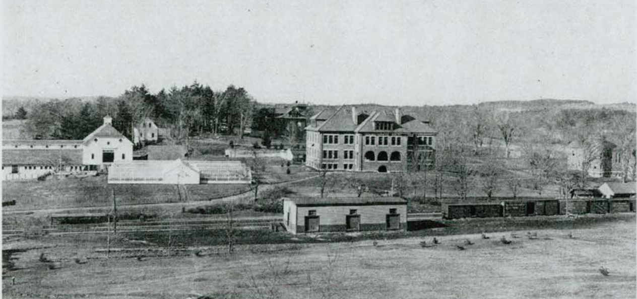
Campus view facing northwest, showing original railroad tracks, Morrill Hall, dairy barn and old greenhouses (not extant), ca. 1906 (Sackett 1974, 52)
