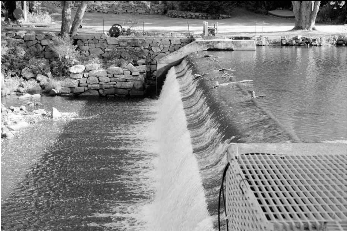
Photo 4: Spillway detail from north abutment/fish ladder
