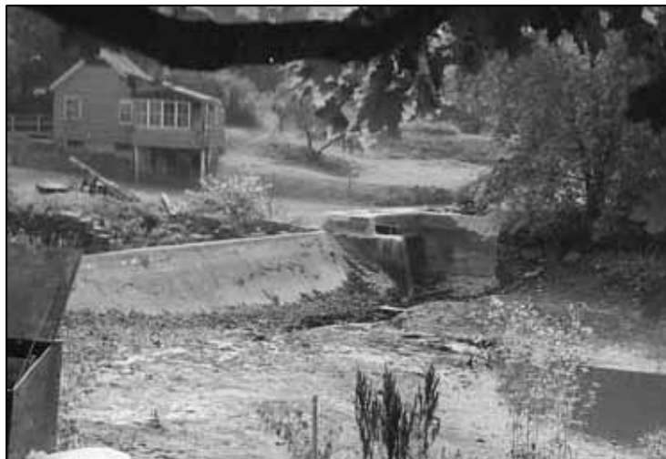
1974 before repairs, facing SE, showing former Jenkins cottage, site 20 Newmarket Road
