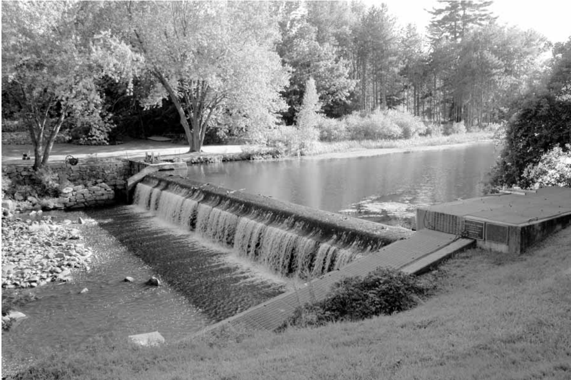
Photo 2: View from north end (parcel 5/3-3), showing top of fish ladder, looking toward mill site (6-9-1) Direction: SW
