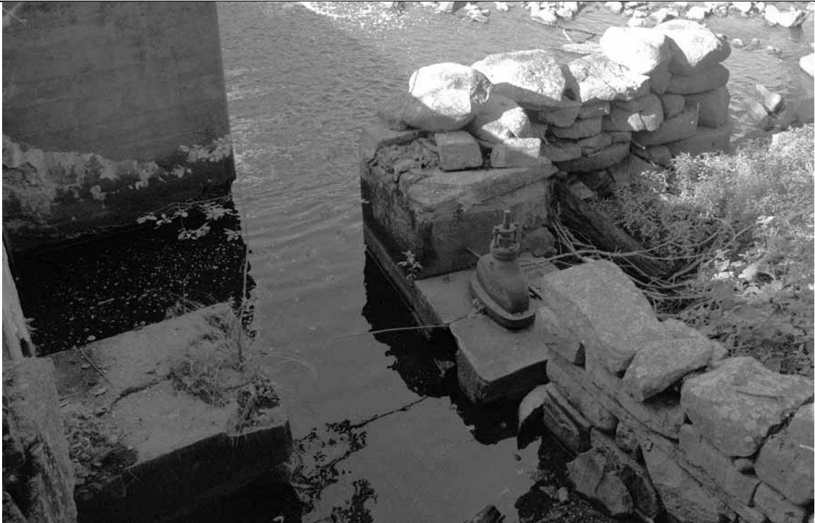
Photo 16: former penstock location
