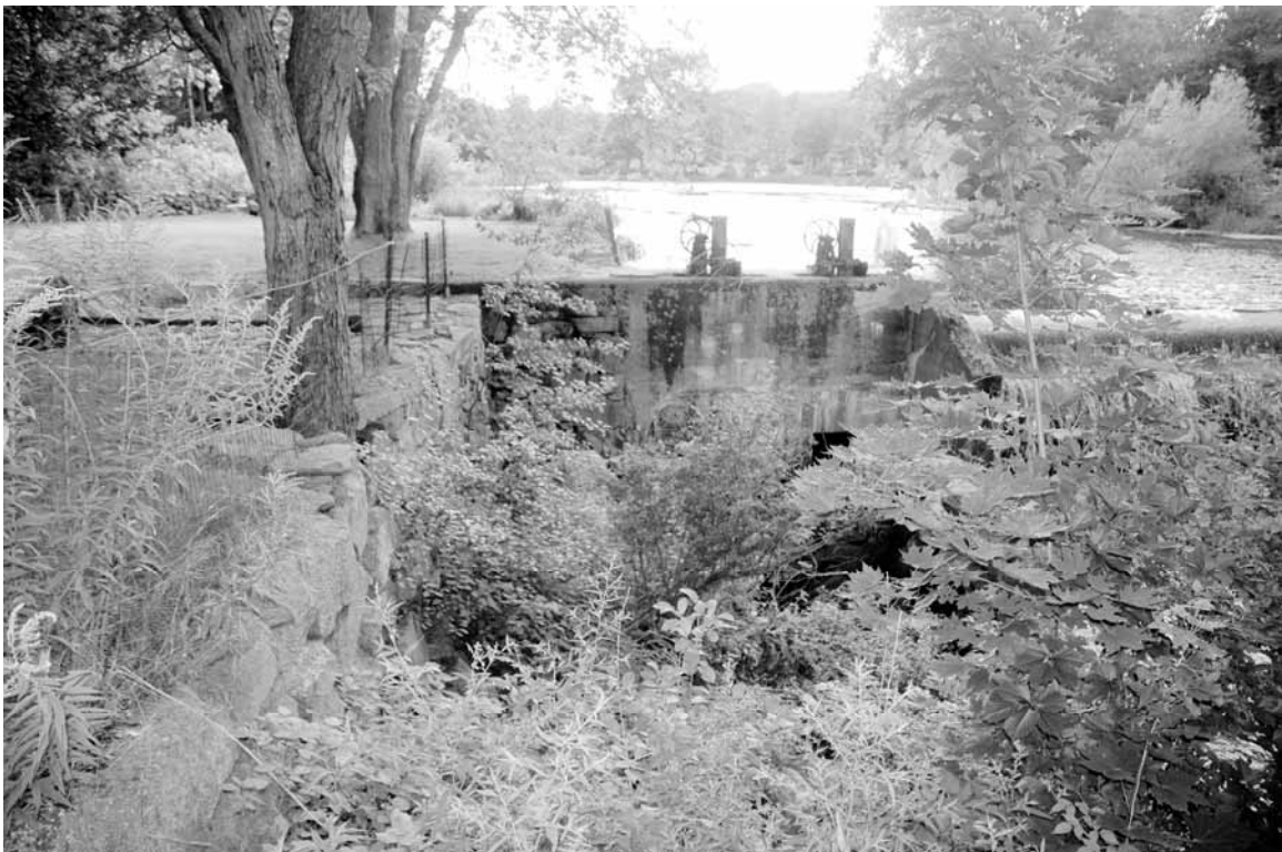
Photo 19: Mill foundation, looking toward gates
