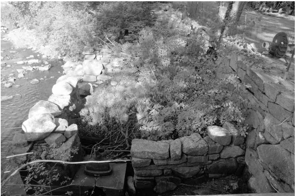
Photo 17: Mill foundation and riverbank, downstream from gates
