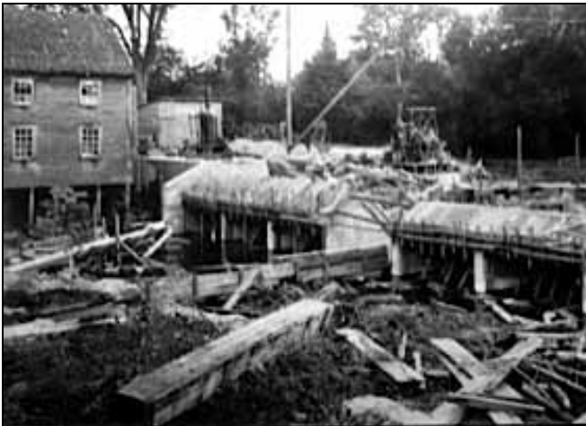
South abutment and spillway construction photographs 1913 (Durham Historic Association)
