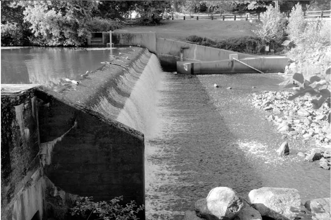
Photo 8: From south abutment, facing north
