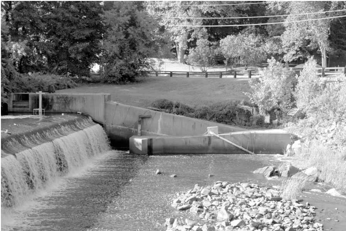
Photo 7: Fish ladder from south end of dam, looking toward map/parcel 5/3-3
