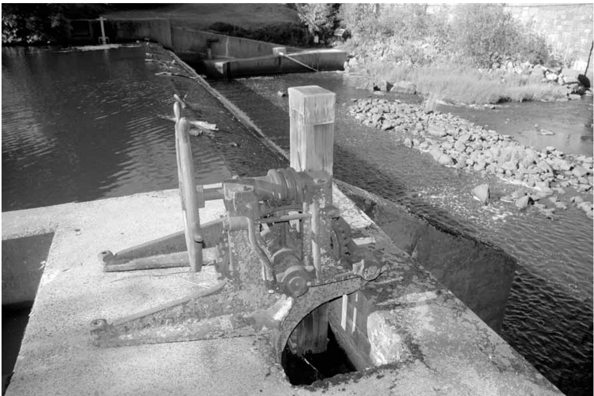
Photo 13: gate mechanism
