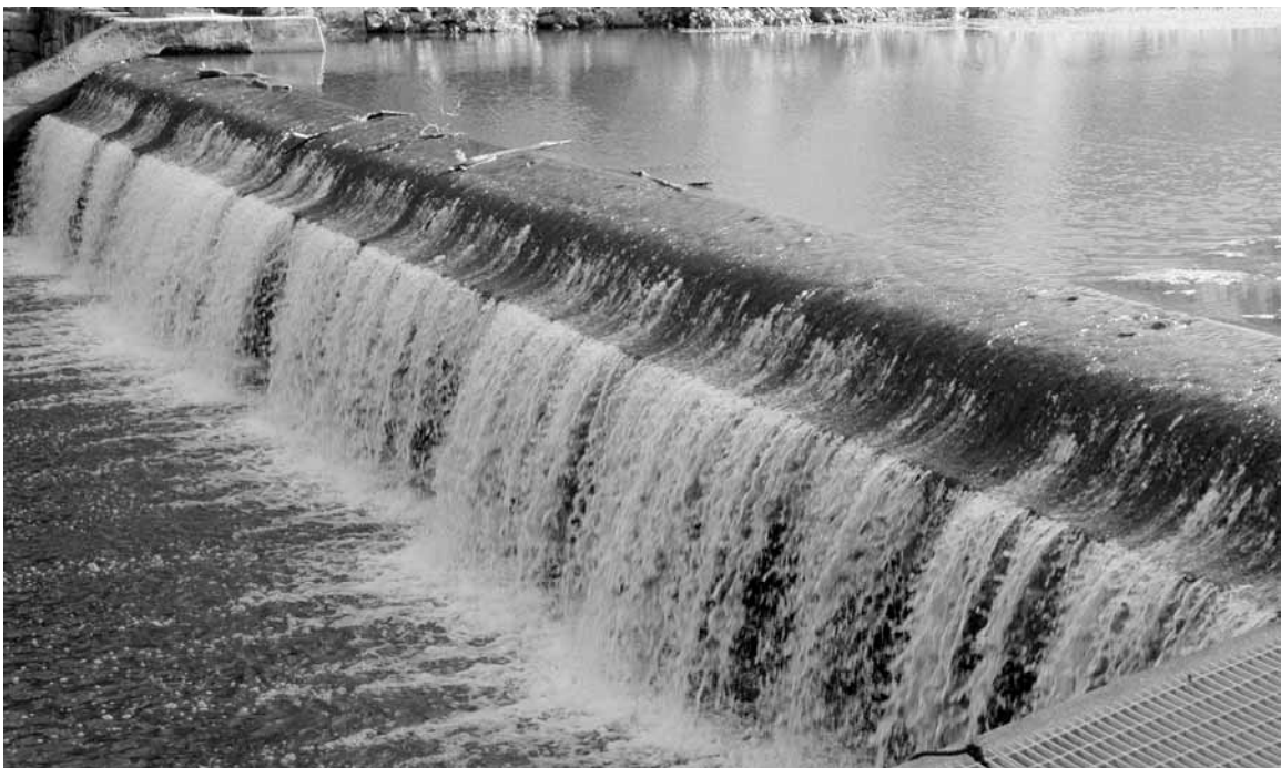
Photo 3: spillway from fish ladder Direction: SW
