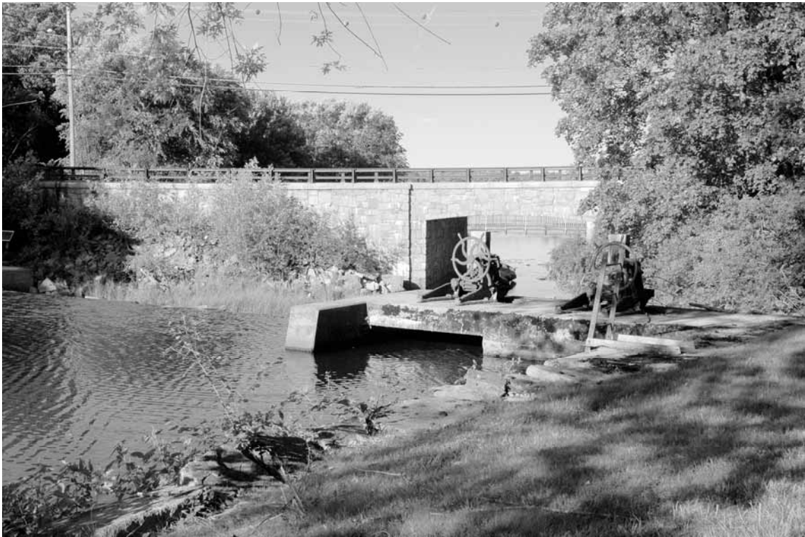
Photo 11: Gates, top of dam looking downstream toward NH 108 Bridge
