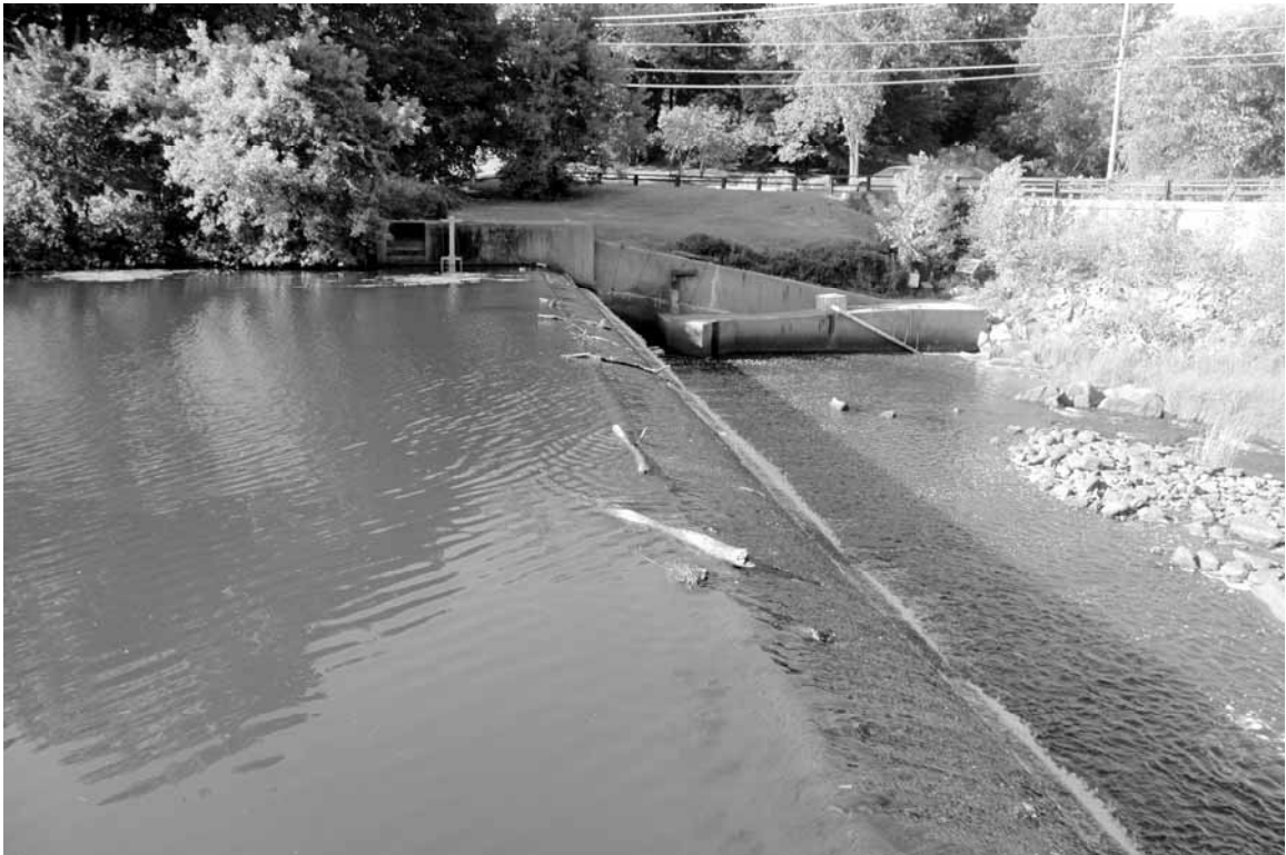
Photo 9: Top of spillway
