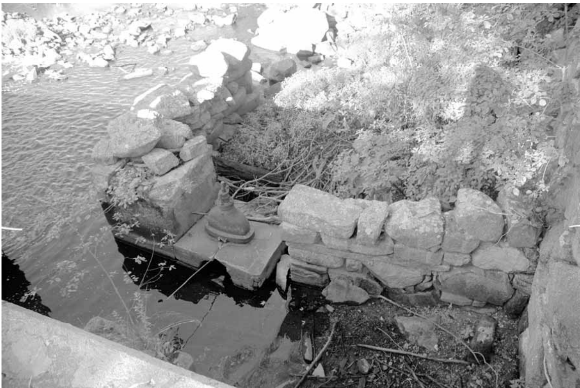
Photo 15: Mill foundation, from top of gates, showing former penstock location
