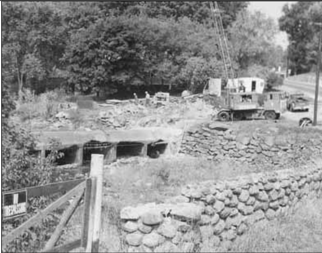
1974 construction, facing NNW toward 14 Newmarket Road (Durham Historic Association)
