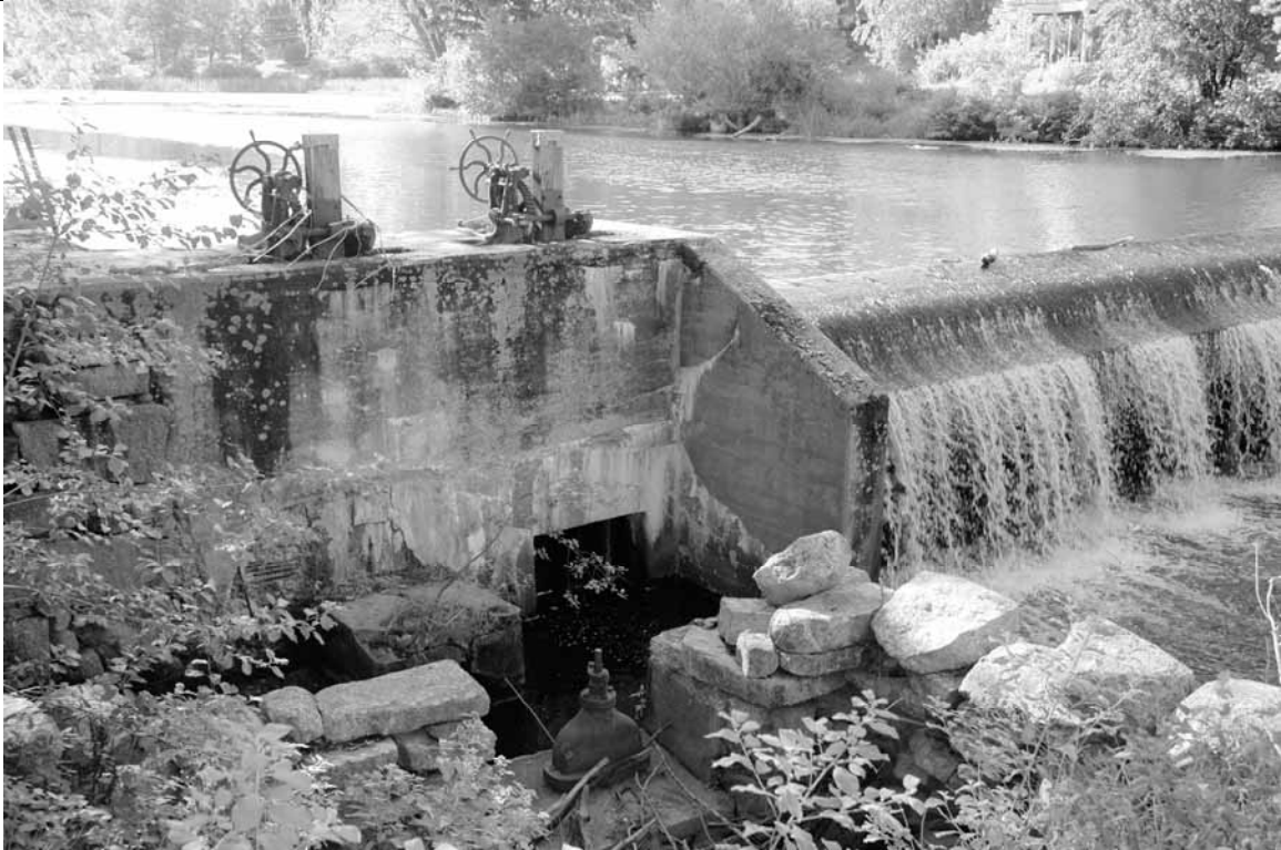
Photo 10: South abutment and gates
