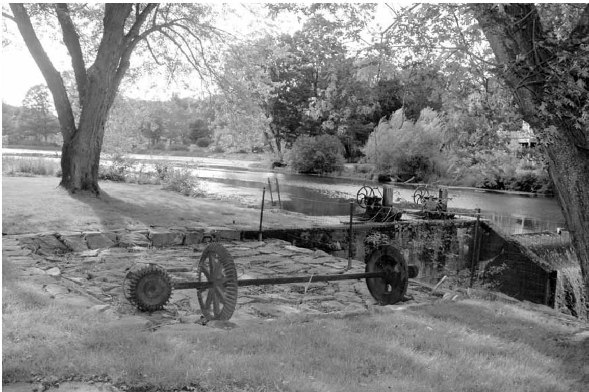
Photo 21: stone patio drain, downstream from south abutment, former mill foundation Direction: NW
