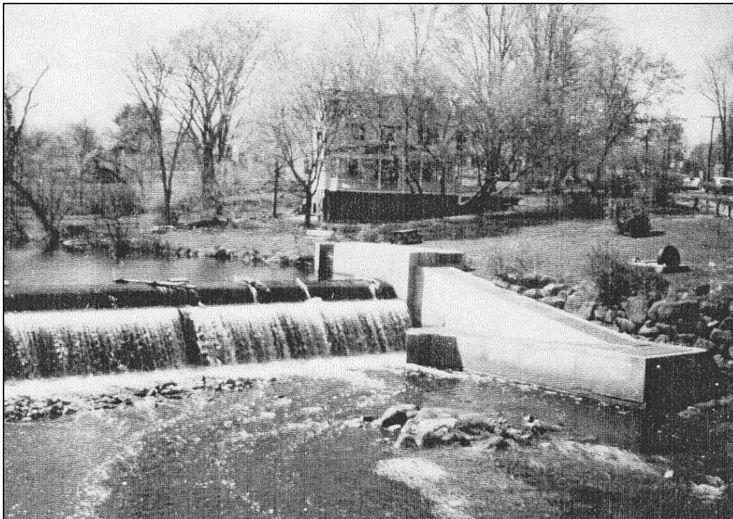
1978 showing newly built fish ladder (NHDES).
