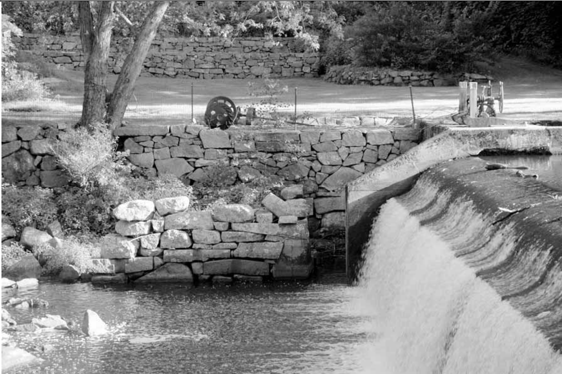
Photo 14: mill foundation, stone walls of 20 Newmarket Road lawn in background
