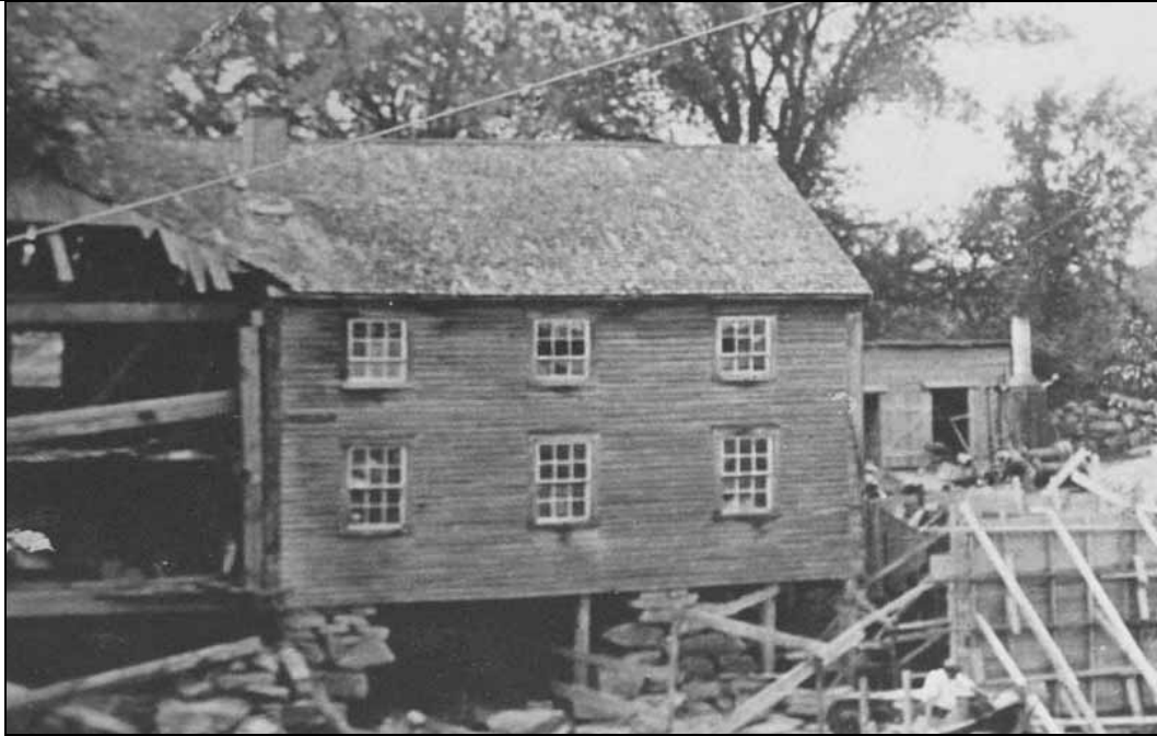
Jenkins Mill at time of concrete dam construction 1913 (Durham Historic Association)
