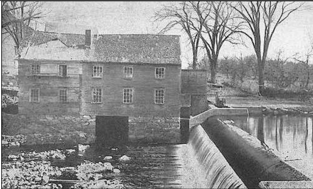
ca. 1920 postcard showing concrete dam, rebuilt mill foundation
