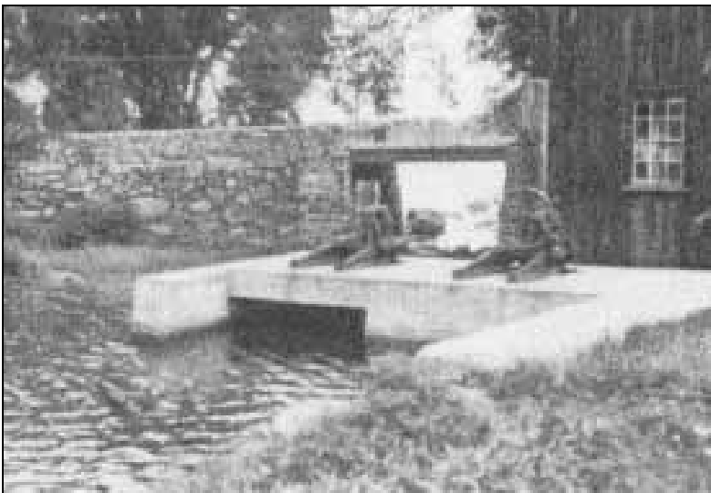
1935 Dam Inspection photos (NHDES)
