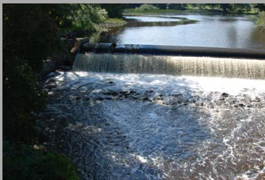
Oyster River Dam built 1913 (private photo-Andrea Bodo)
