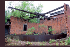
The 1859 Claremont Gasholder House ruins before demolition in 2015. The components of the rare pre-Civil War structure are expressed by the concentric pavement rings, vertical wood and steel posts, and overhead truss rods of the plaza around you.
