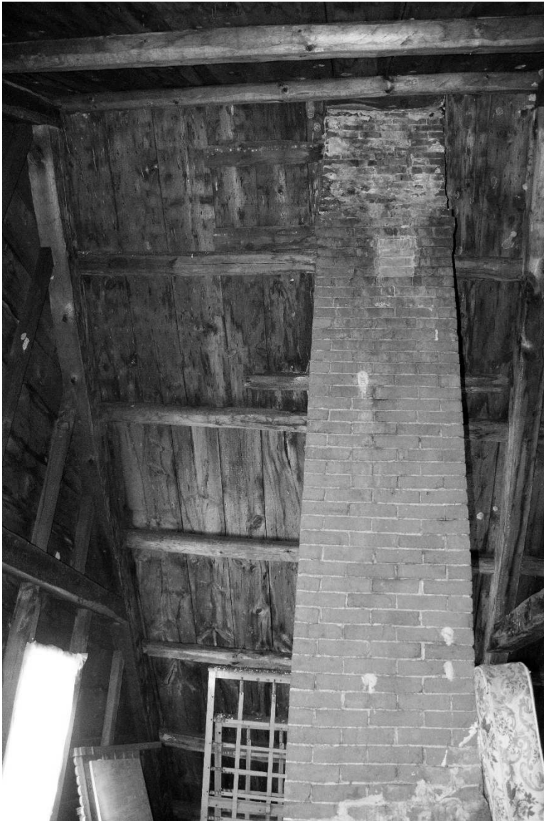
Photo 40) attic, western chimney shows original chimney cap Reference (file name): PIC_0606
