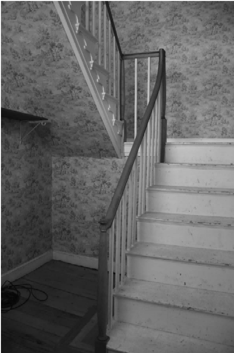
Photo 17) front staircase Reference (file name): PIC_1850
