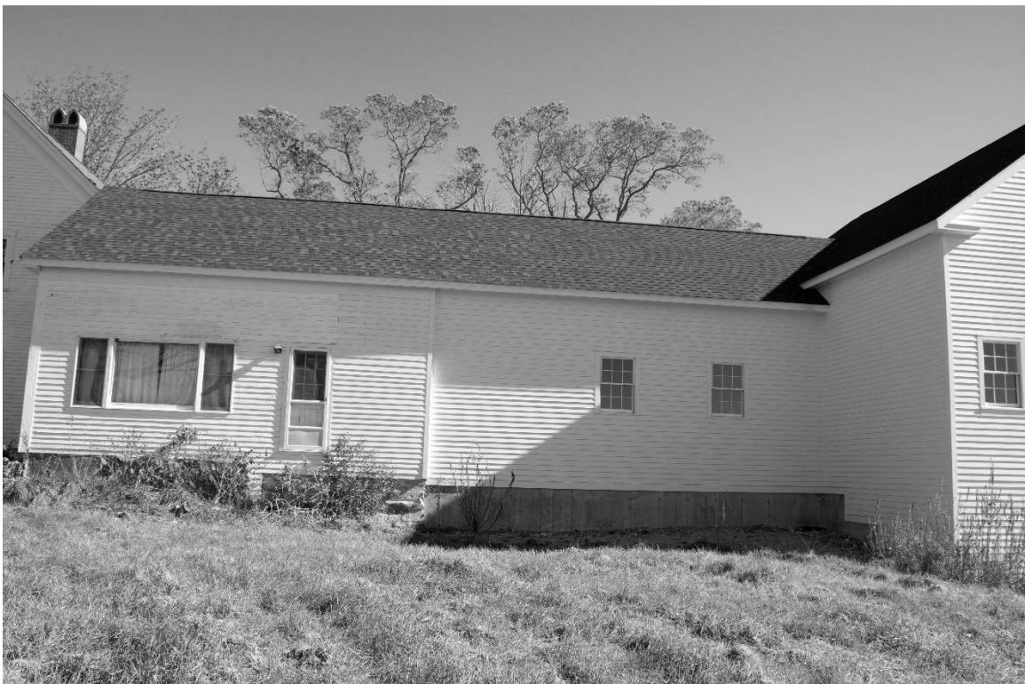
Photo 12) ell, west elevation shows original (left) and reconstructed ell Reference (file name): PIC_0518
