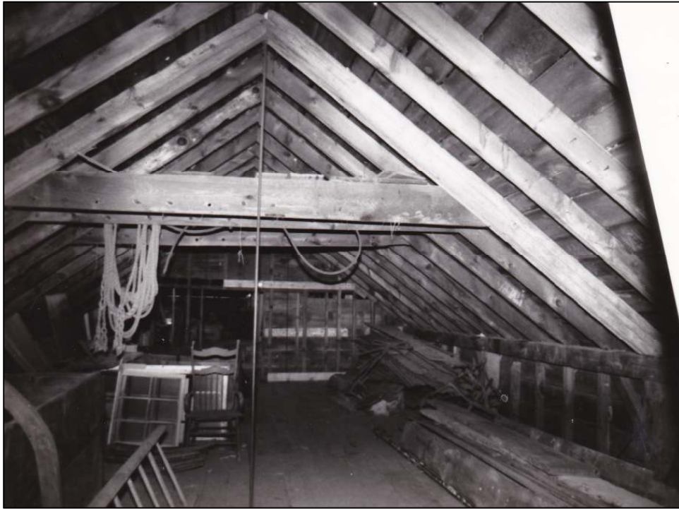
1990 interior of ell interior loft, partially rebuilt in 2017 (Federer 1991)
