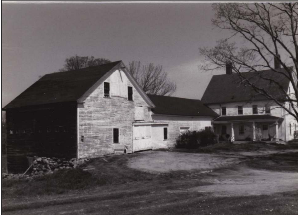
1990 rear elevation showing original stable and ell (Federer 1991)
