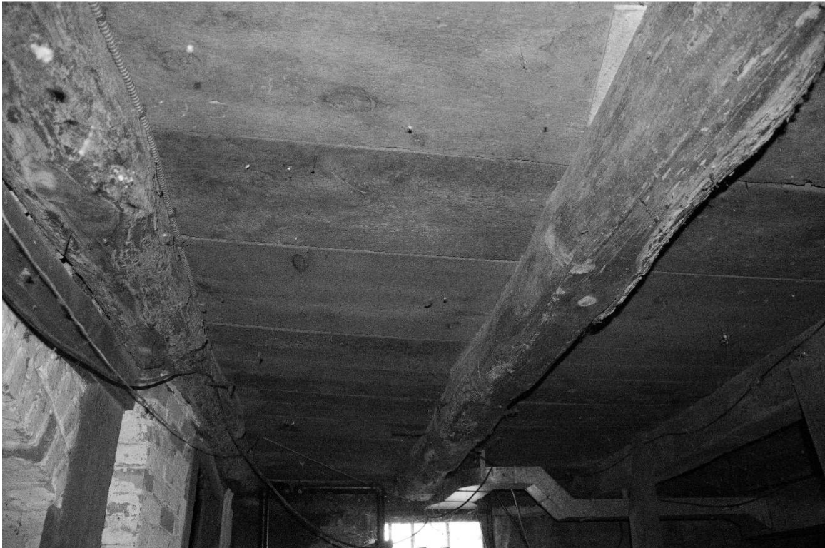
Photo 34) basement, floor framing detail Reference (file name): PIC_0604
