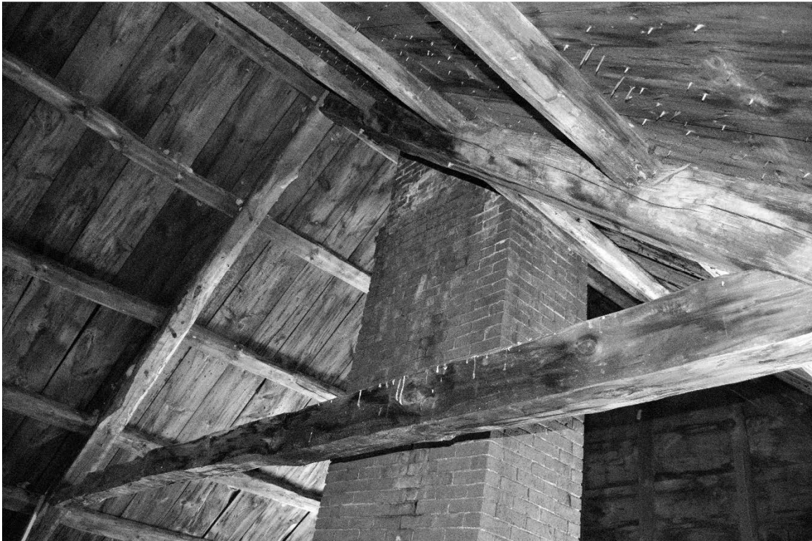
Photo 43) roof framing and chimney Reference (file name): PIC_0629
