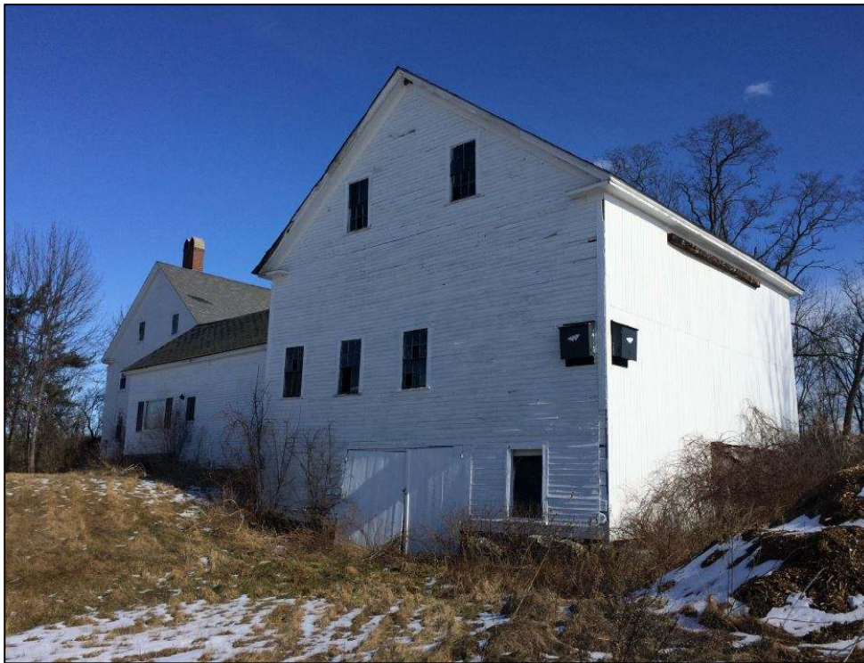
2017 stable rear elevation before reconstruction (Town of Durham)
