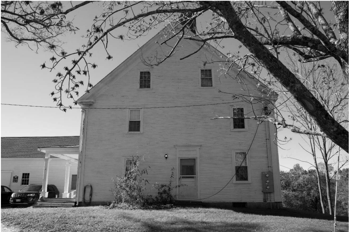
Photo 7) east elevation from driveway Reference (file name): PIC_0545
