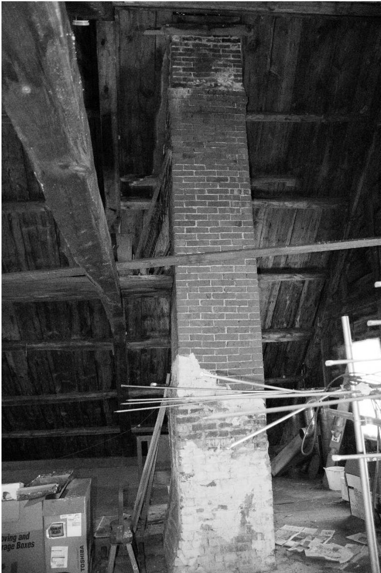
Photo 39) eastern chimney, showing original roofline, chimney cap and added stack above Direction: N Reference (file name): PIC_0623 Date taken: October 2018
