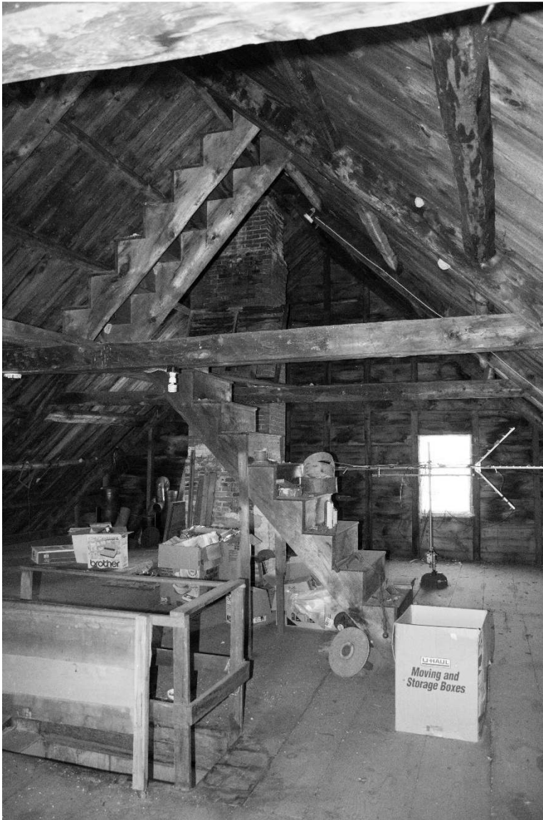
Photo 36) attic showing stairs to roof Reference (file name): PIC_0605
