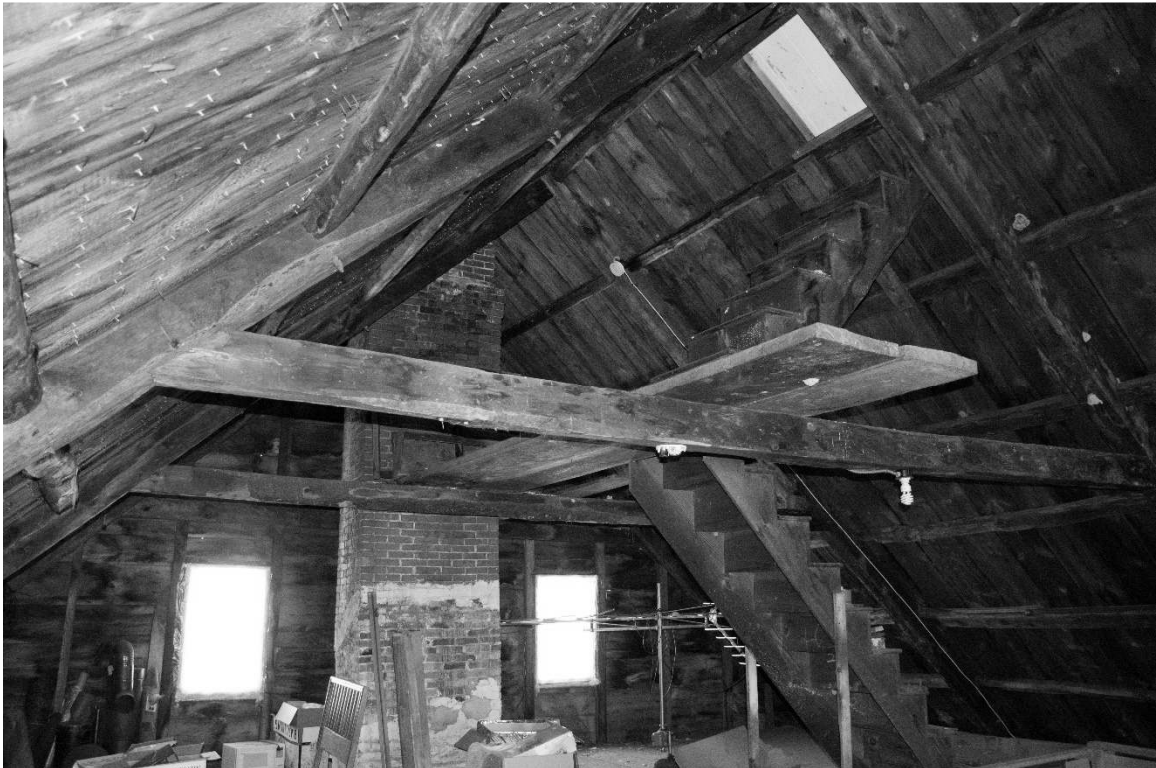
Photo 37) attic roof framing and stairs Reference (file name): PIC_0609
