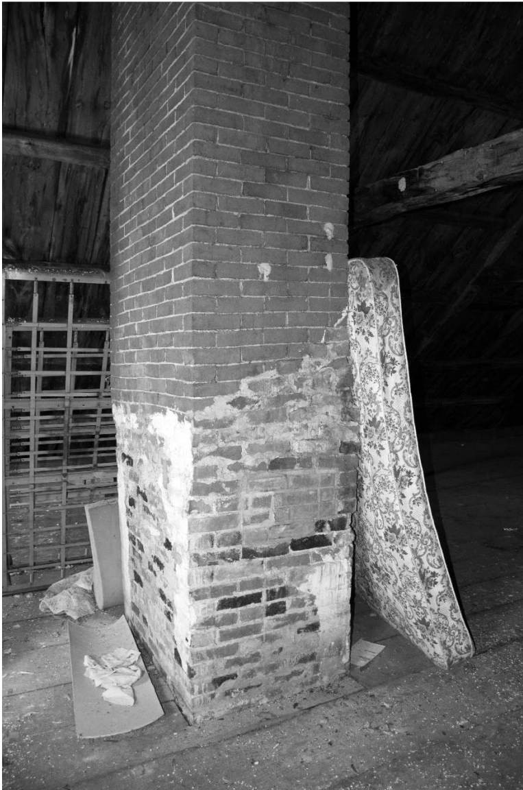
Photo 41) attic, western chimney shows original roofline Reference (file name): PIC_0619
