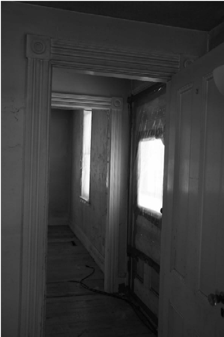
Photo 24) east side entry, Greek Revival trim Reference (file name): PIC_1848
