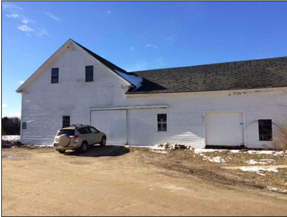
2017 stable and ell before reconstruction (Town of Durham)
