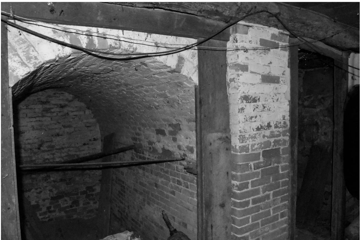
Photo 29) chimney arch, east chimney Reference (file name): PIC_1884
