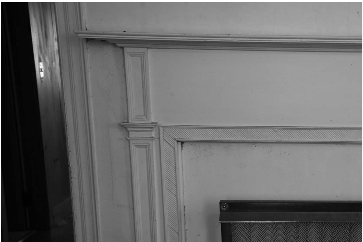
Photo 21) northwest front room, fireplace detail Reference (file name): PIC_1855
