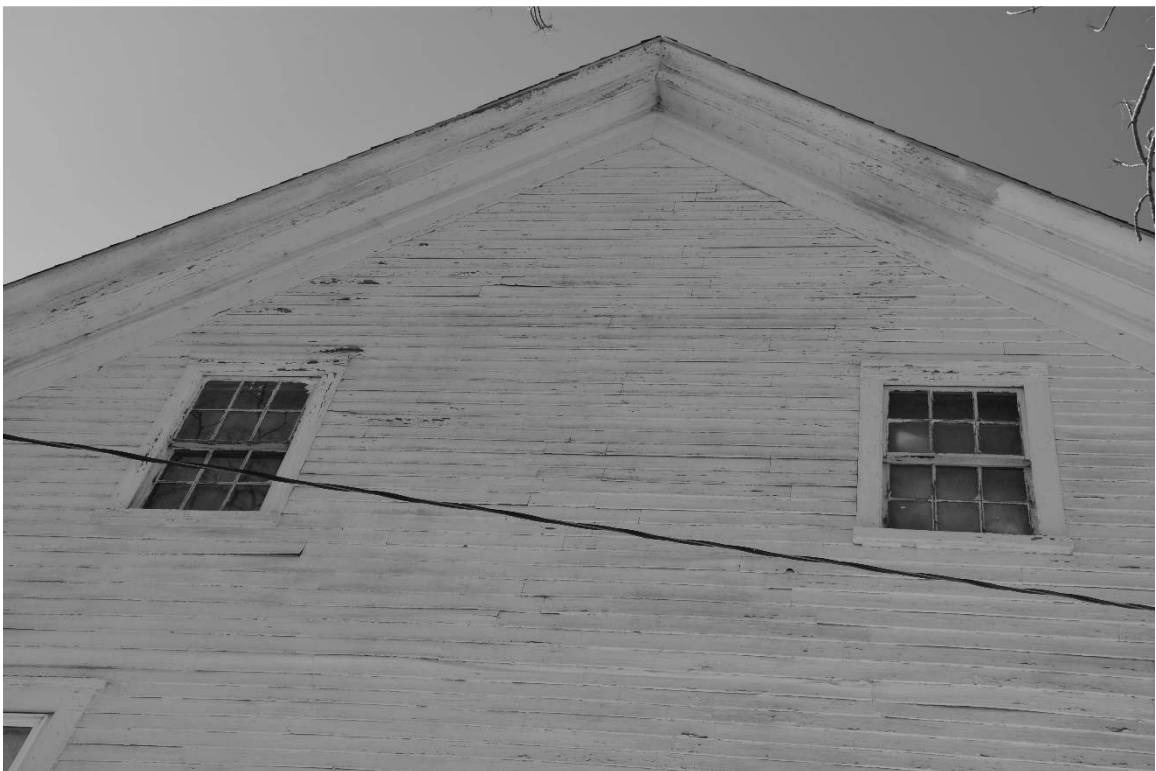
Photo 8) east elevation, attic windows and cornice detail Reference (file name): PIC_1893
