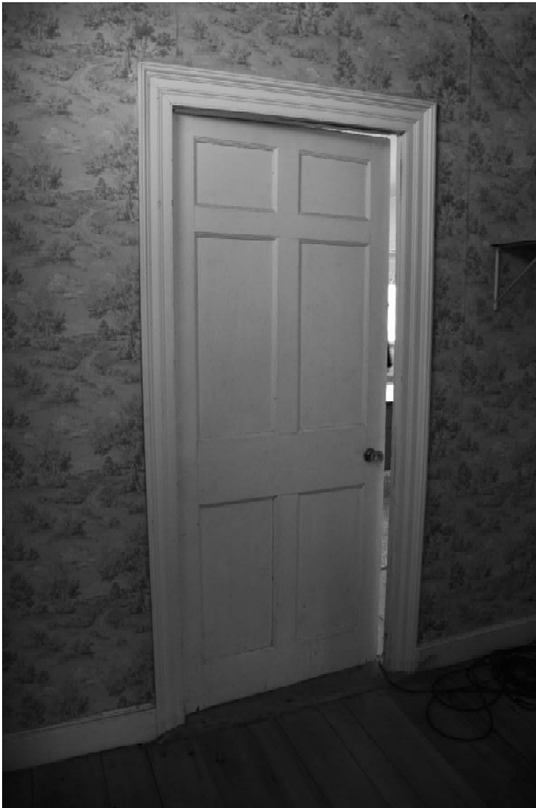
Photo 19) door, hallway to northwest front room Reference (file name): PIC_1851
