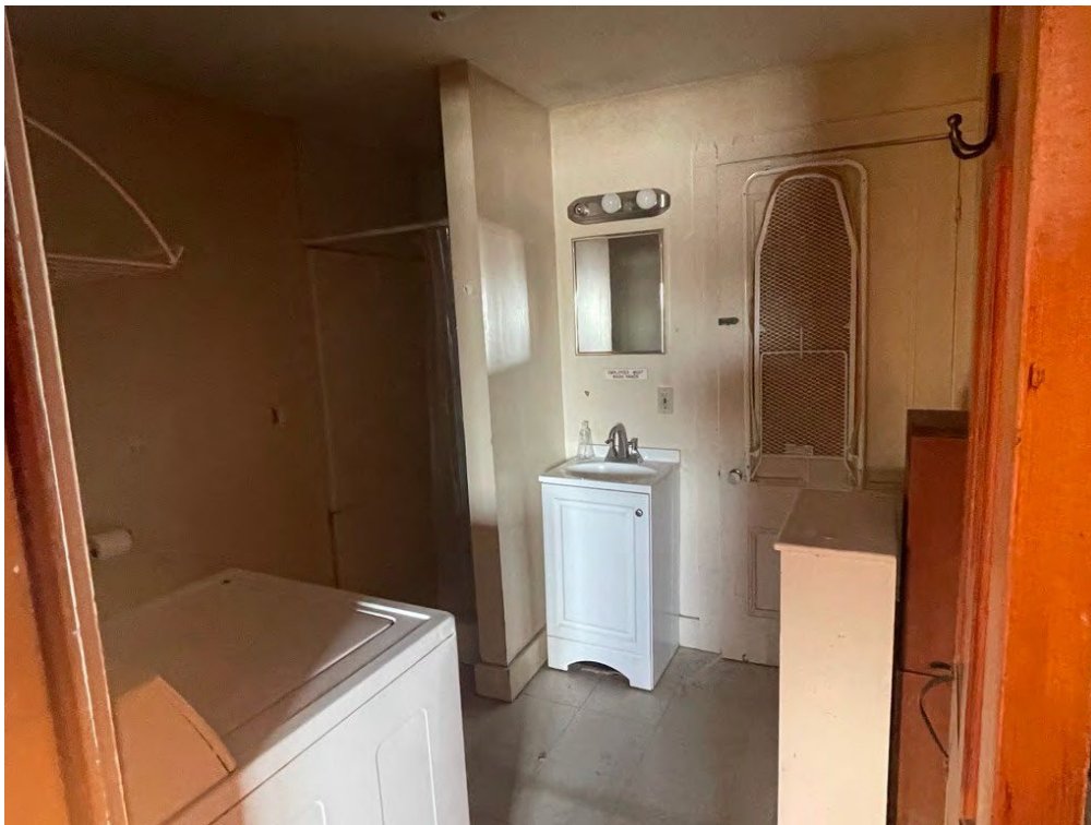
Image 24: View of the first-floor bathroom looking east.
