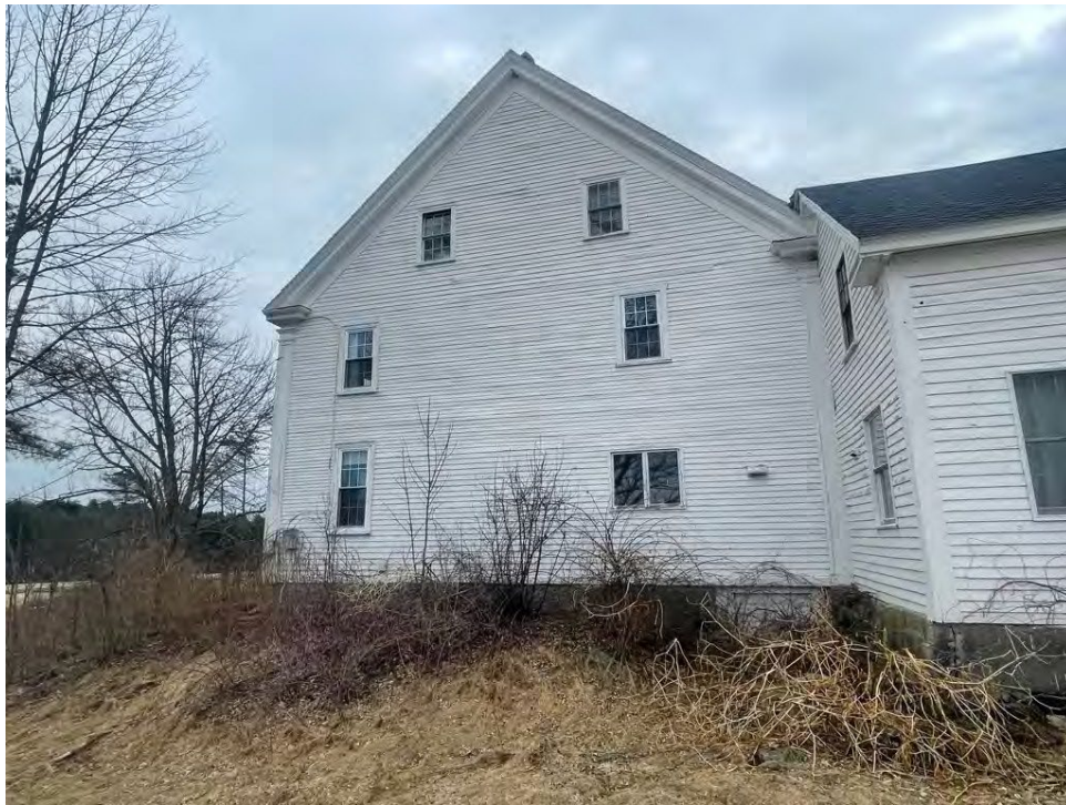
Image 52: View of the west elevation looking east, showing overgrowth.
