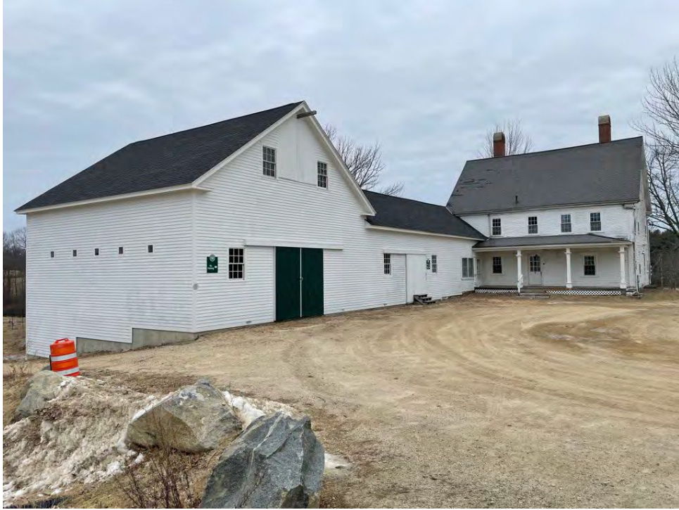
Image 7: South elevation of the building complex looking north.
