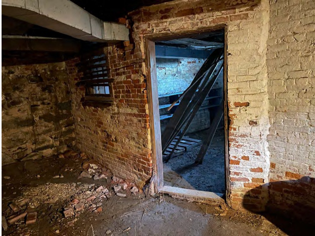
Image 13: View of added brick partition leading to the dairy, looking northeast.
