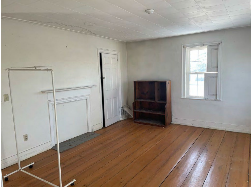
Image 27: View of the northwest chamber looking southwest.
