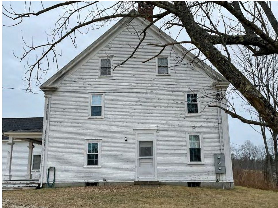
Image 6: View of east elevation looking west.
