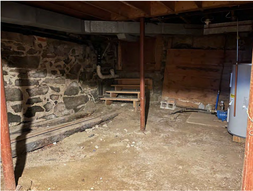
Image 11: View of basement looking southwest, showing rubble granite.
