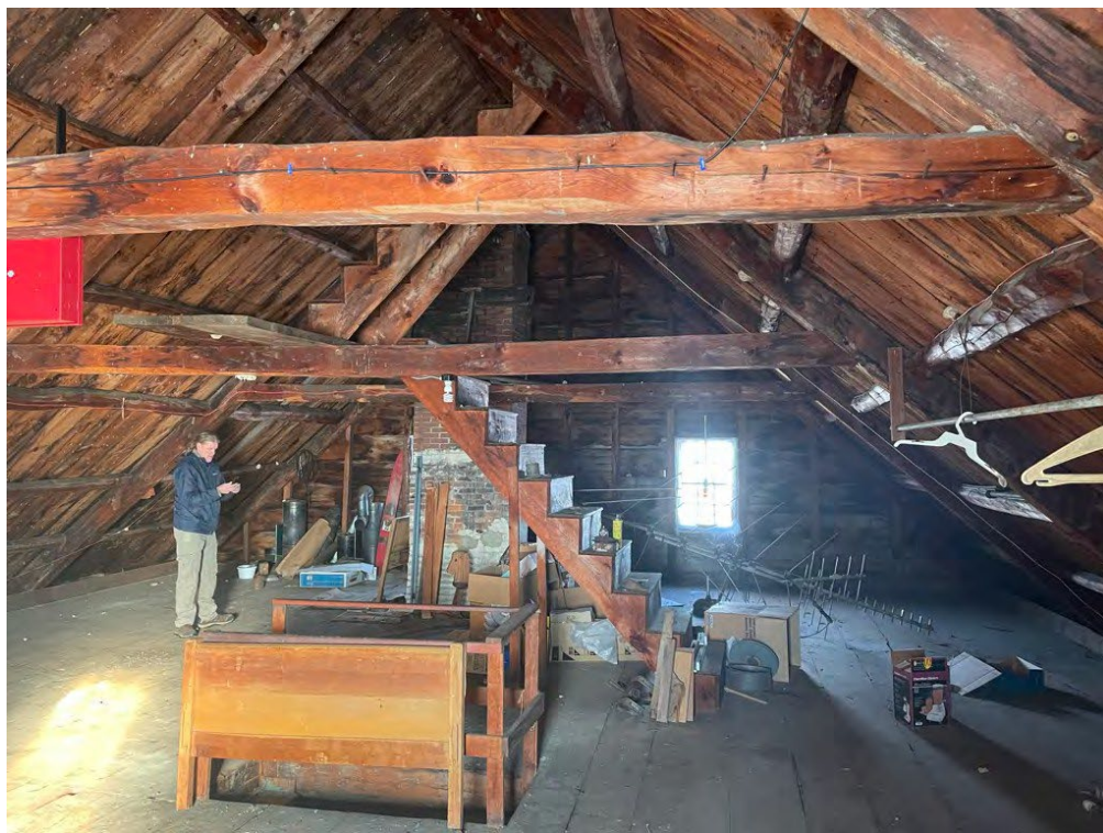
Image 14: View of the attic looking east.
