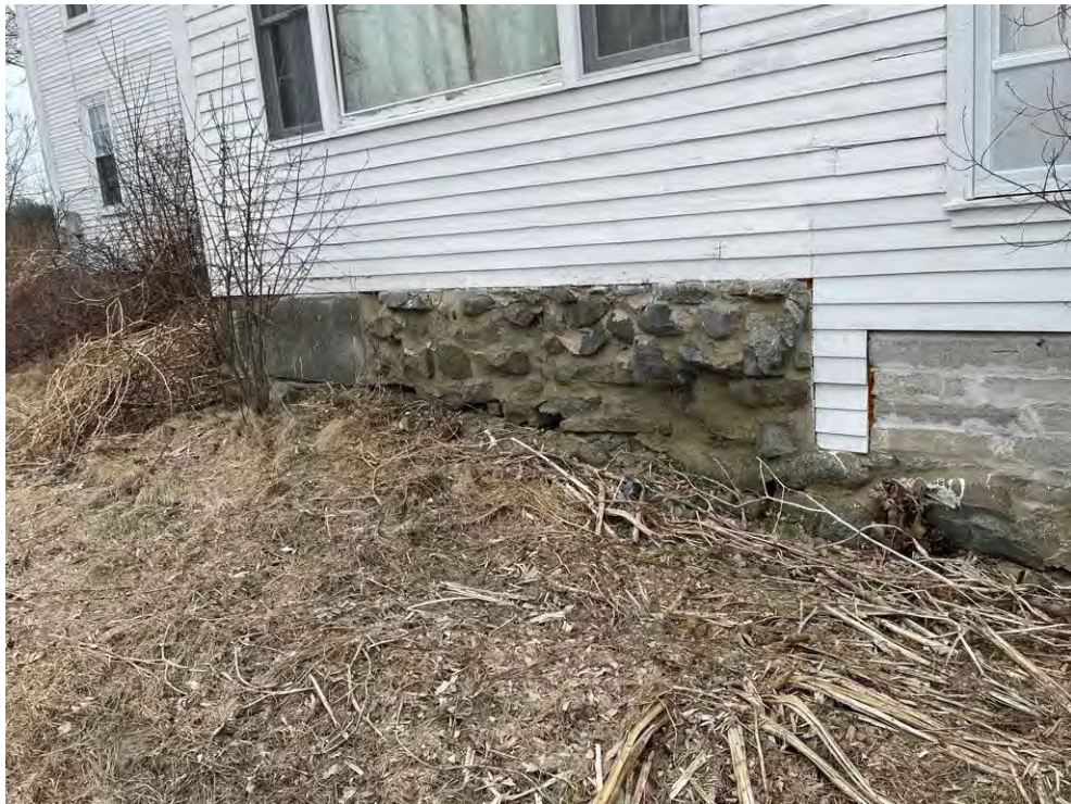
Image 48: View of the west elevation of the ell's foundation, showing variable materials and conditions.
