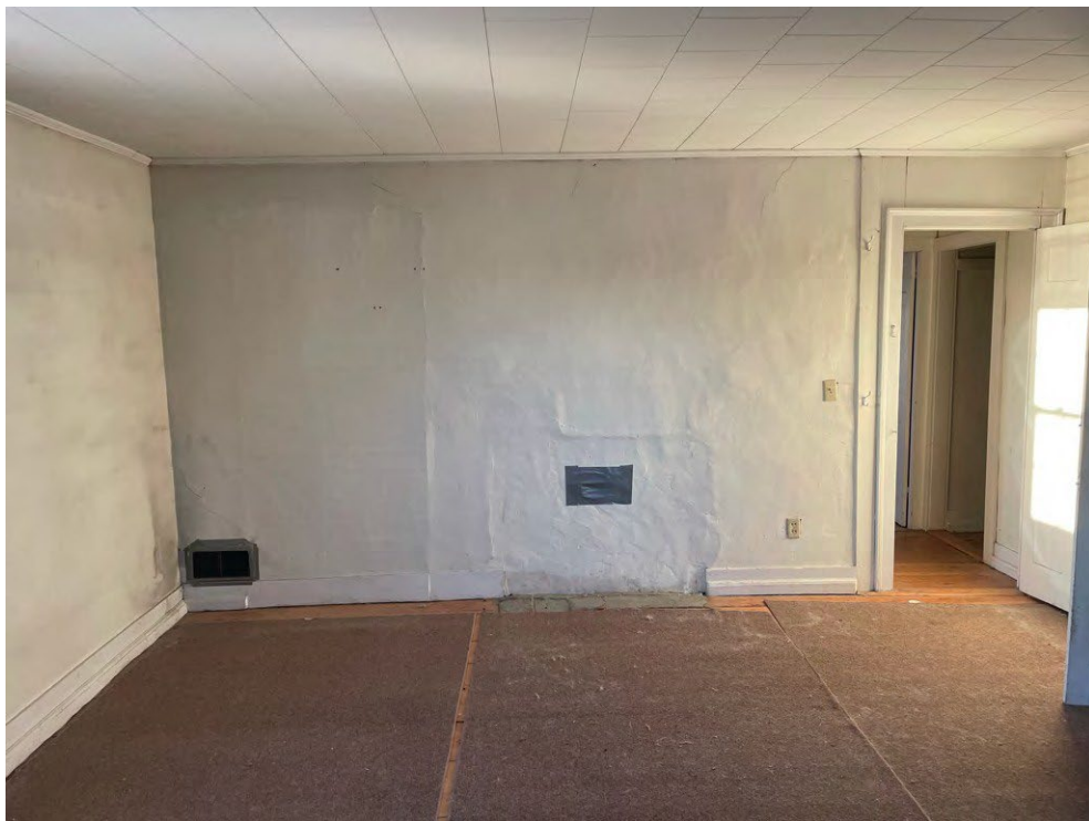
Image 30: View of southwest chamber looking north.
