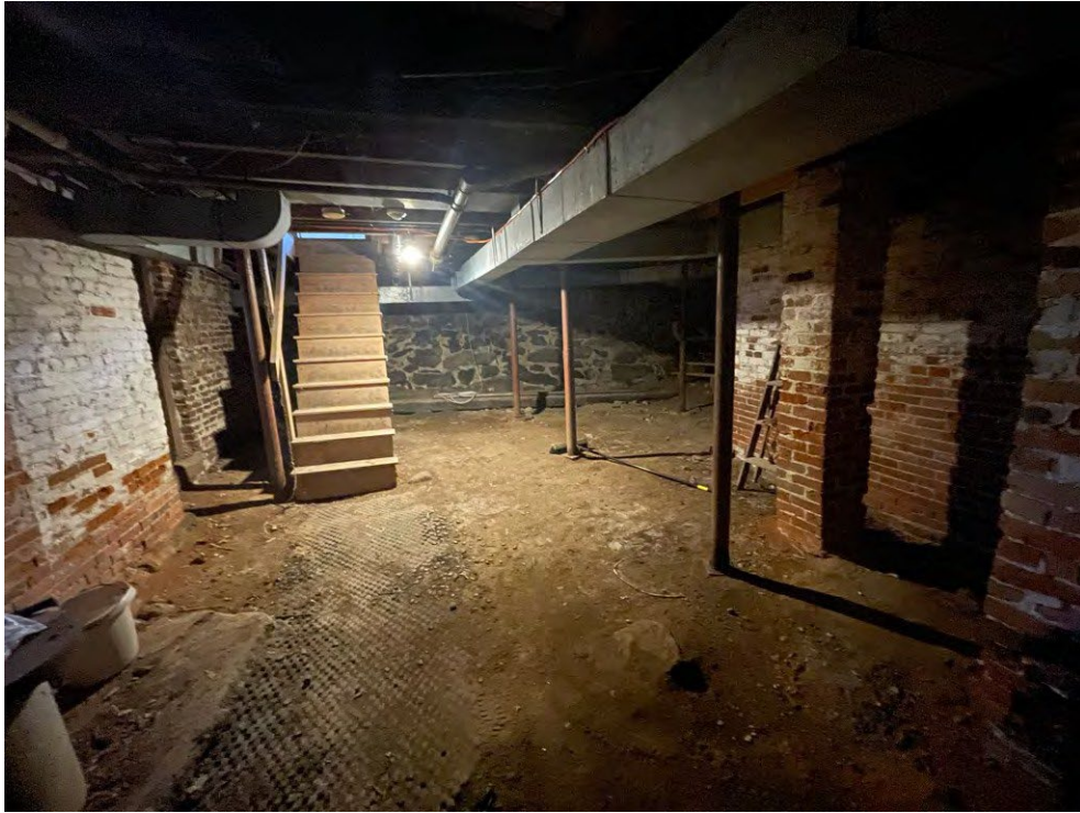
Image 9: View of basement looking south.
