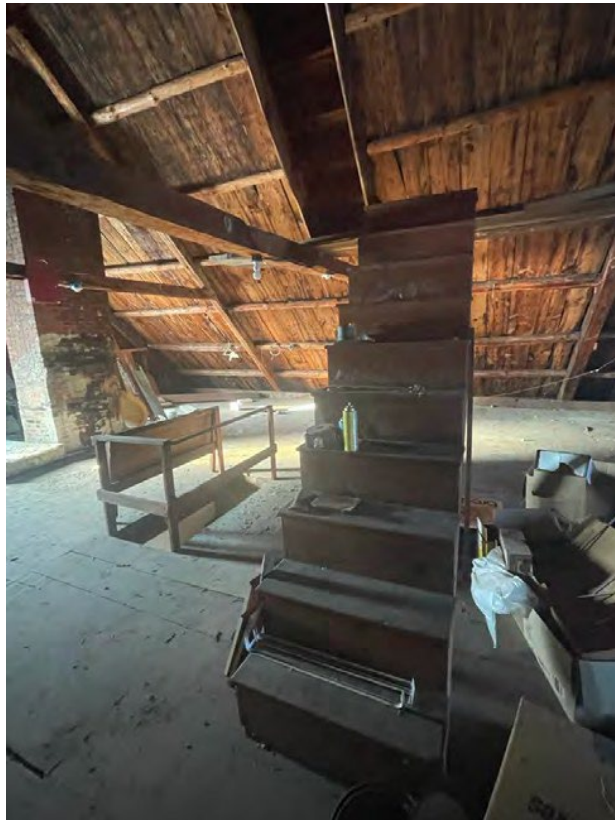
Image 15: View of the stairs leading to the attic scuttle looking north.
