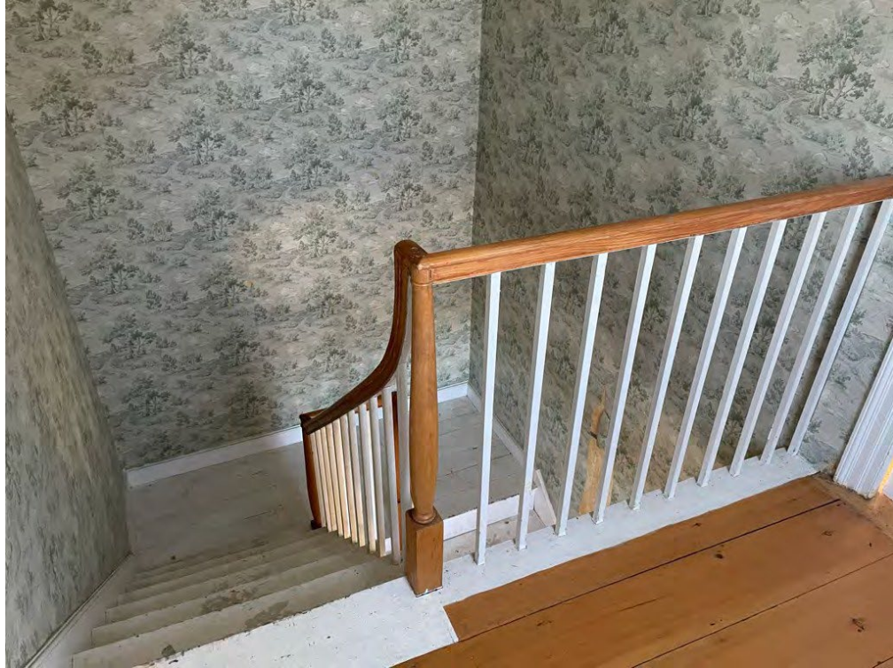
Image 25: View of the center hall stairs, second floor, looking down and south.
