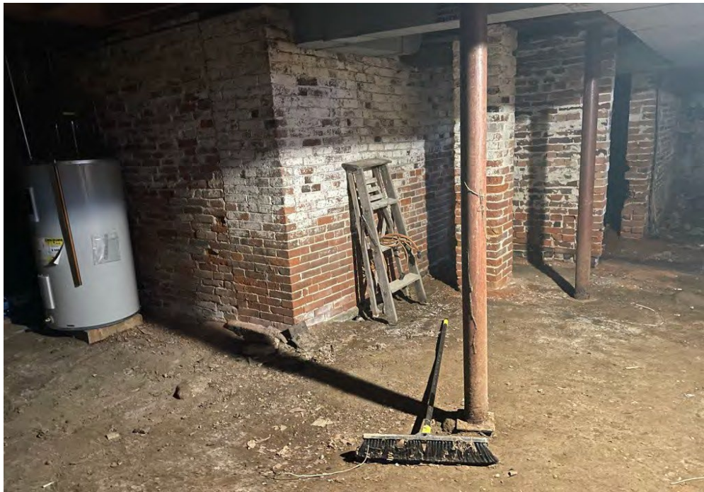
Image 10: View of basement looking northwest showing the west chimney base, added brick room partition and steel lolly columns.
