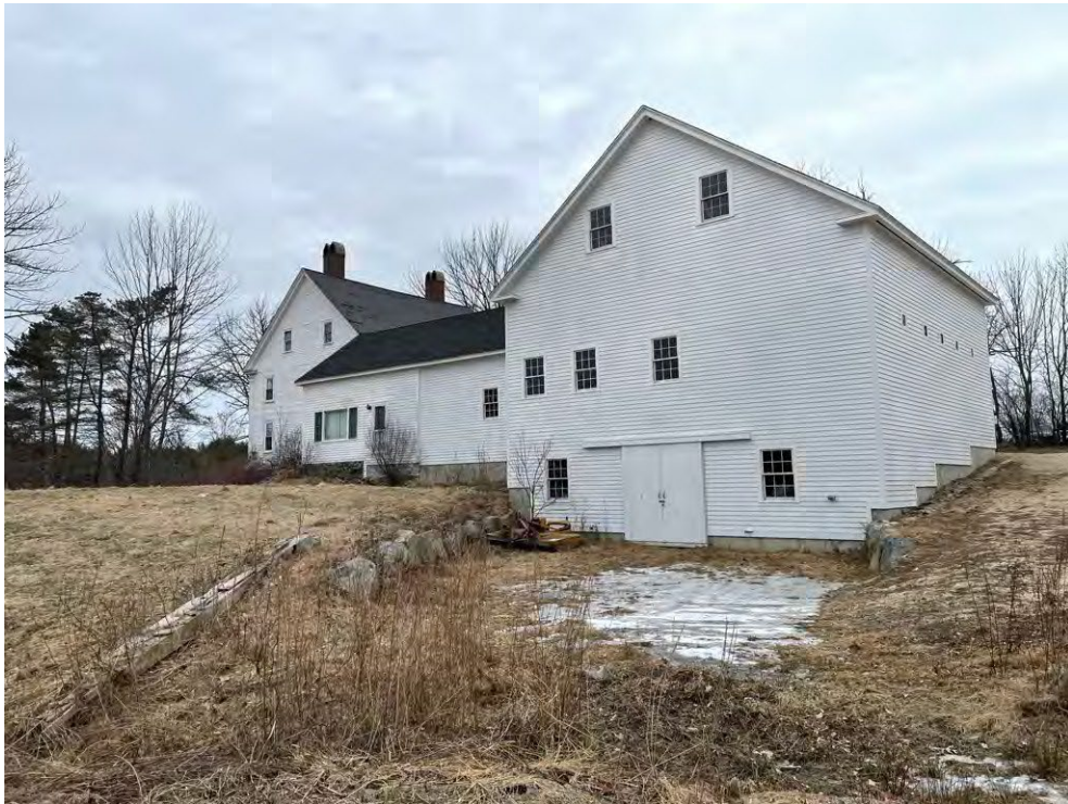
Image 8: View of the building complex looking northeast
