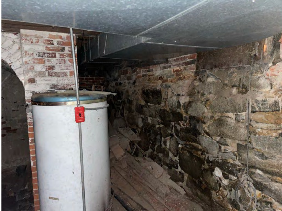
Image 47: View of the north foundation wall, west end, looking west.
