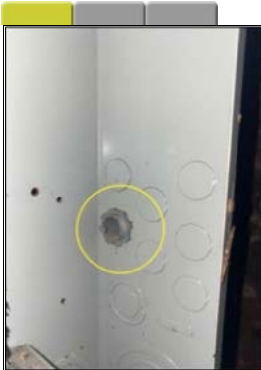
Small opening in large panel
