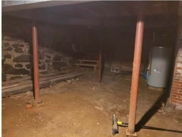
Photo 9 Previously re-framed section at southwest corner of main house
