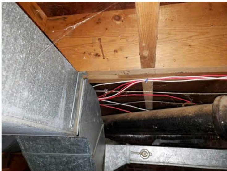
Photo 16 Reframed area at southwest corner of main house lacking hangers at common joists, beam is improperly spliced
