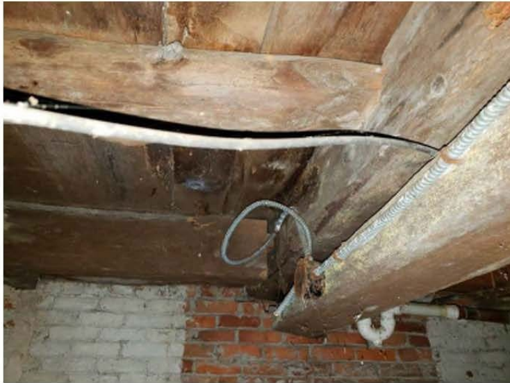
Photo 15 Various flush-framed conditions
