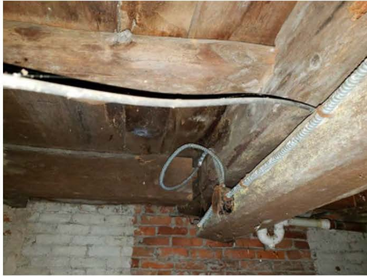
Photo 15 Various flush-framed conditions
