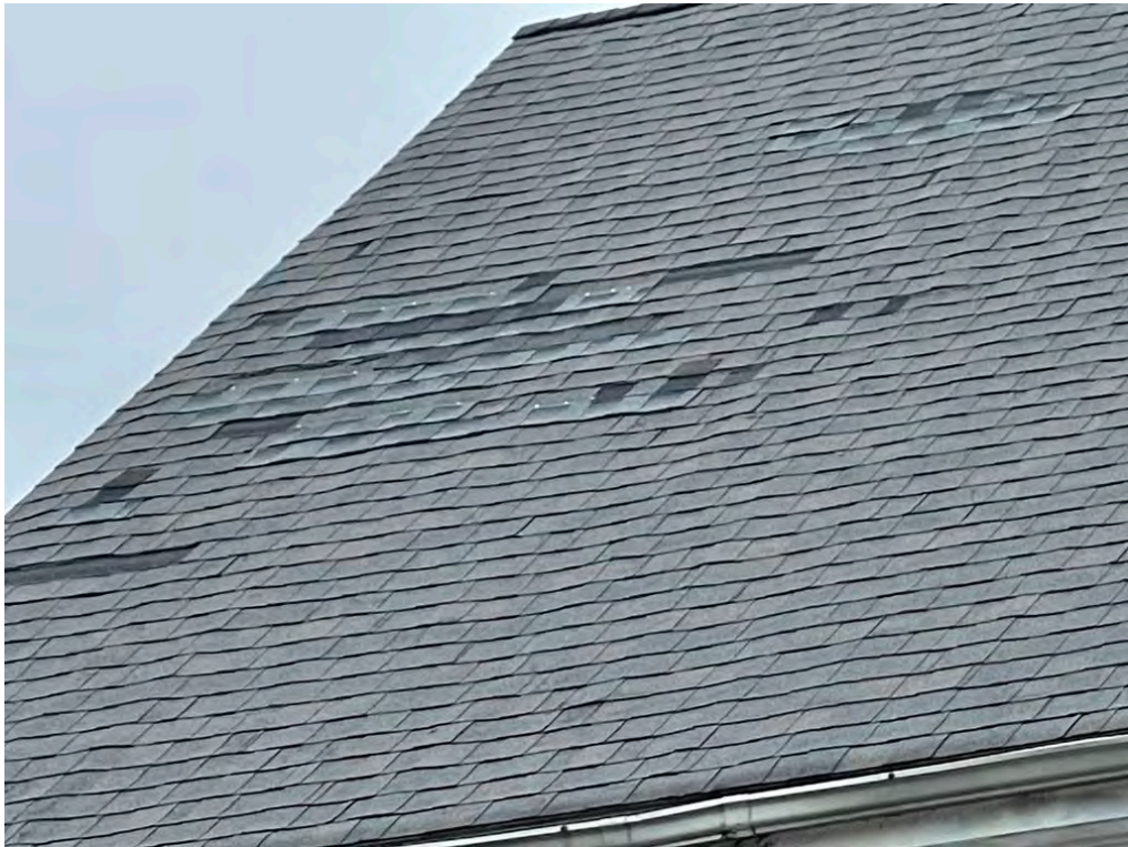
Image 36: Detail of the roof, main house, south elevation, showing shingle repairs.
