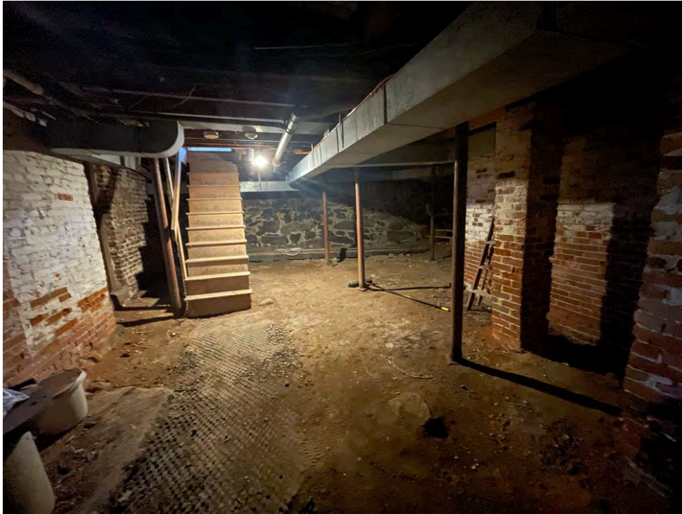
Image 9: View of basement looking south.
