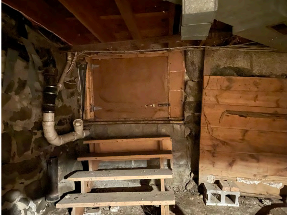
Image 33: View of basement, southwest corner looking west, showing replaced floor framing.
