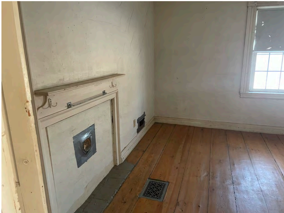
Image 28: View of southeast middle chamber looking east.
