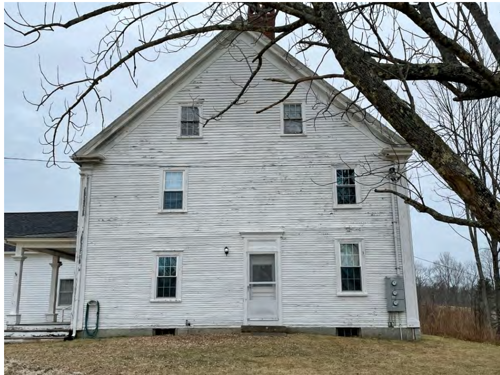
Image 6: View of east elevation looking west.
