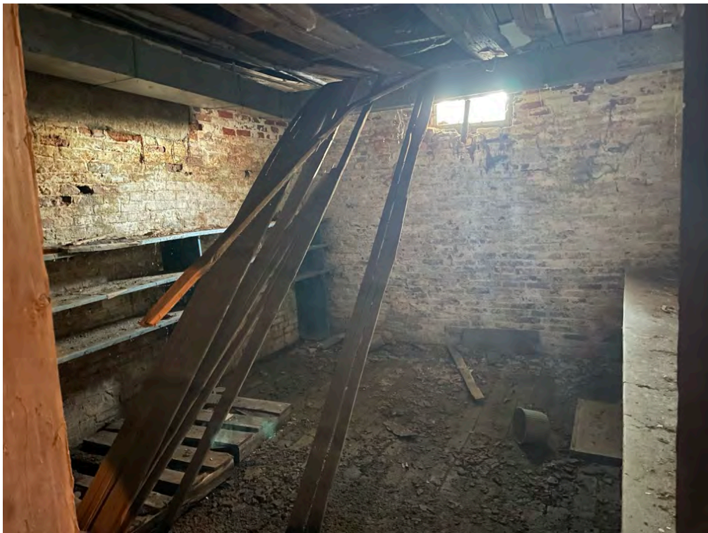
Image 12: View of basement dairy room looking northeast.
