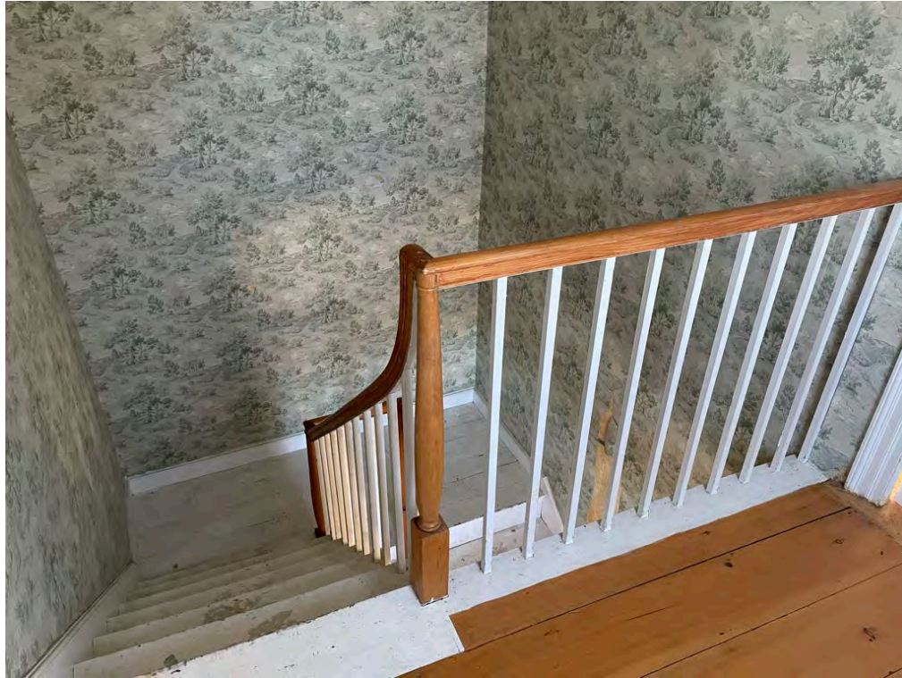
Image 25: View of the center hall stairs, second floor, looking down and south.
