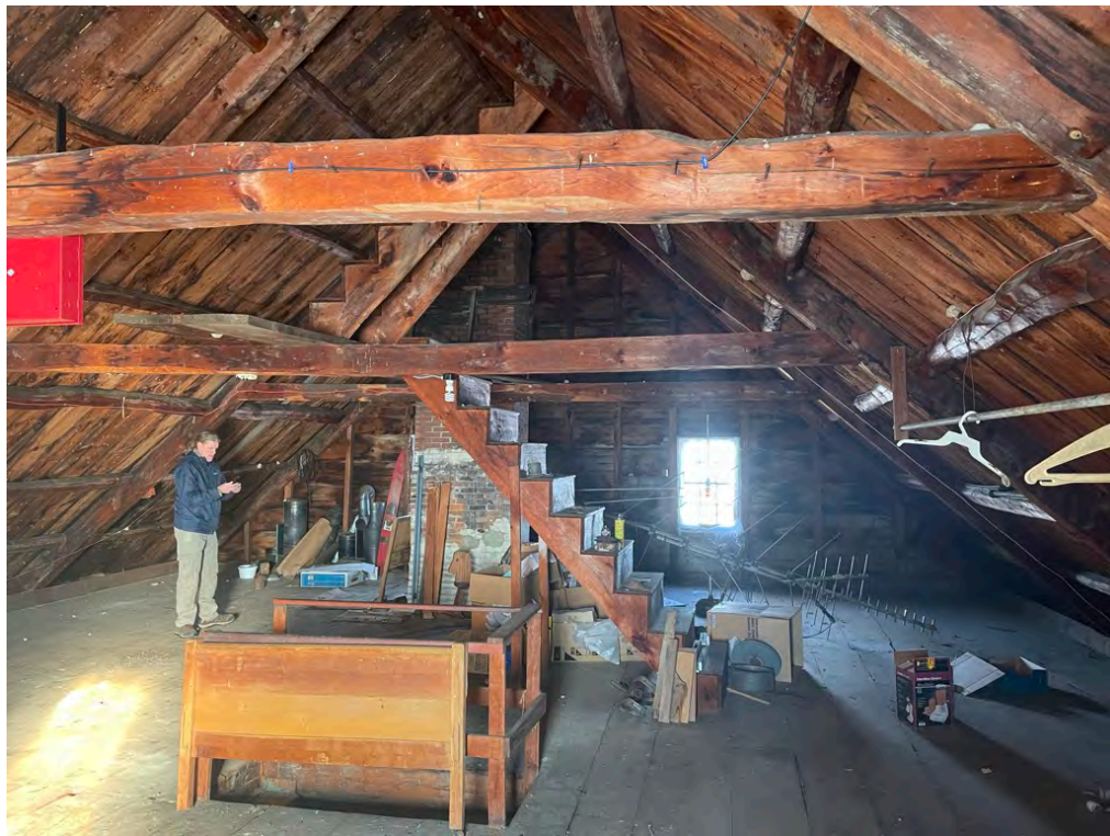
Image 14: View of the attic looking east.
