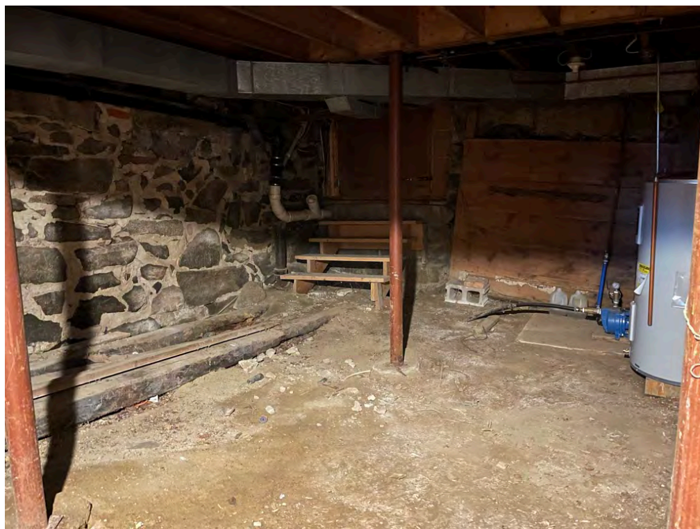
Image 46: View of the south basement wall, west end, looking west.
