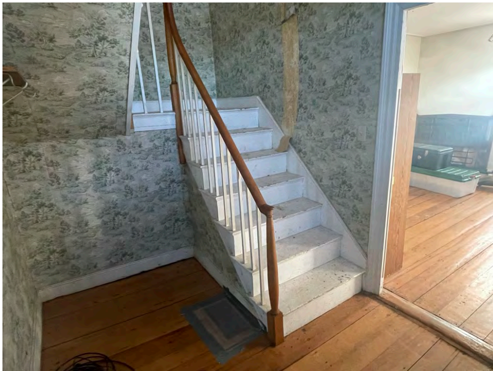
Image 18: View of the front stair hall looking southwest.
