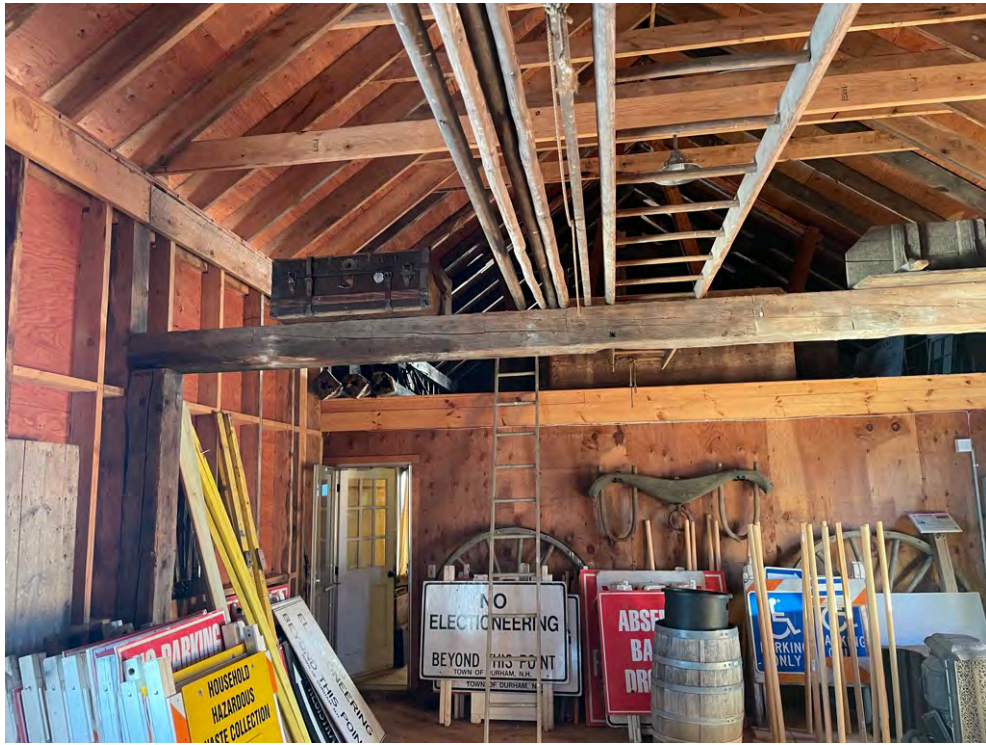
Image 17: View of the roof framing of the original portion of the ell looking north from the modern portion of the ell.
