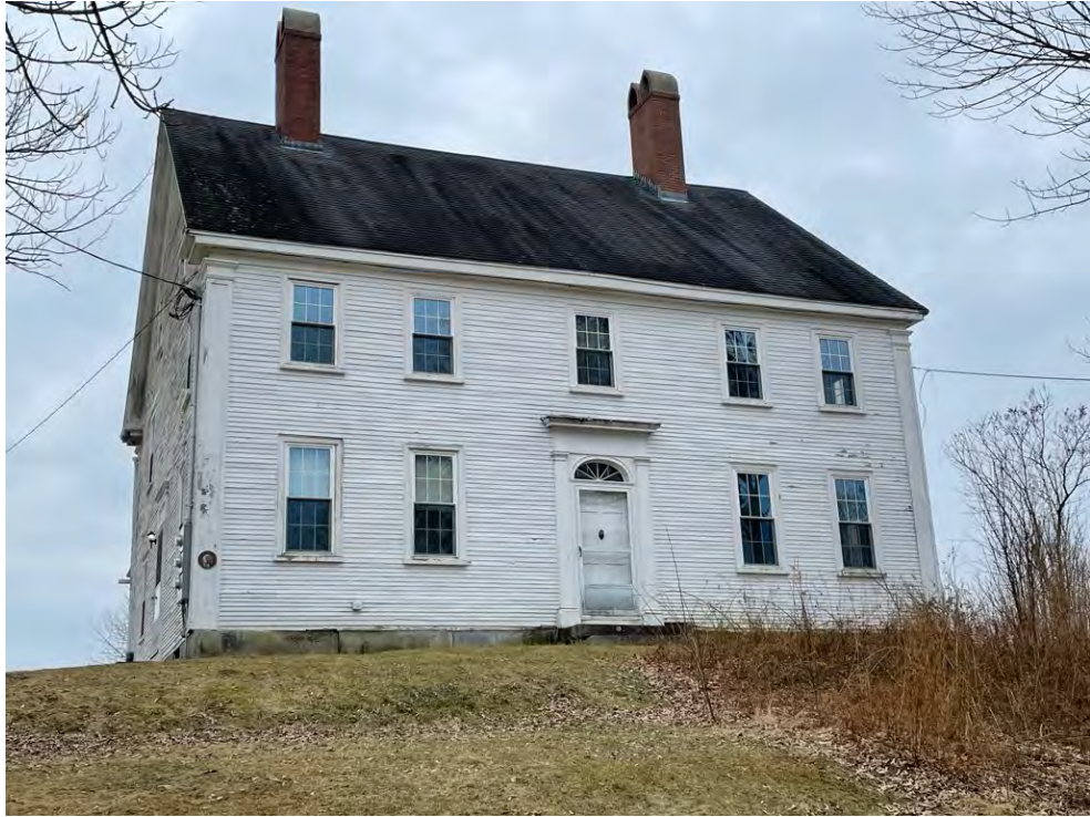
Image 5: Front elevation of the main house looking south.
