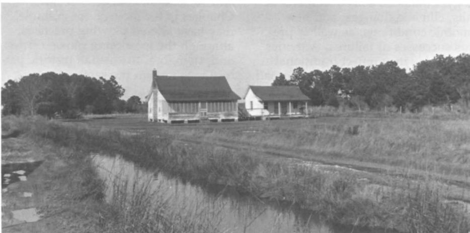
Drainage ditches and canals divide the agricultural fields and flat plains of Lake Landing in Hyde County, North Carolina. Implemented in the 19th century, this system made possible water transportation and the farming of swampy lowlands. Coastal plain cottages represent the common housing stock of the region. (J. Timothy Keller)
