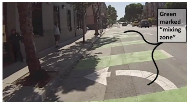
Mixing Zone with Green Coloring Photo from survey (shown): Fell St. and Broderick St. Video Location(s): Fell St. and Baker St.
