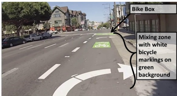
Mixing Zone with Sharrow Photo from survey (shown): Oak St. and Broderick St. Video Location(s): Oak St. and Broderick St
