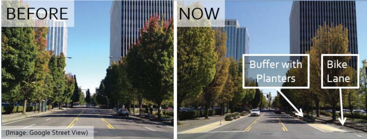
Figure 3-26. NE Multnomah St., Portland, OR, Before and After Installation of Protected Bike Lane
