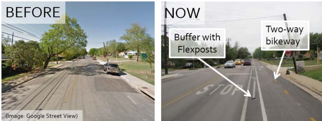
Figure 3-10. Bluebonnet Lane, Austin, TX, Before and After Installation of Protected Bike Lane
