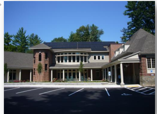
Photo 6: Solar Photovoltaic installation at the Public Library
