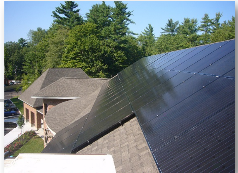
Photo 4: Solar photovoltaic (PV) installation on the Durham Public Library
