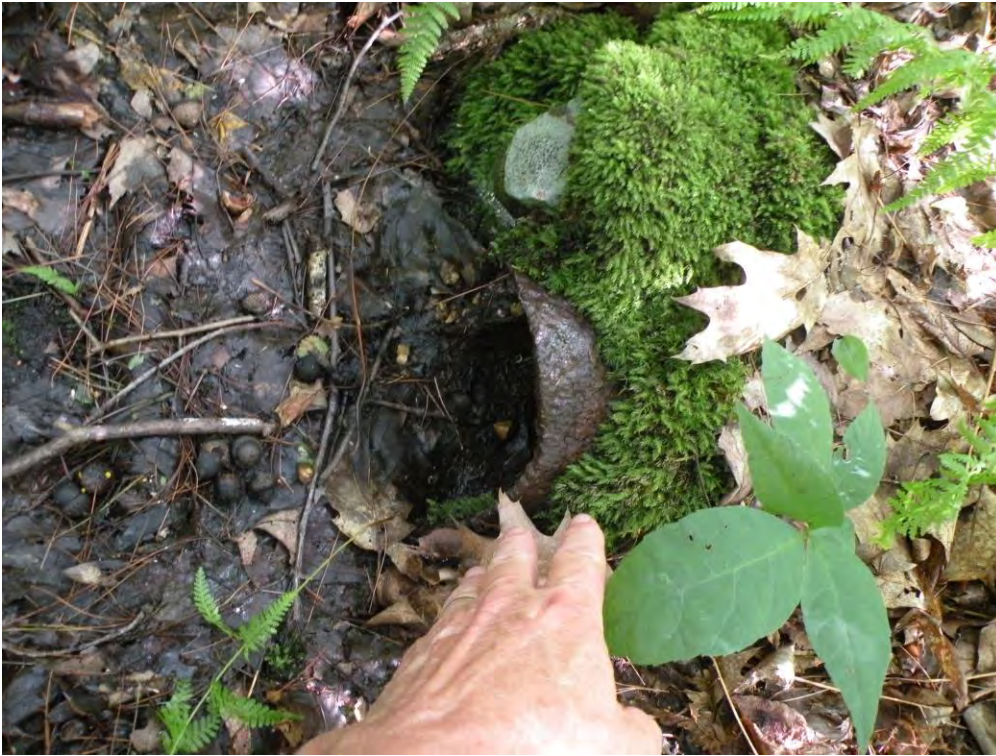
25. This is an iron culver connecting Wetland 8b and 8a.
