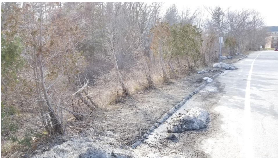
Picture E - Current snow management, pushing snow over the bank down into the riparian corridor. Notice the trees are bent and dying, from this practice.
