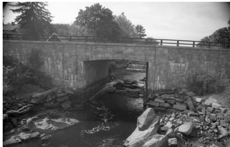
fig. 9 neg0003 looking SW from under rt 108 bridge. falls visible beneath bridge
