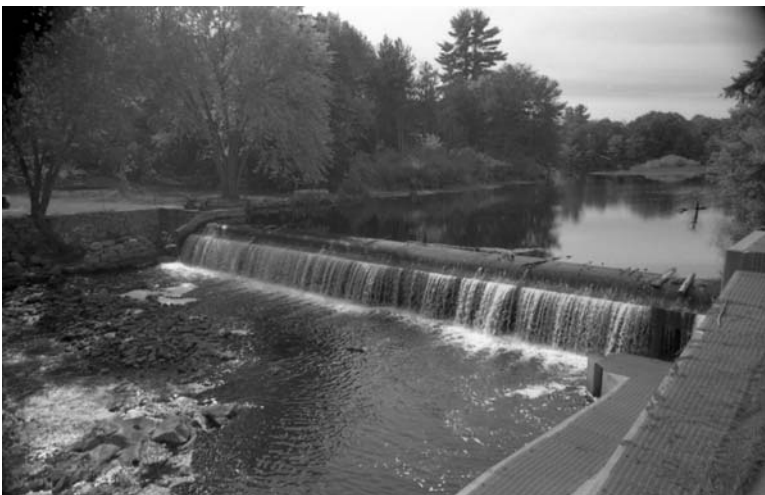
fig. 6 neg0007 looking SW. fish ladder right foreground
