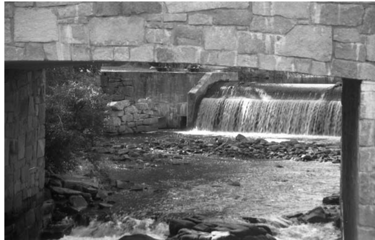
fig.10 neg0006 view from under rt 108 bridge looking SW
