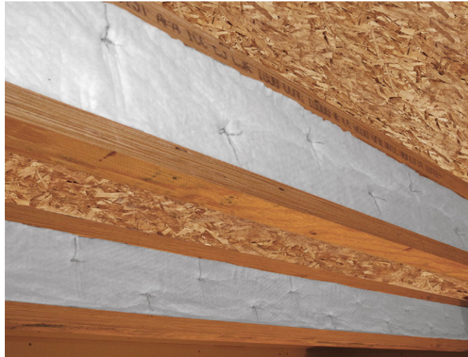
A proprietary ceramic fiber blanket insulation can be attached to the web of the I-joists to comply with IRC provisions. Photo courtesy of Mei Guo International, LLC (USA) FireBreak™.
