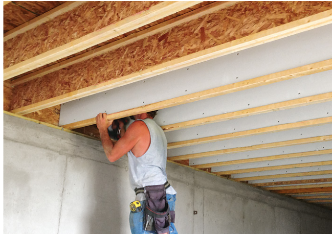
Installing 1/2-inch gypsum board to I-joist webs is one of several methods builders and installing dealers can use to meet the IRC provisions.
