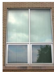
There is no lintel, or special treatment, over this window, so it appears that the brick above would simply collapse. (95)
