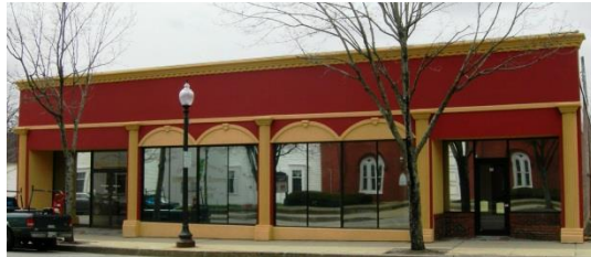
Rochester – new façade (59)
