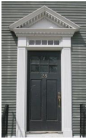
Door surround Ballard House (100)
